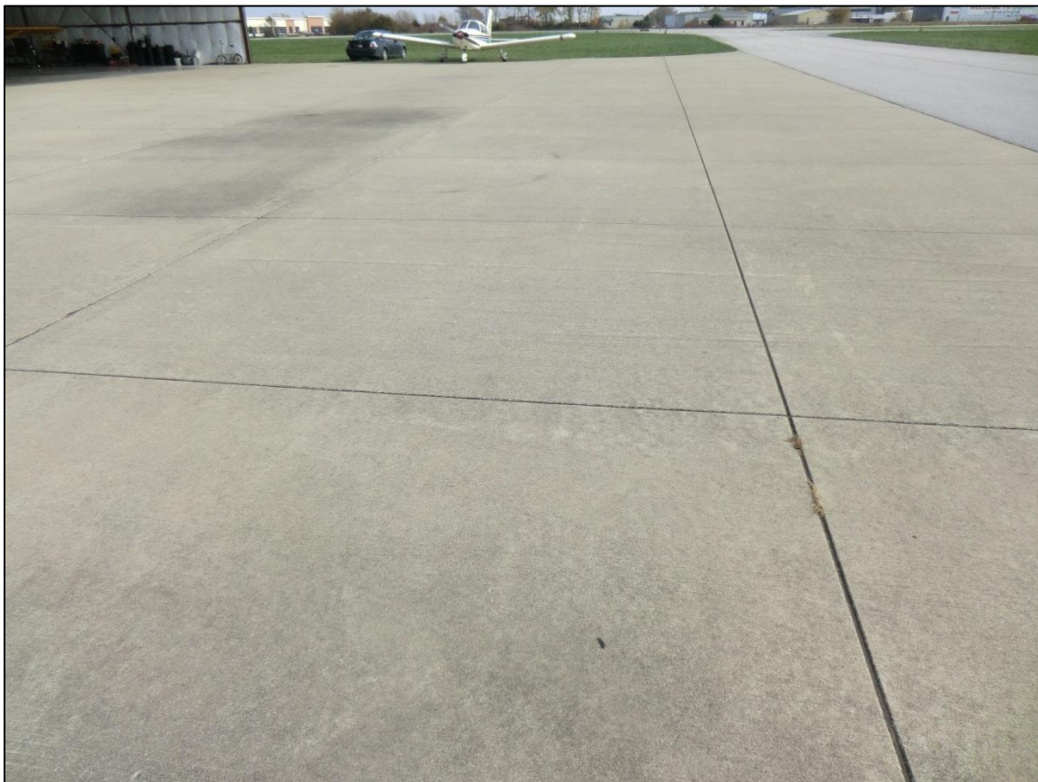
Figure 2-3. Typical Good PCC Pavement (Feature 3105)
