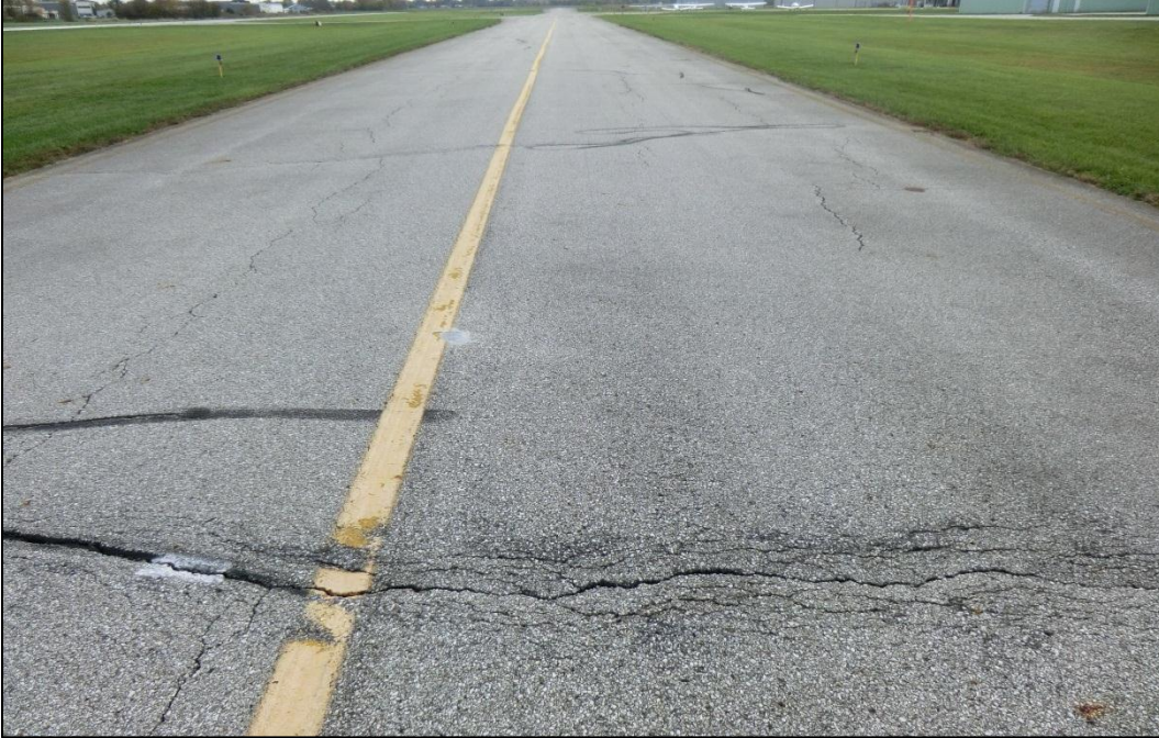
Figure 2-6. Typical Poor AC Pavement (Feature 110)
