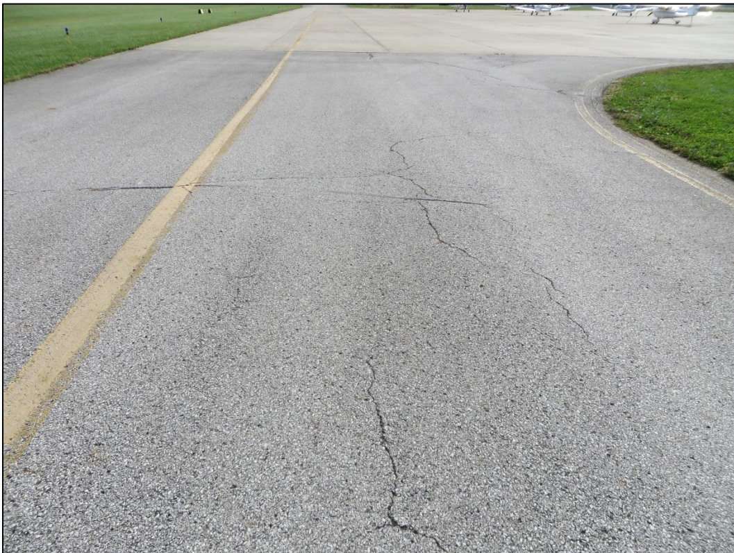
Figure 2-5. Typical Fair AC Pavement (Feature 115)
