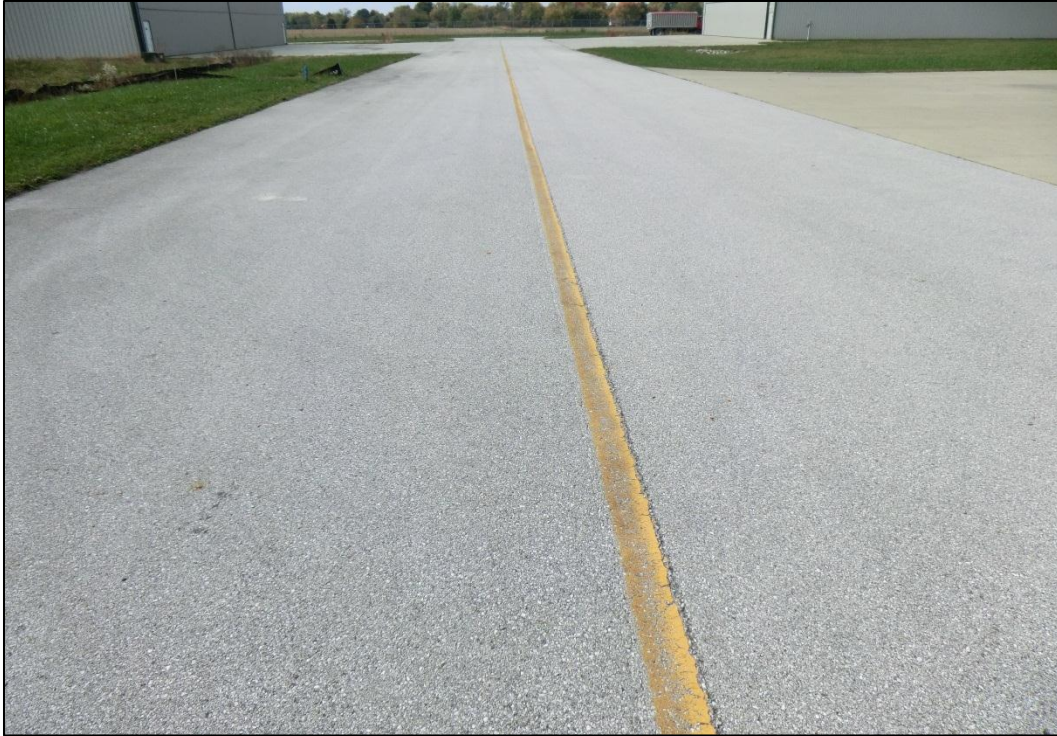
Figure 2-4. Typical Good AC Pavement (Feature 155)
