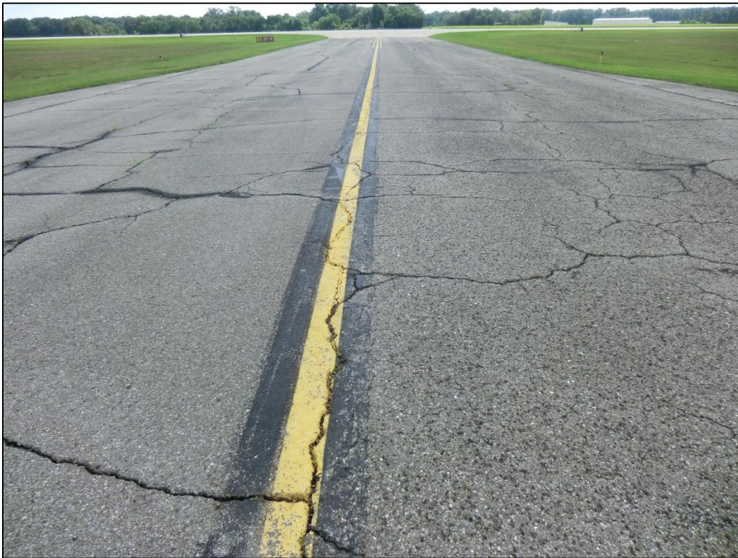
Figure 2-7. Typical Serious AC Pavement (Feature 240)
