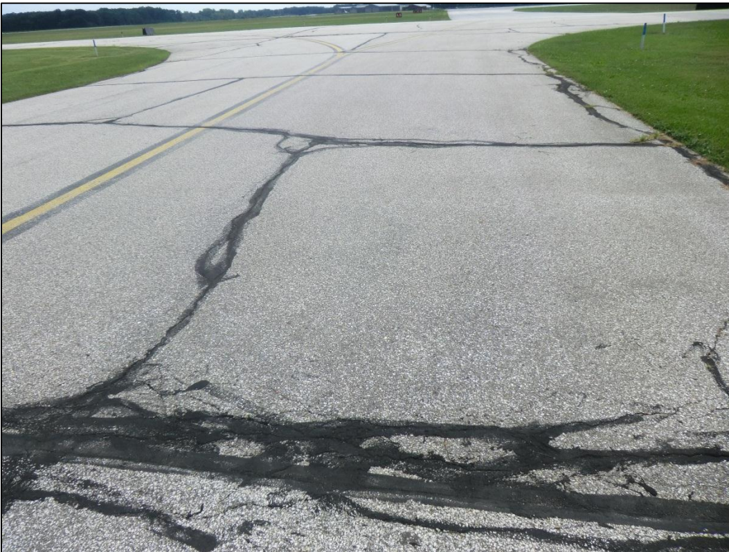
Figure 2-5. Typical Fair AC Pavement (Feature 515)
