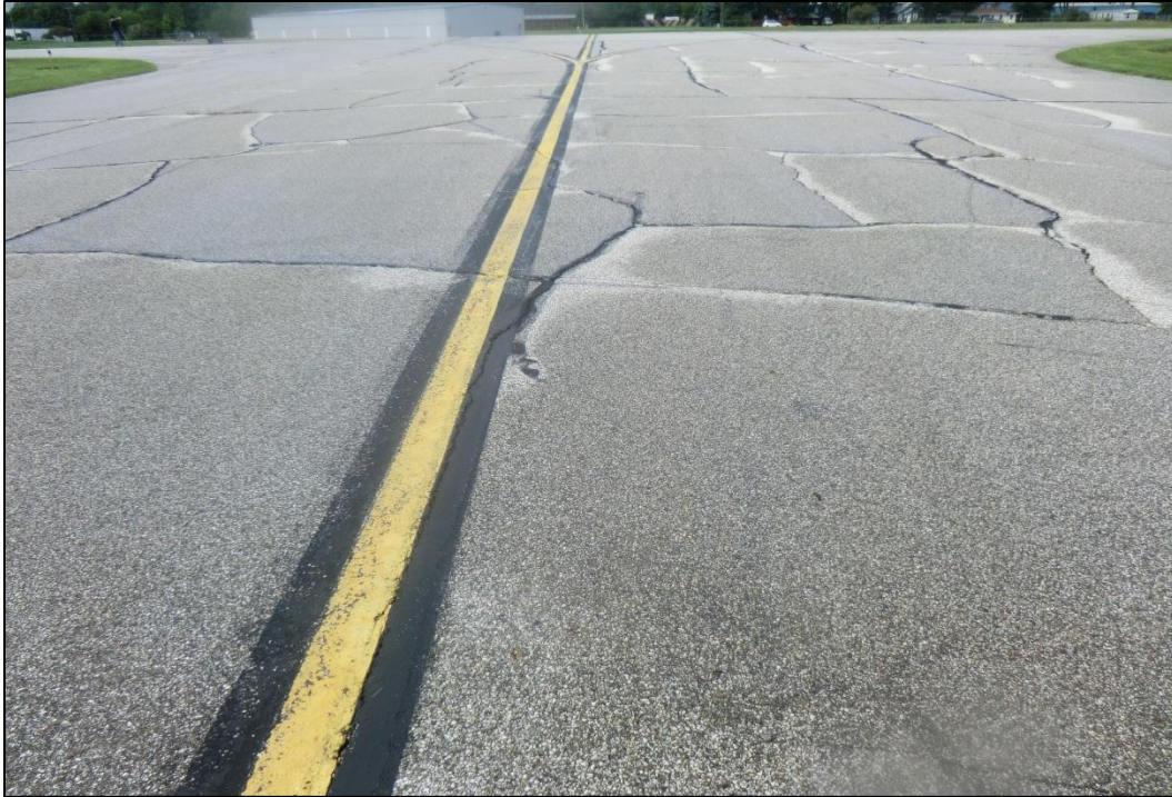
Figure 2-6. Typical Poor AC Pavement (Feature 265)
