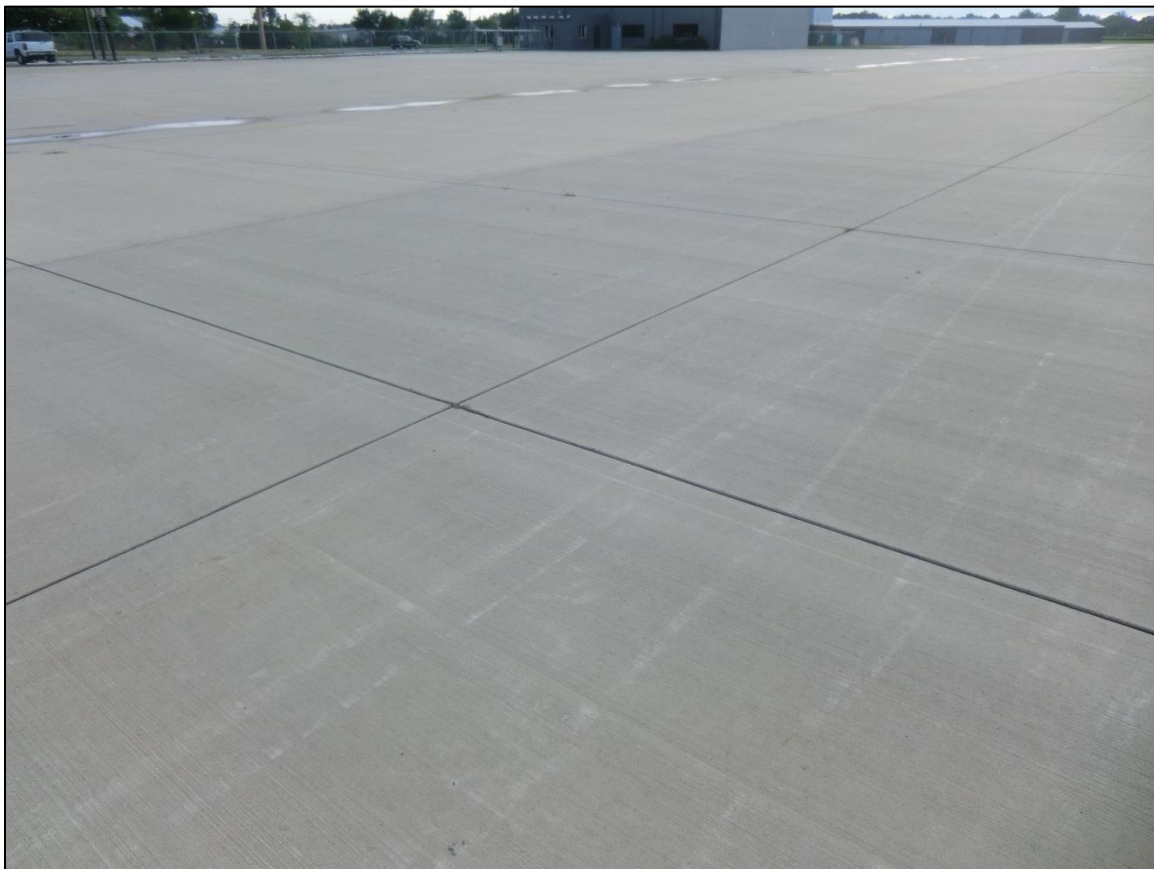
Figure 2-3. Typical Good PCC Pavement (Feature 3105)
