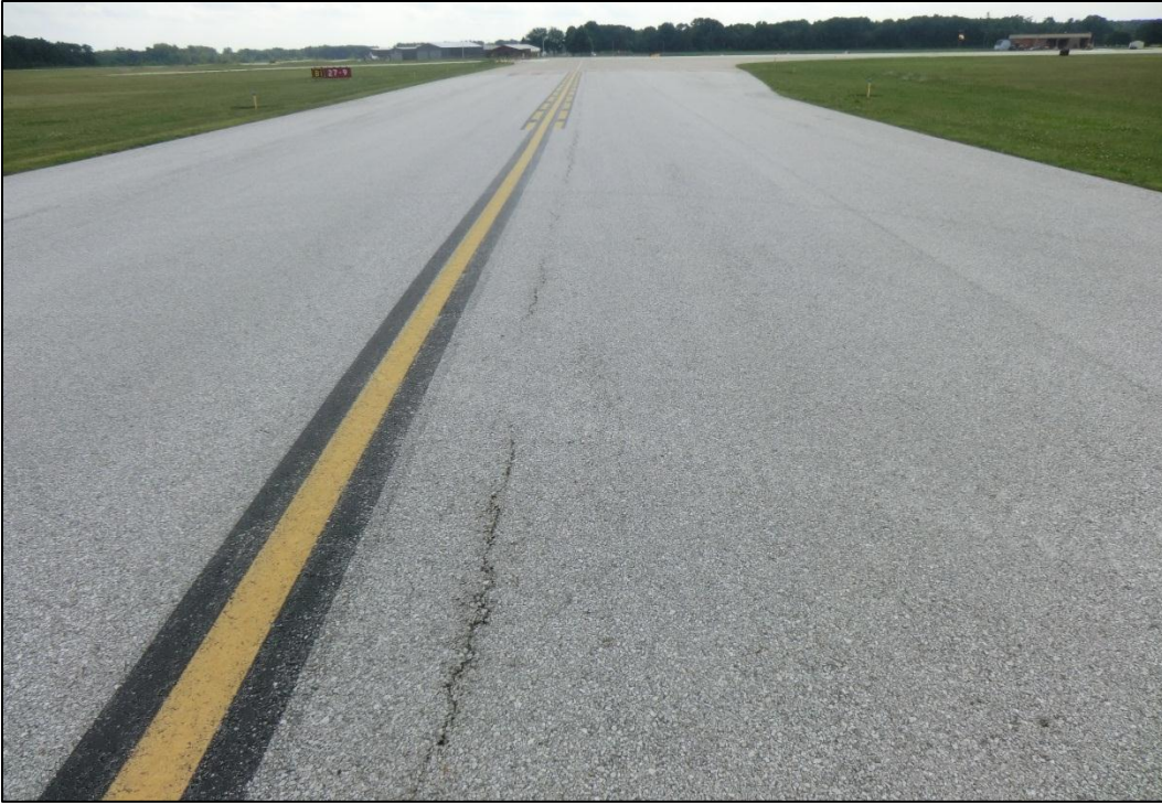
Figure 2-4. Typical Good AC Pavement (Feature 230)
