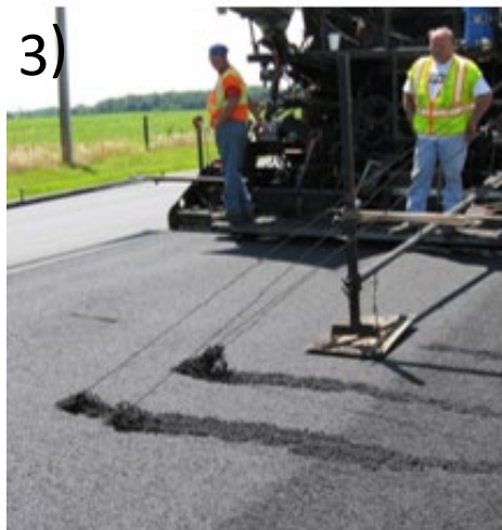
Figure 7-6 Plate Sampling: 1) Setting plates; 2) Final plate arrangement; 3) Locating plates after paving; 4) Collecting loose HMA material for testing
