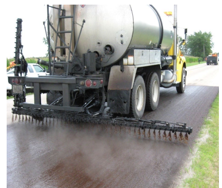
Figure 4-7 Tack Coat Application
