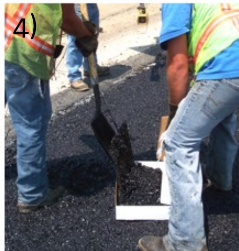
Figure 7-6 Plate Sampling: 1) Setting plates; 2) Final plate arrangement; 3) Locating plates after paving; 4) Collecting loose HMA material for testing
