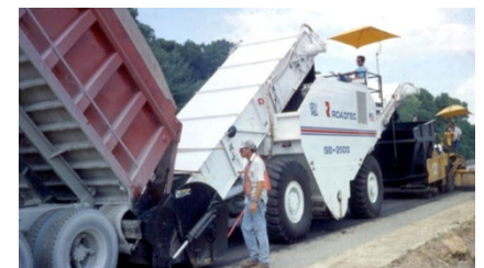
Figure 3-15 Material Transfer Vehicle
