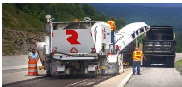
Figure 4-2 Milling Machine
