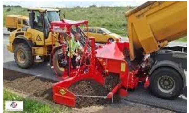
Figure 3-7 Widening Machine
