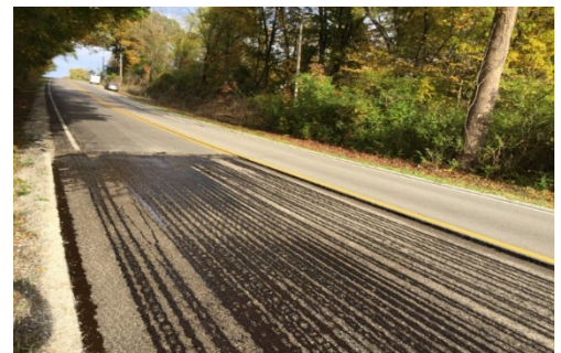
Figure 4-8 Poor Tack Coat Application
