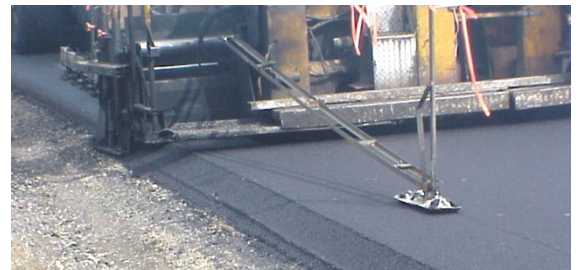
Figure 5-5 Safety Edge
