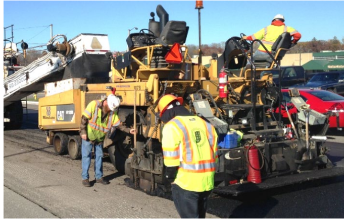
Figure 3-3 HMA Paver
