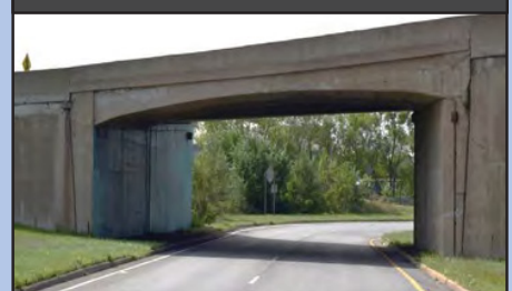
Figure 4: Ramp B over B bridge
