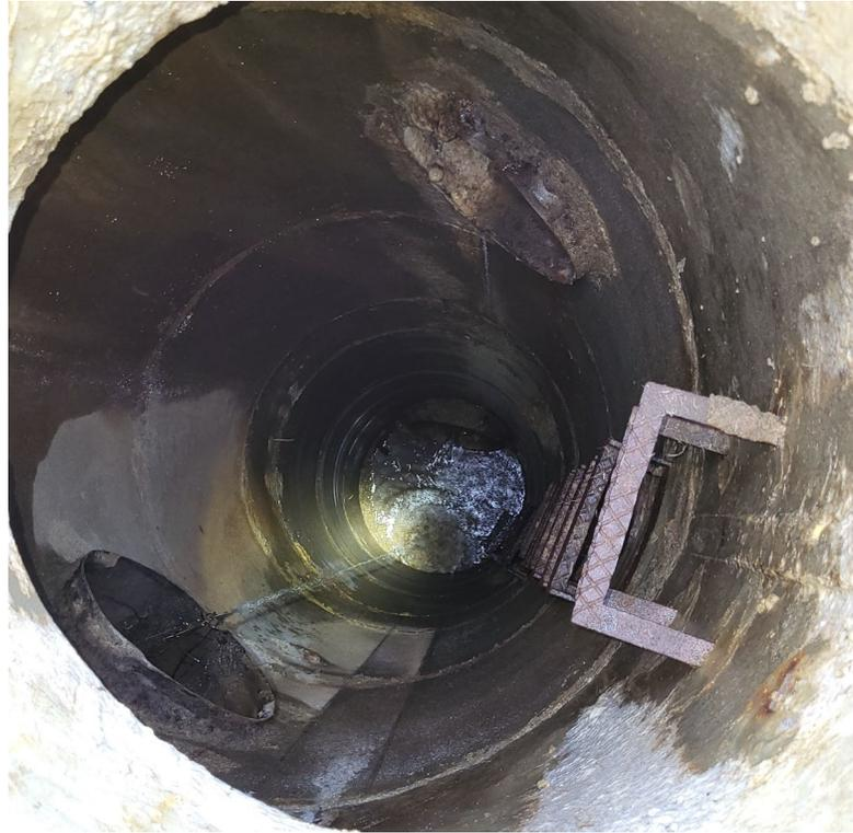
**Special MH Type C-4 – CLV-67047: Interior of MH, approx. 30' deep. Plans specify 8' structure depth with no additional pipe at invert**
