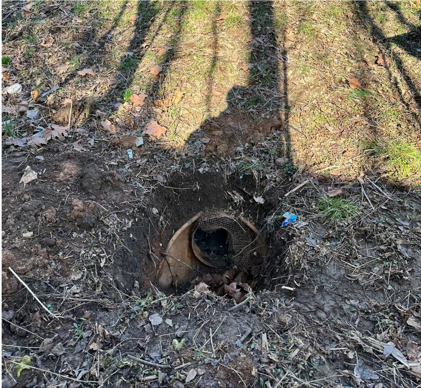
**Chimney Structure – East Inlet of CLV-67029: Note the existing metal mesh and heavy sedimentation of adjacent ditches**
