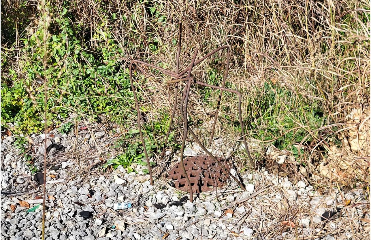
**R.C. sinkhole cap with special pipe Cctch basin Located along the east toe of embankment slope near CLV-67016**
