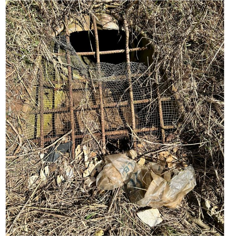
**Special MH Type C-4 – CLV-67047: Inlets of connecting pipes still retain the as designed rebar grating and steel mesh fabric**
