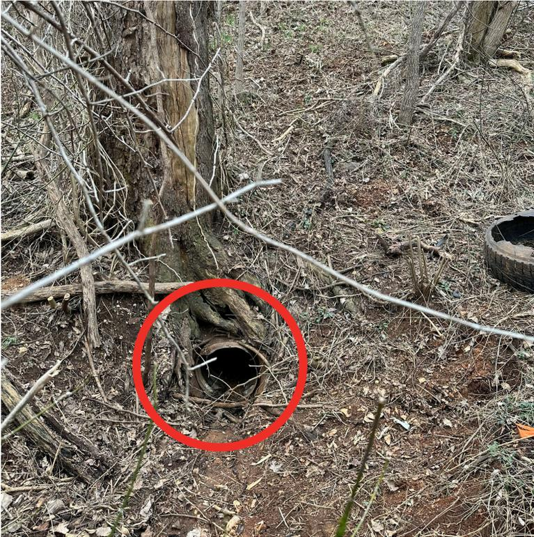
**Chimney Structure – East Inlet of CLV-67023: A number of structures have been encroached upon by trees**
