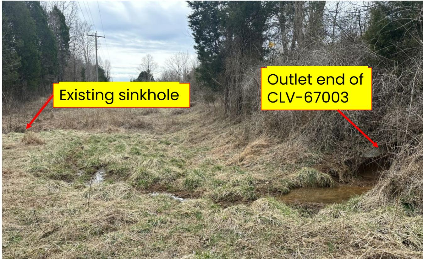
**Existing sinkhole located along the east side of SR 135 that receives CLV-67003 discharge**
