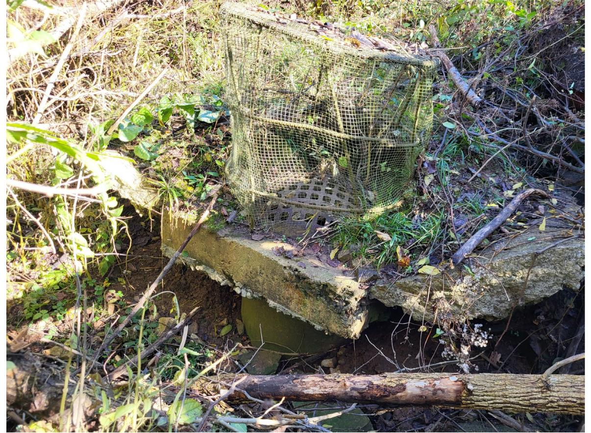
**R.C. sinkhole cap with special pipe catch basin located along the west side of embankment slope near CLV-67610**
