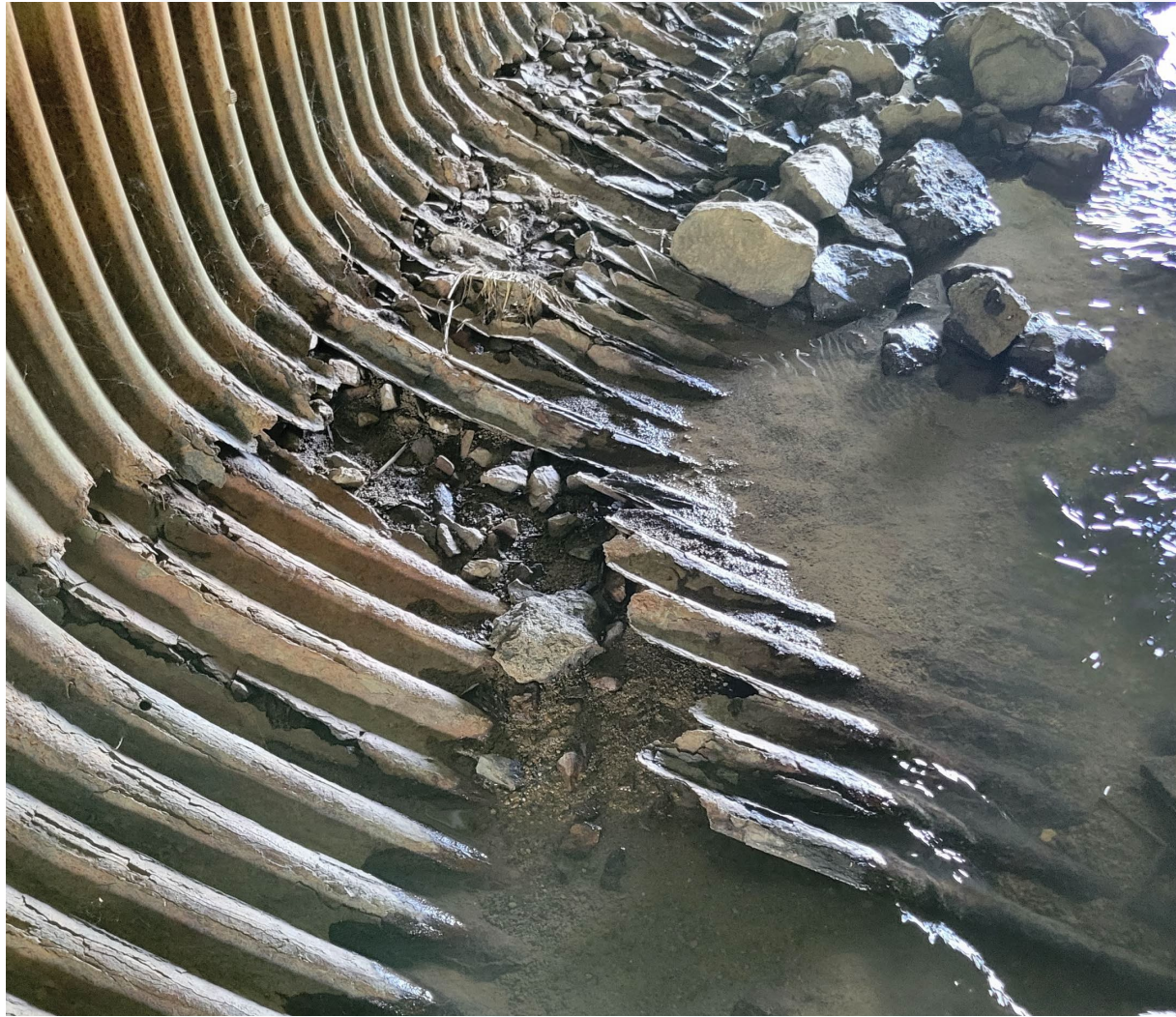
Rust Through at the Waterline
