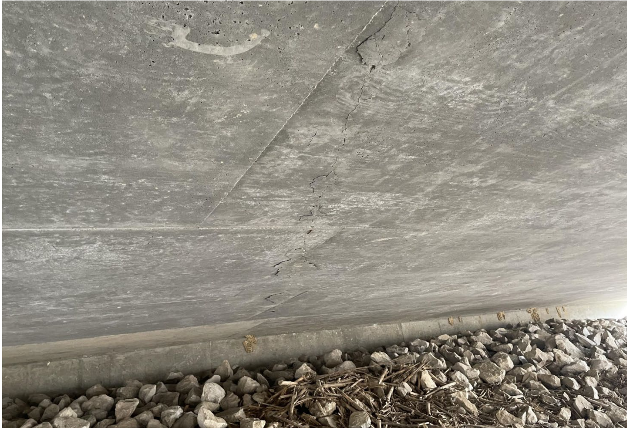
Minor Cracking and Delaminations in the Center of Slab
