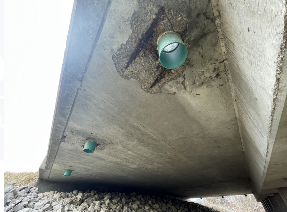
Exposed Steel in Span A, South Coping
