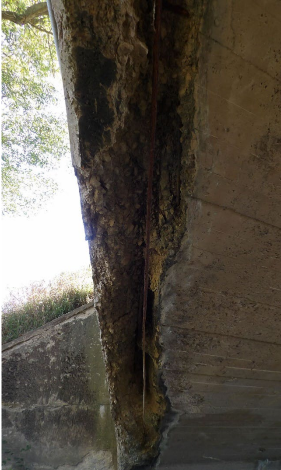
Exposed Steel on NE Coping
