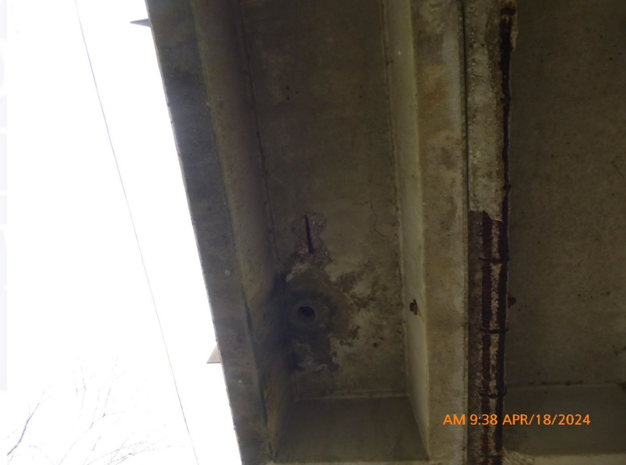
Underside of the Deck with a Minor Spall with Exposed Steel
