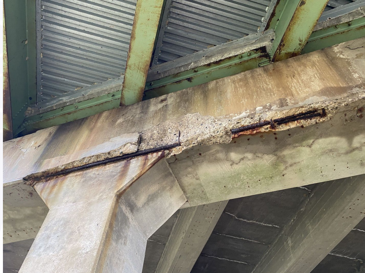
Pier 5 with Exposed Steel
