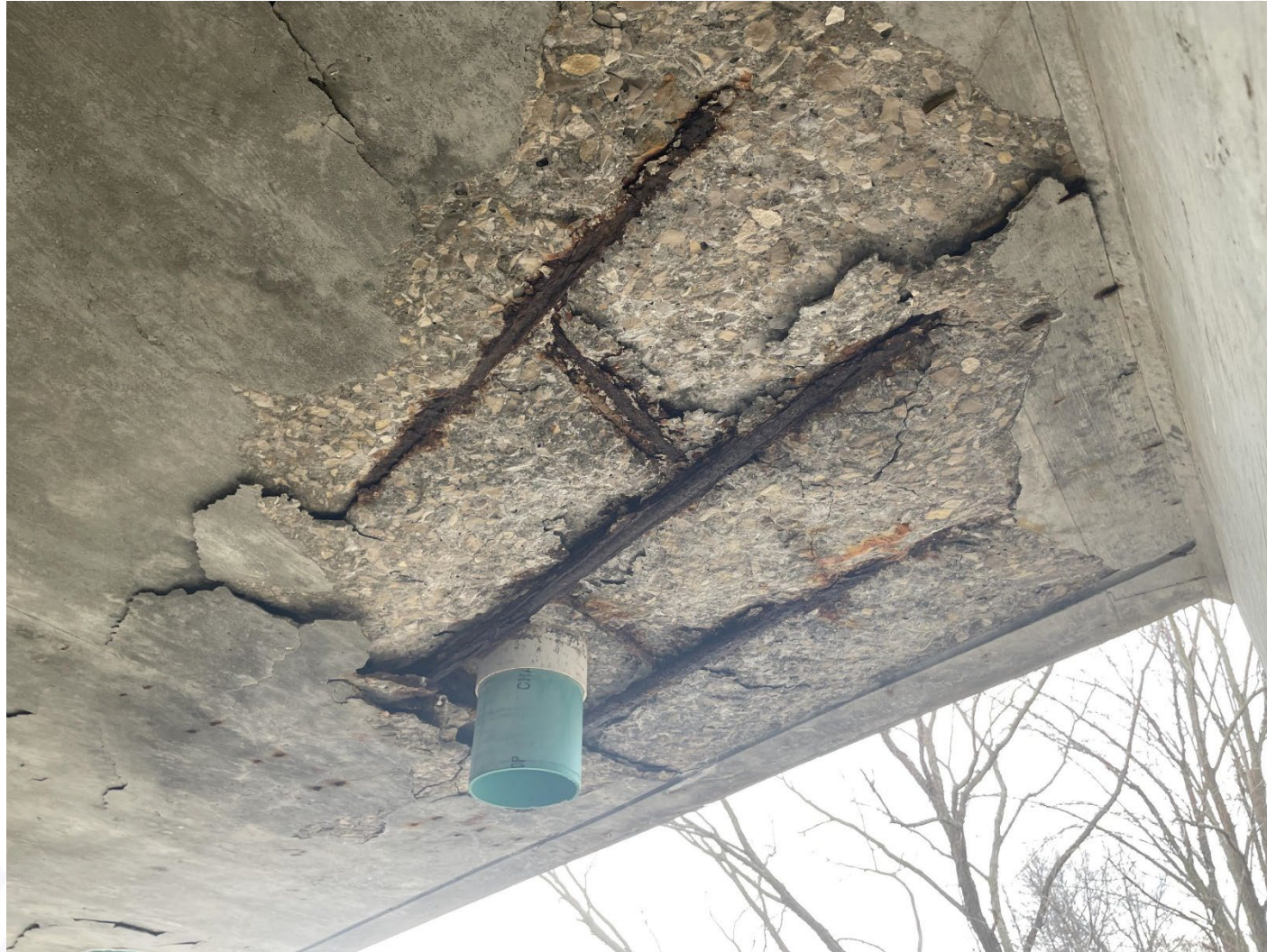
Exposed Steel in Span C, South Coping
