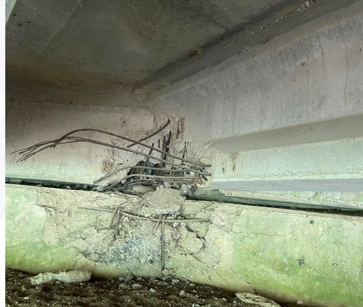
Exposed Strands at Beam 3C (North)
