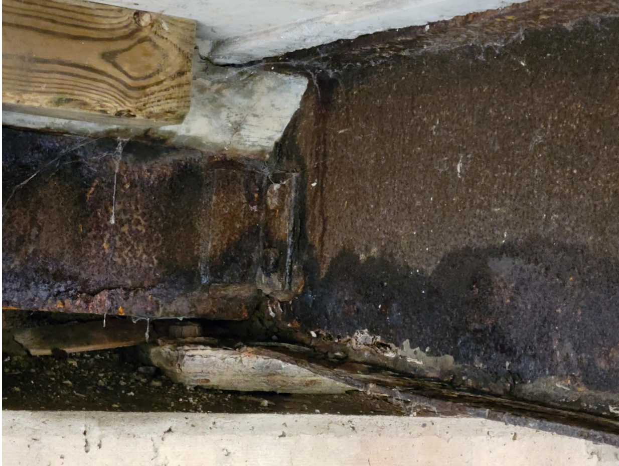
Rust Through of Beam 3C
