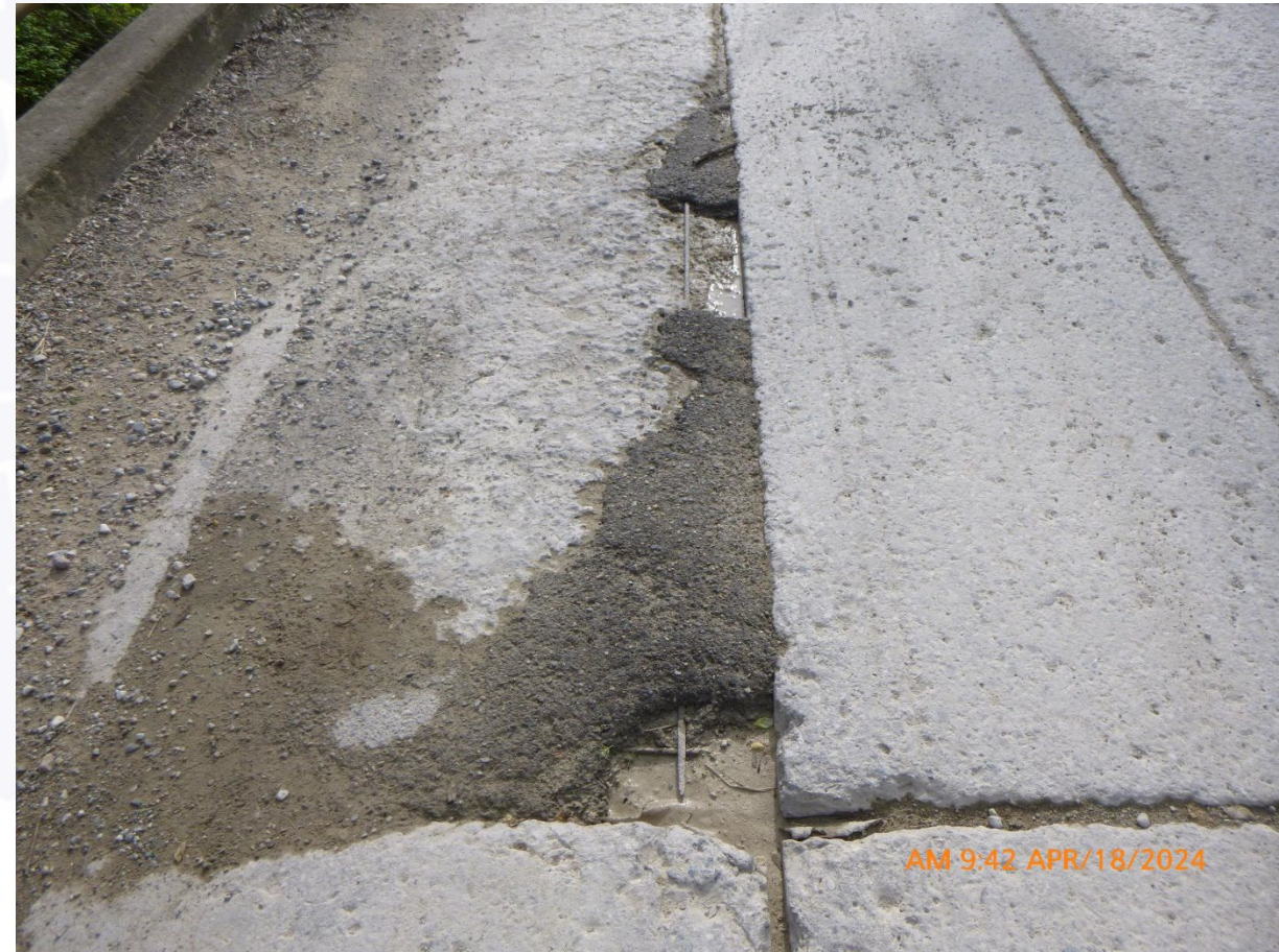
Exposed Steel that has been Partially Repaired
