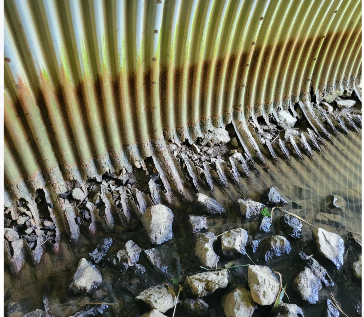
Rust Through at the Waterline
