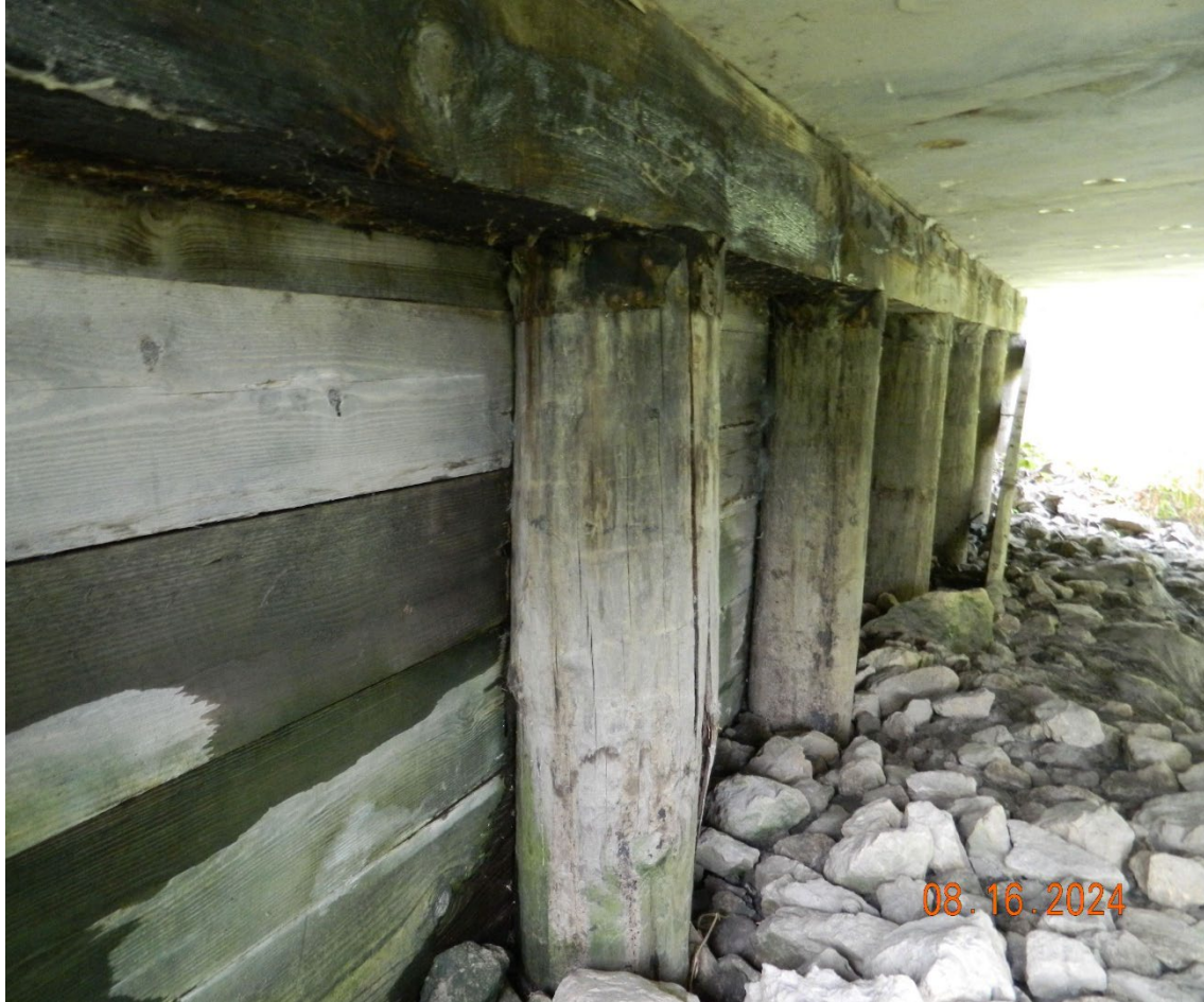
East Bent Piles
