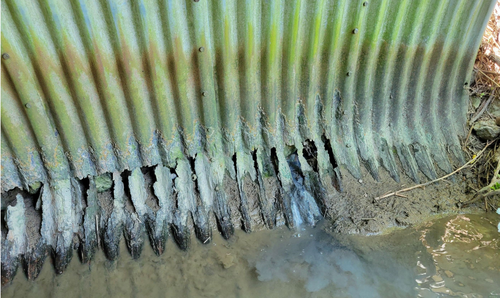
Rust Through at the Waterline
