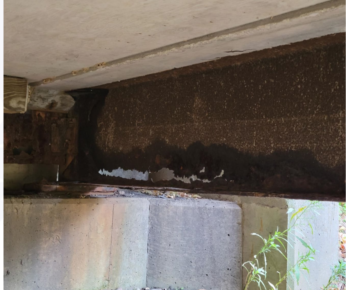
Rust Through of Beam 1A
