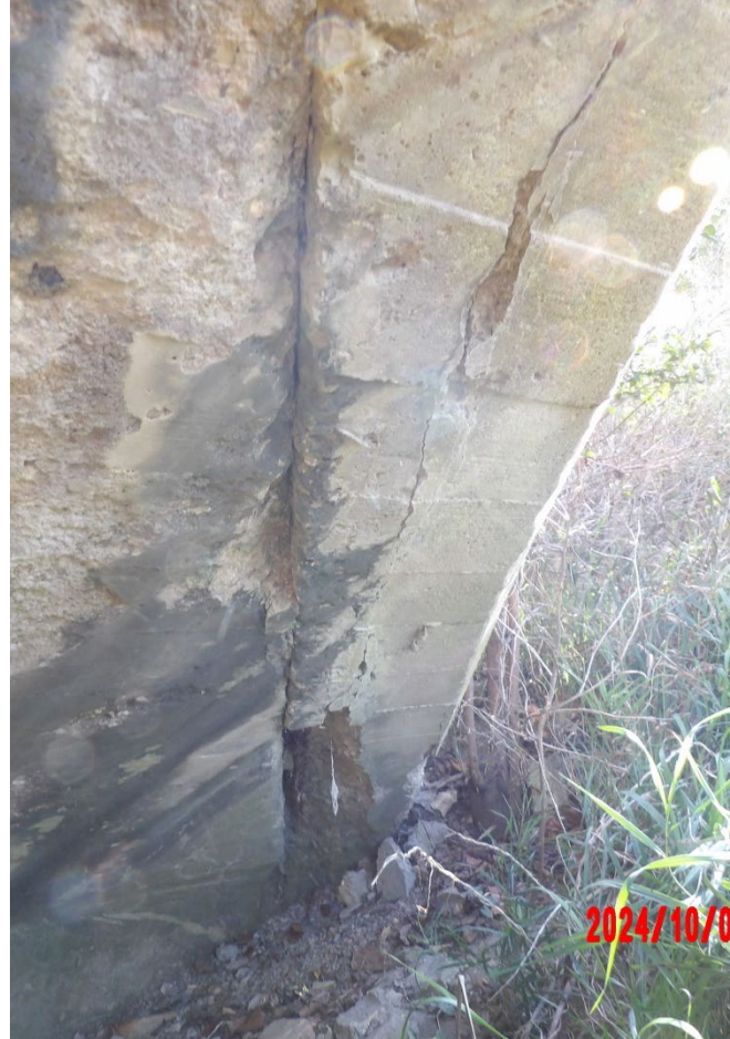
Spalling on the Southeast Coping
