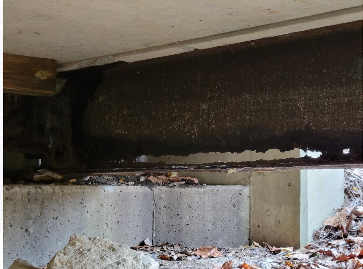
Rust Through of Beam 4C
