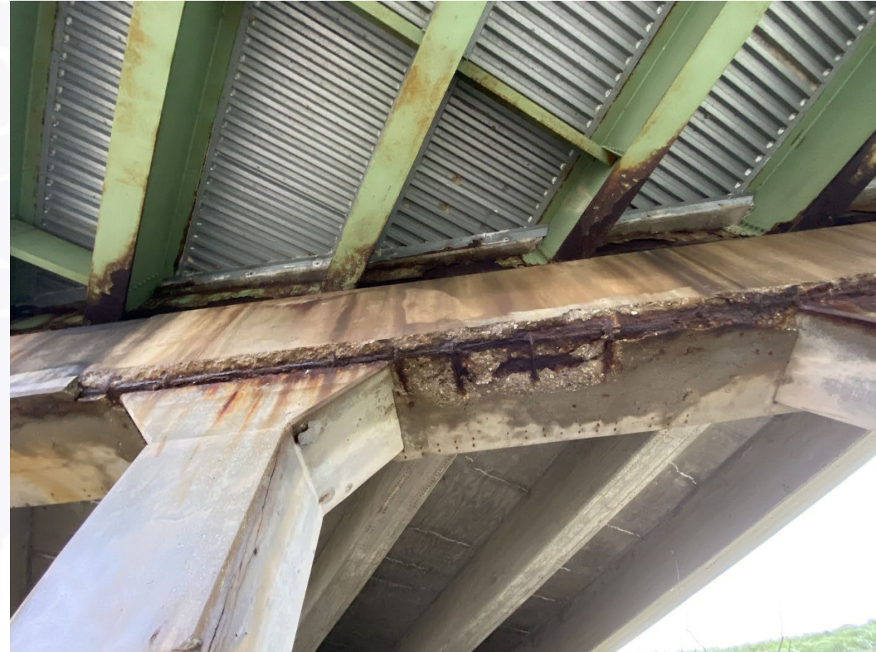
Exposed Steel on the Pier 2 Cap
