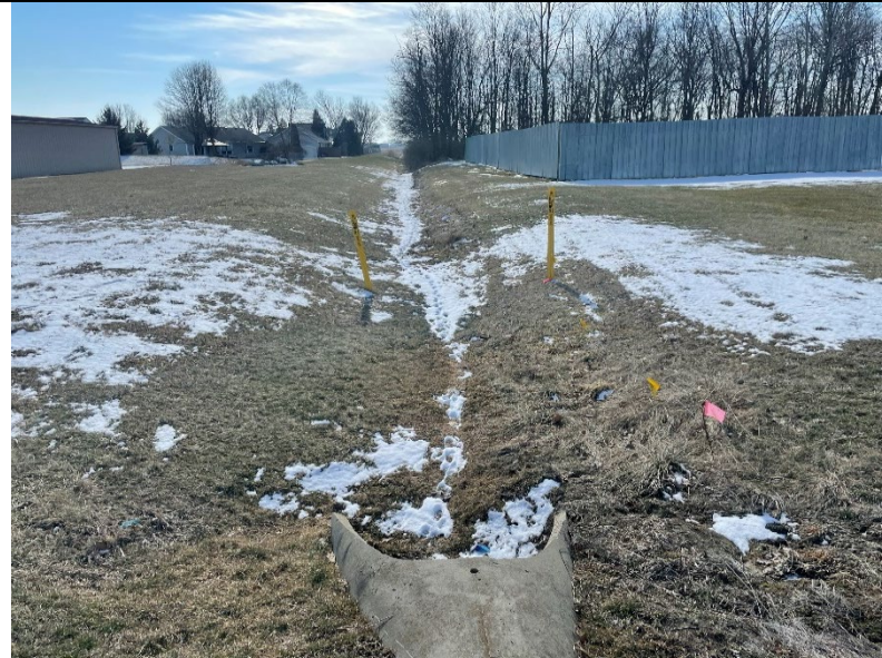
Photo 10: Facing south at UNT to Eagle Creek and culvert, located south of SR 47 (1/31/2021)
