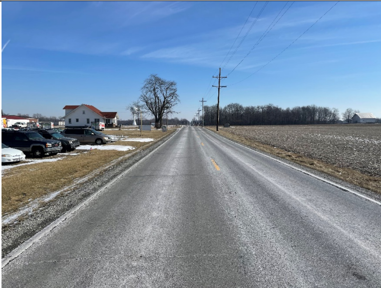
Photo 3: Facing east at SR 47 (1/31/2021)
