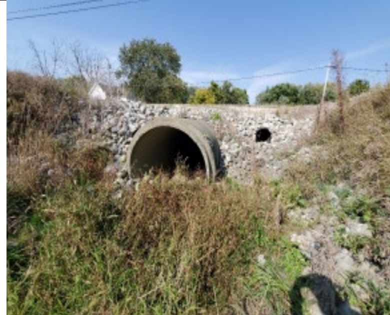
Photo 14: Facing northwest at Eagle Creek and culvert
