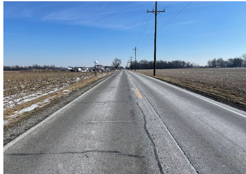
Photo 2: Facing east at SR 47 (1/31/2021)
