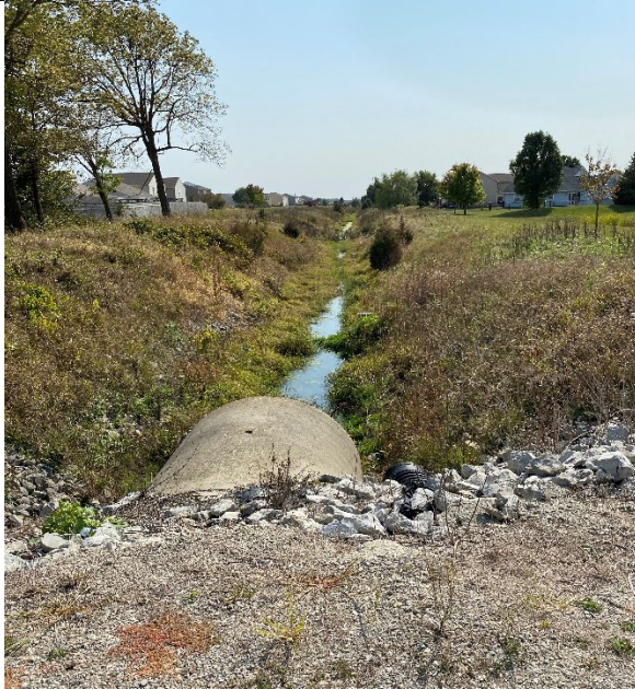
Photo 13: Facing south at Eagle Creek and culvert (10/6/2020)
