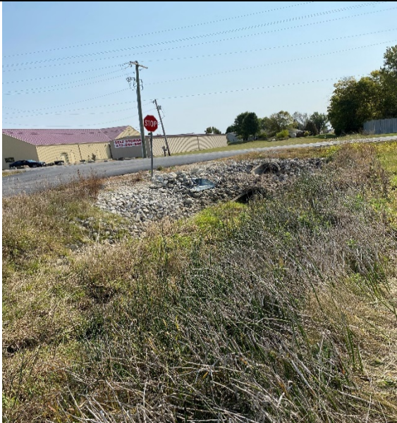
Photo 11: Facing southeast at UNT to Eagle Creek (10/6/2020)
