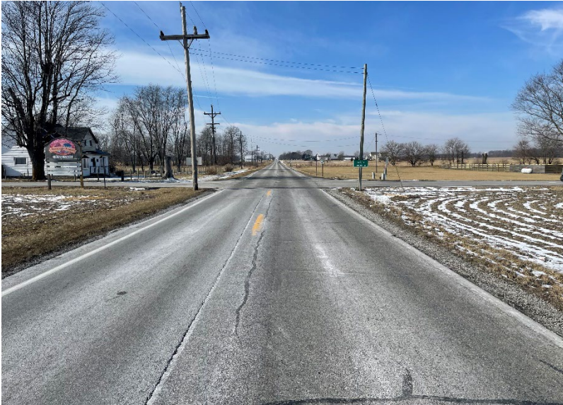
Photo 1: Facing west at SR 47 and the Boone/Hamilton County Line (1/31/2021)
