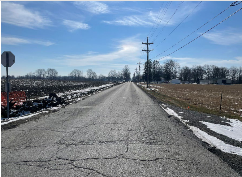
Photo 23: Facing south at Mule Barn Road (1/31/2021)
