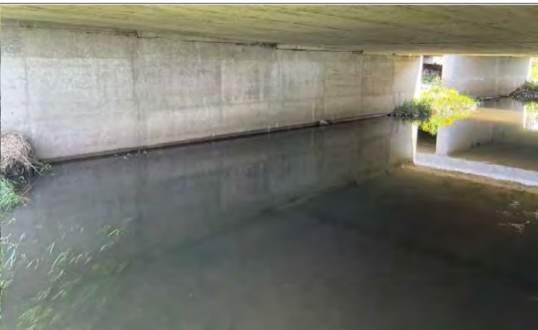
24. Looking southwest at the north concrete pylon under the US 41 NB bridge from the northeast bank of Mud Creek. There were no signs of bats or birds.
