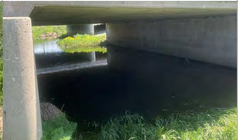
58. Looking northwest, from the northeast side of the US 41 NB bridge, along Mud Creek under the US 41 NB bridge.
