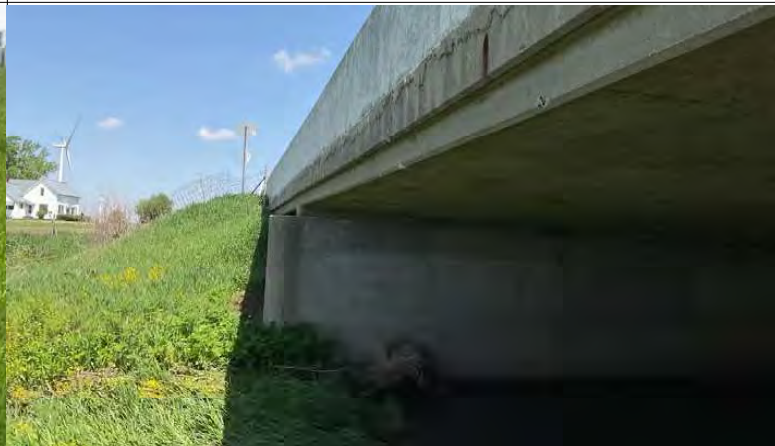
44. Looking northwest towards the US 41 NB bridge north bank of Mud Creek.
