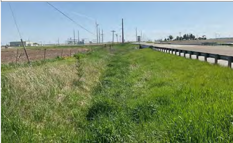
7. Looking south along RSD 7, on the east side of US 41 northbound (NB).
