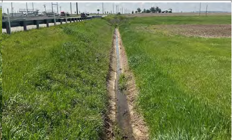
6. Looking south along RSD 2, toward Mud Creek, on the west side of US 41 SB.
