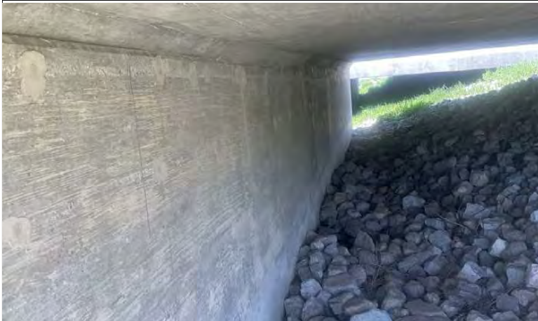
47. Looking west at the north concrete pylon of the US NB bridge. There were no signs of birds or bats. There was riprap on this side of the pylon up the slope under the bridge.
