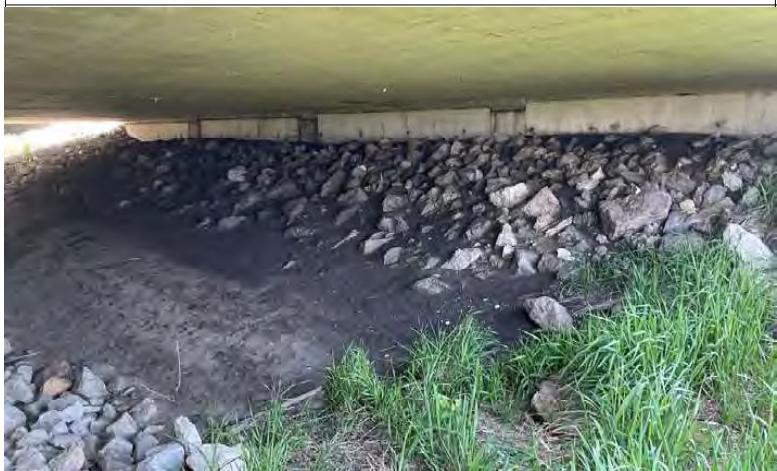
23. Looking northwest at the north concrete wall under the US 41 NB. There were no signs of bats or birds.
