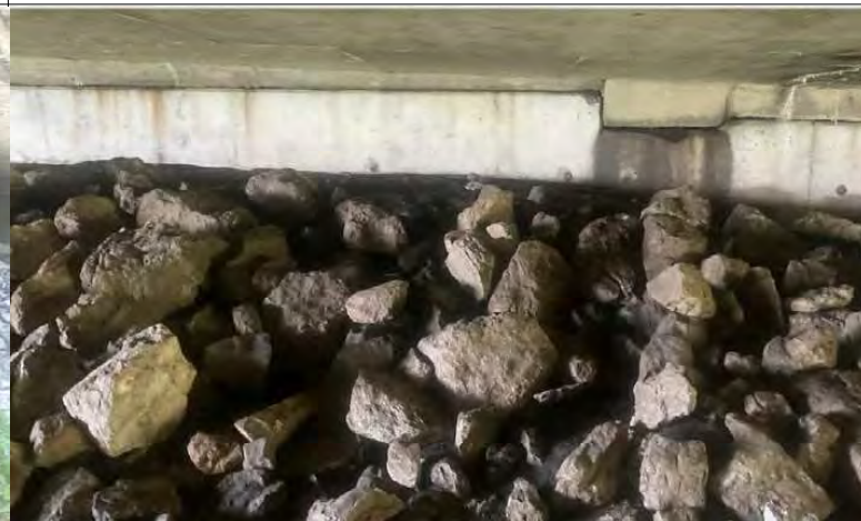
54. Looking northeast towards north wall of the US 41 SB bridge from the slope between the north pylon and the north wall of the bridge. There were no signs of birds or bats.
