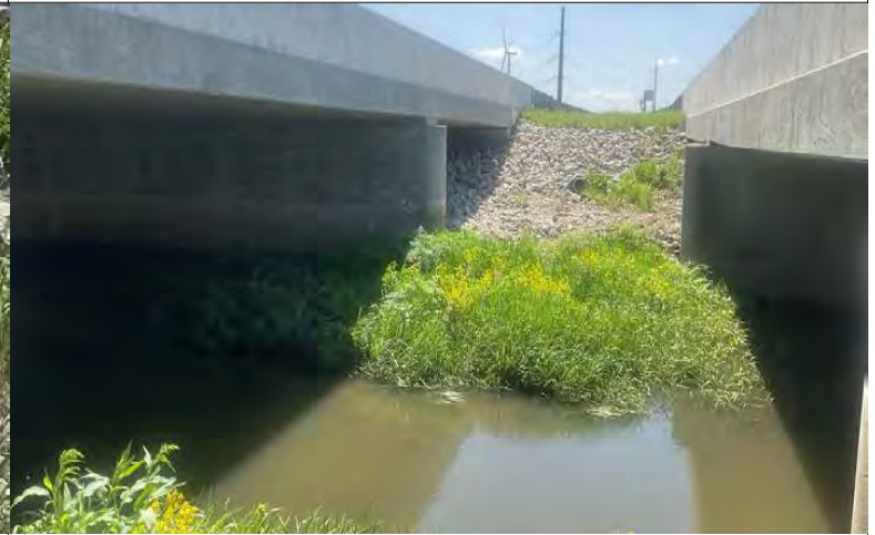
52. Looking south across Mud Creek towards south bank between both bridges.
