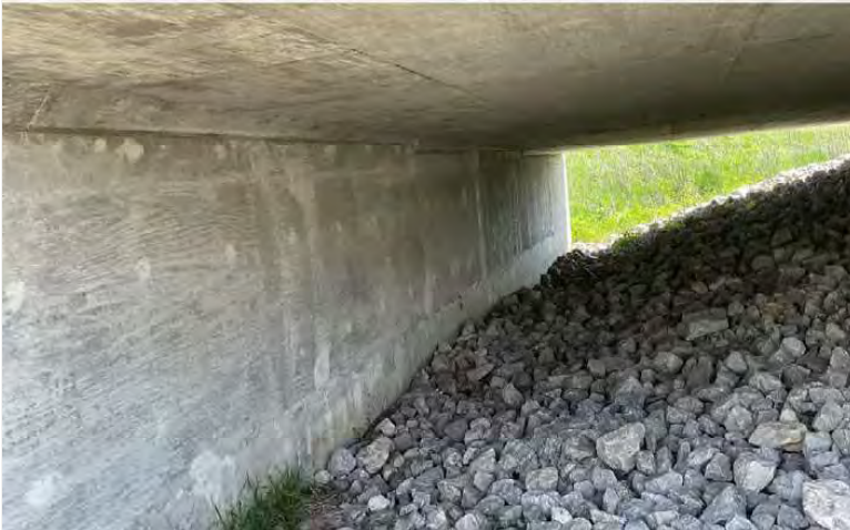
29. Looking southeast towards the north central concrete pylon of the NB US 41 bridge. There were no signs of birds or bats.
