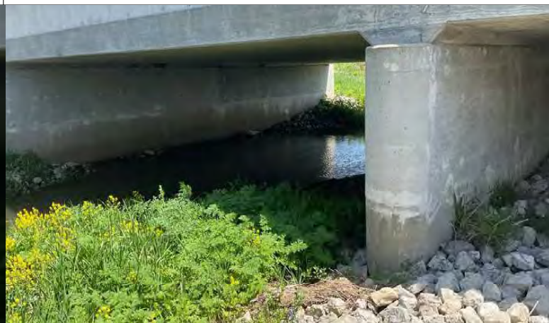
28. Looking northeast towards the east side of the north concrete pylon of the US 41 NB bridge. There were no signs of bats or birds.
