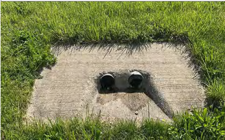
3. Looking east, at the underdrain outlet near RSD 1 on the west side of US 41 SB.
