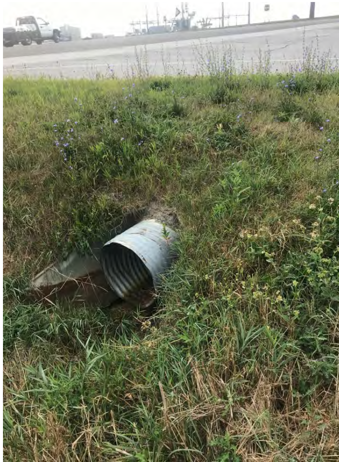
Photo 1. Culvert CLV-16825, a corrugated metal pipe, which is typical of all the culverts in this undertaking
