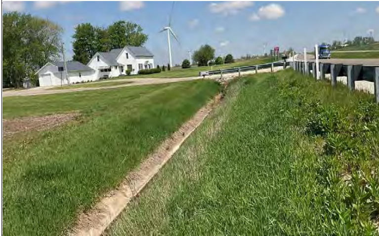
9. Looking north towards RSD 2, on the west side of US 41 SB.
