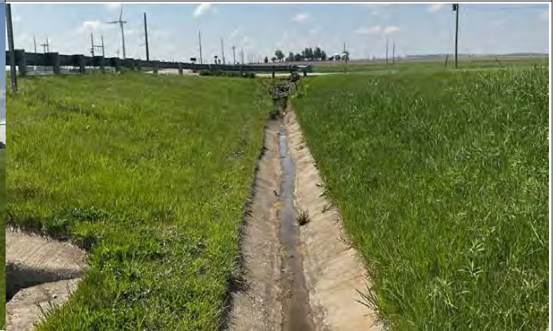
2. Looking south along RSD 1 on the west side of US 41 southbound (SB).
