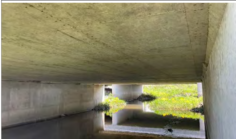
25. Looking east along Mud Creek from the west opening of the US 41 SB bridge through both bridges. There are no signs of bats or birds under the center of the US 41 SB bridge.
