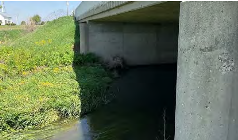
22. Looking north towards the north concrete pylon of the US 41 SB bridge.
