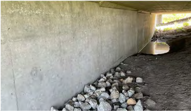
85. Looking southeast at the north pylon of the US 41 SB bridge from the northwest bank of Mud Creek.
