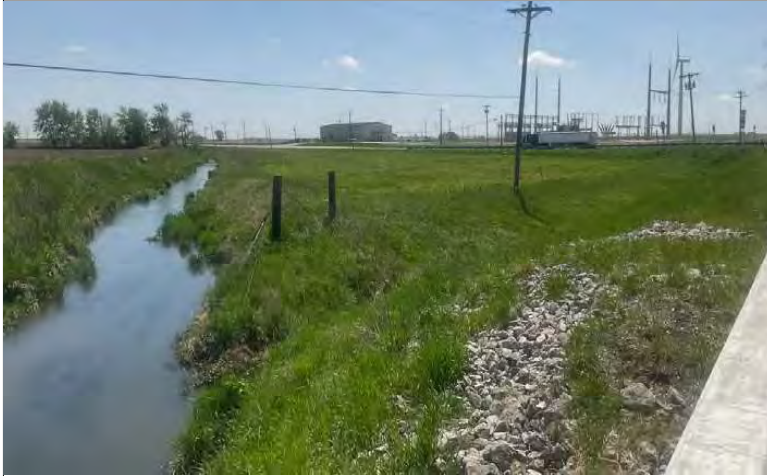
45. Looking east along Mud Creek from the east side of the US 41 NB bridge.
