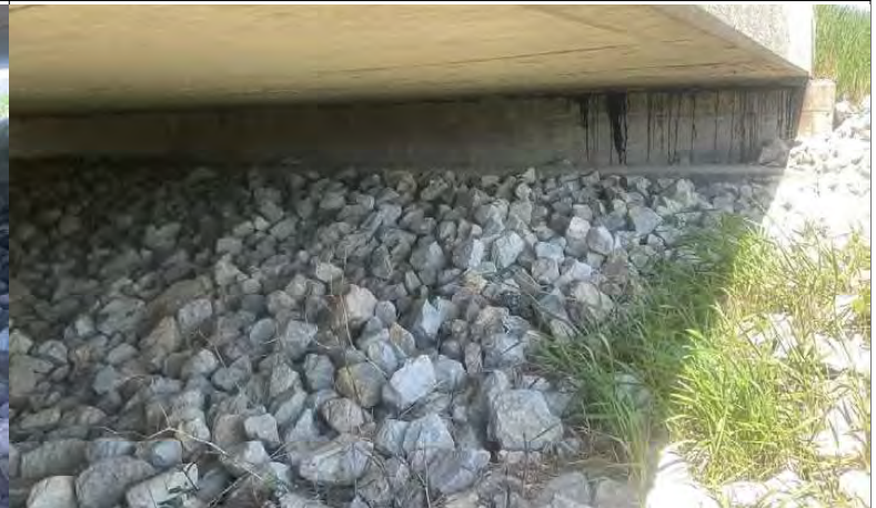
48. Looking north at the north wall of the US 41 NB bridge from the center of the bridges. There were no signs of birds or bats.
