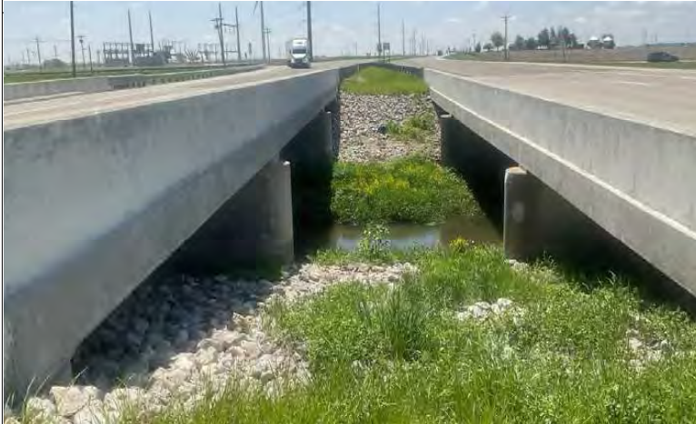
49. Looking south across the US 41 Mud Creek crossing of both bridges from the north Mud Creek bank
