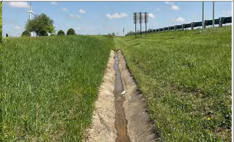
4. Looking north along RSD 1 on the west side of US 41 SB.
