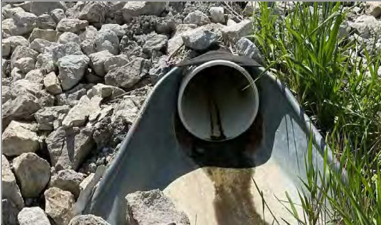
31. Looking south towards pipe on south bank slope between both bridges.
