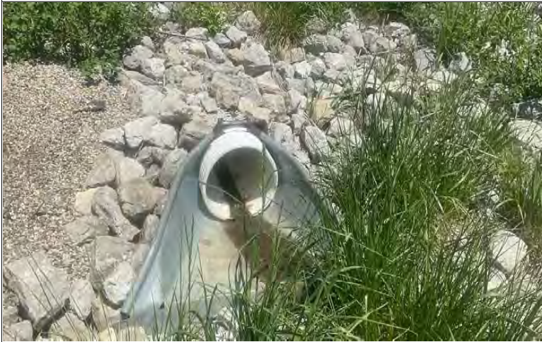
51. Looking north towards pipe on north bank slope between both bridges.
