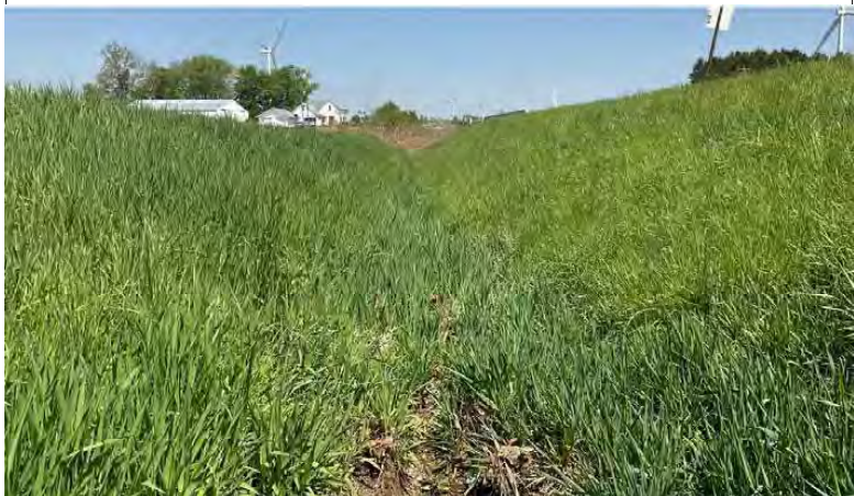
21. Looking north along RSD 3, on the west side of the US 41 SB bridge.
