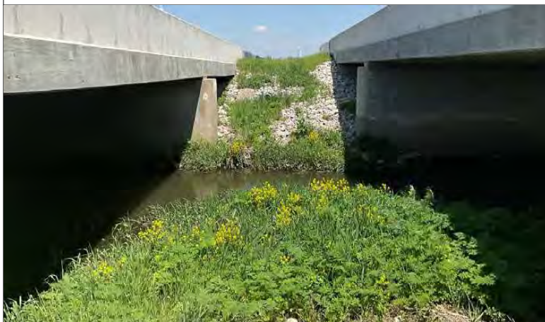
27. Looking north, at the north bank of Mud Creek, from the center of the south bank between both US 41 bridges.
