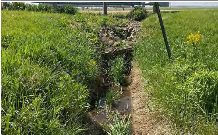
5. Looking south at the inlet of CLV 041-004-201.09, on the west side of US 41 SB.
