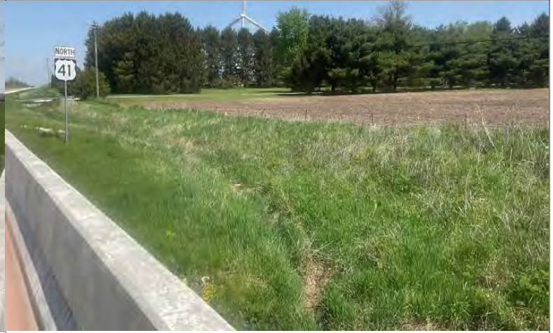
46. Looking north along RSD 7 from the northeast corner of the US 41 NB bridge.
