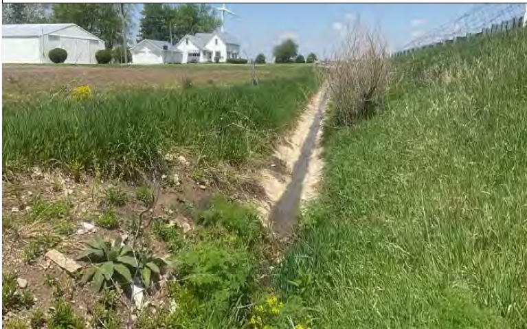
11. Looking north along RSD 2, on the west side of US 41 SB.
