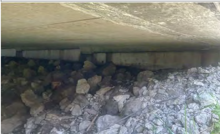
53. Looking north towards north wall of the US NB bridge from the slope between the north pylon and the north wall of the bridge. There were no signs of birds or bats.
