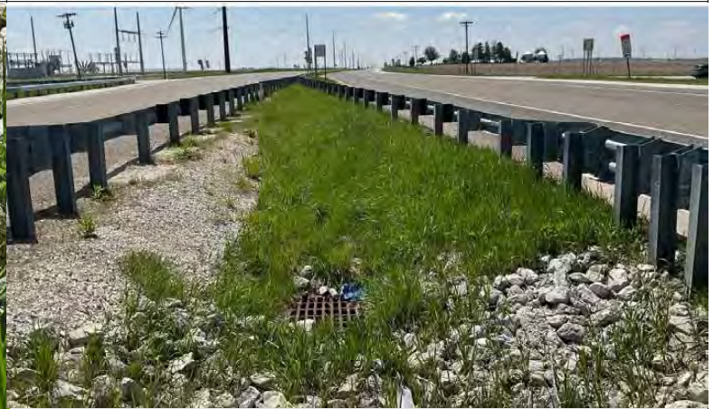
32. Looking south at the drain and grassy swale in the median between the guardrails of the bridges on US 41.
