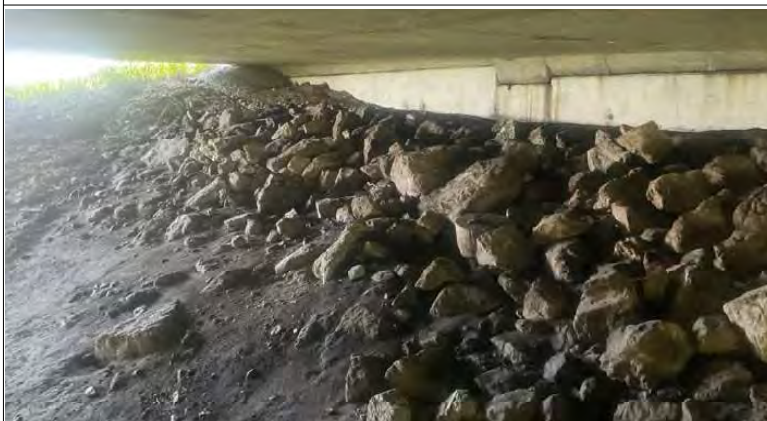
55. Looking southeast towards the south wall of structure of the US 41 SB bridge from the slope between the south pylon and the south wall of the bridge. There were no signs of birds or bats.
