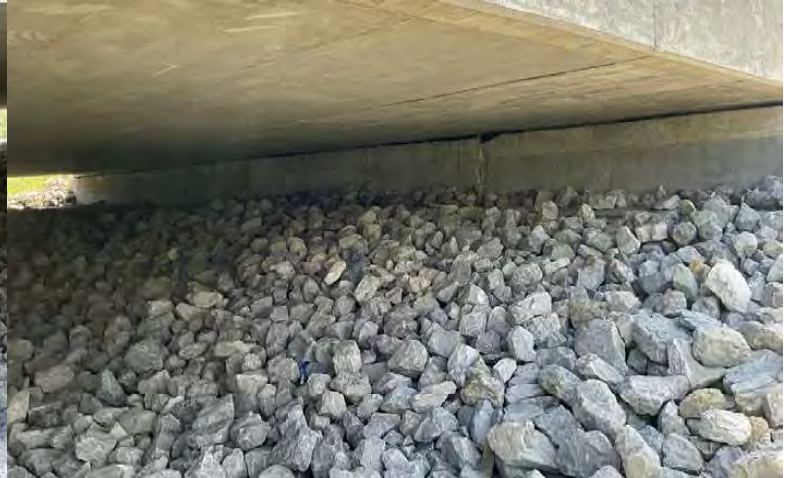
30. Looking south towards the south wall of the US 41 NB bridge. There were no signs of birds or bats.
