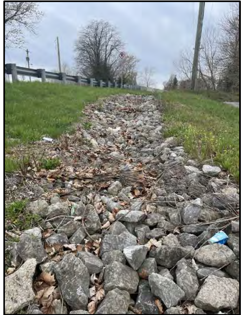
24. View of riprap lined ditch looking west along SR 252. 4/20/2022
