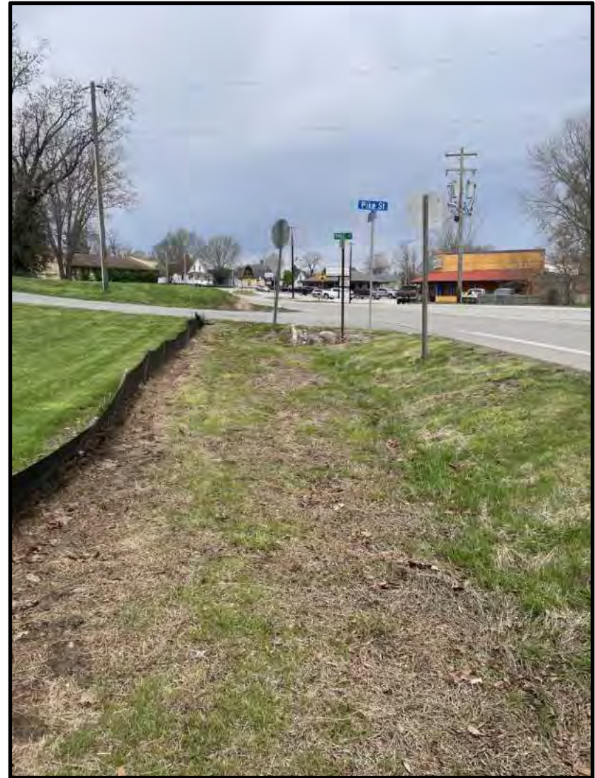
22. View of drainage swale connecting Wetland A to Wetland B, looking northwest along SR 135. 4/20/2022
