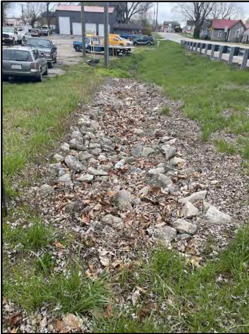
23. View of riprap lined ditch looking east along SR 252. 4/20/2022
