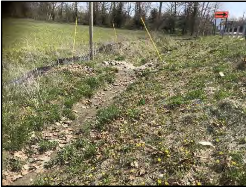
21. View of RSD1 looking southeast. 4/20/2022
