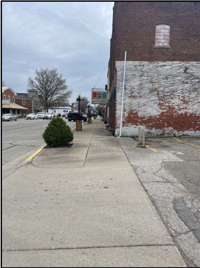
25. View East along Washington Street. 4/20/2022
