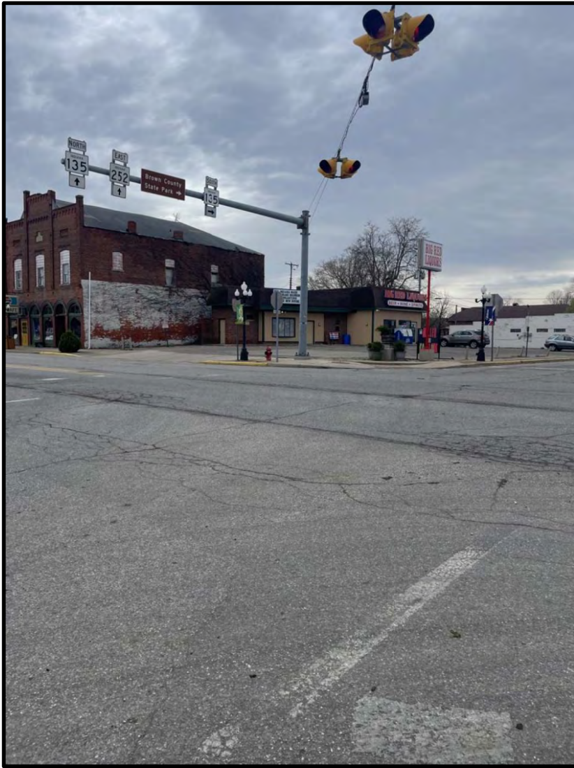
29. View Southeast along Washington Street. 4/20/2022
