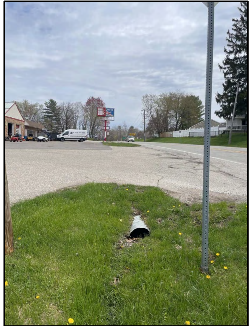
6. View East along SR 135. 4/20/2022
