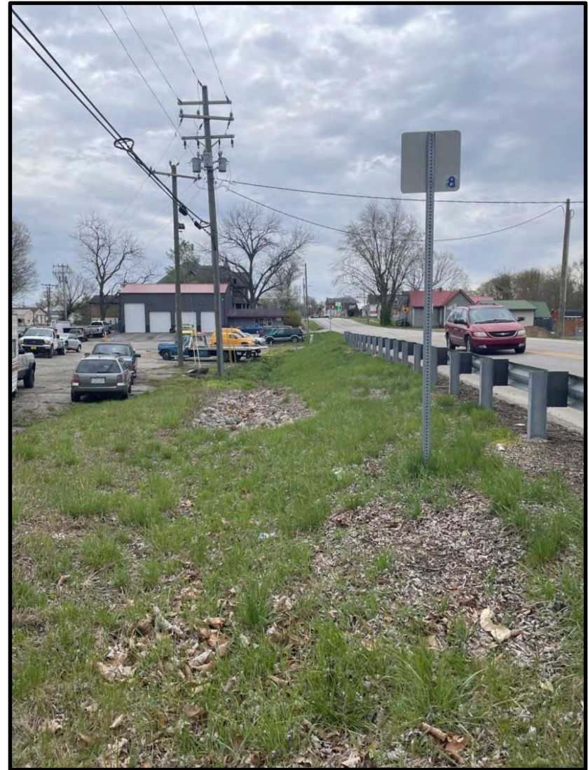
42. View East along Washington Street. 4/20/2022
