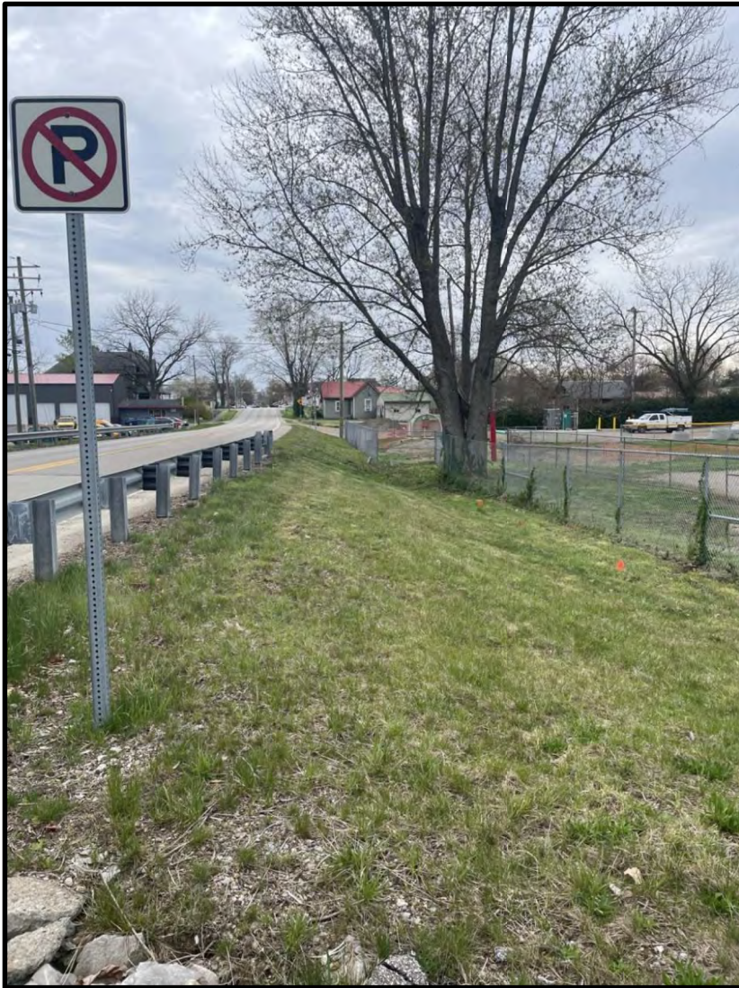
43. View East along Washington Street. 4/20/2022
