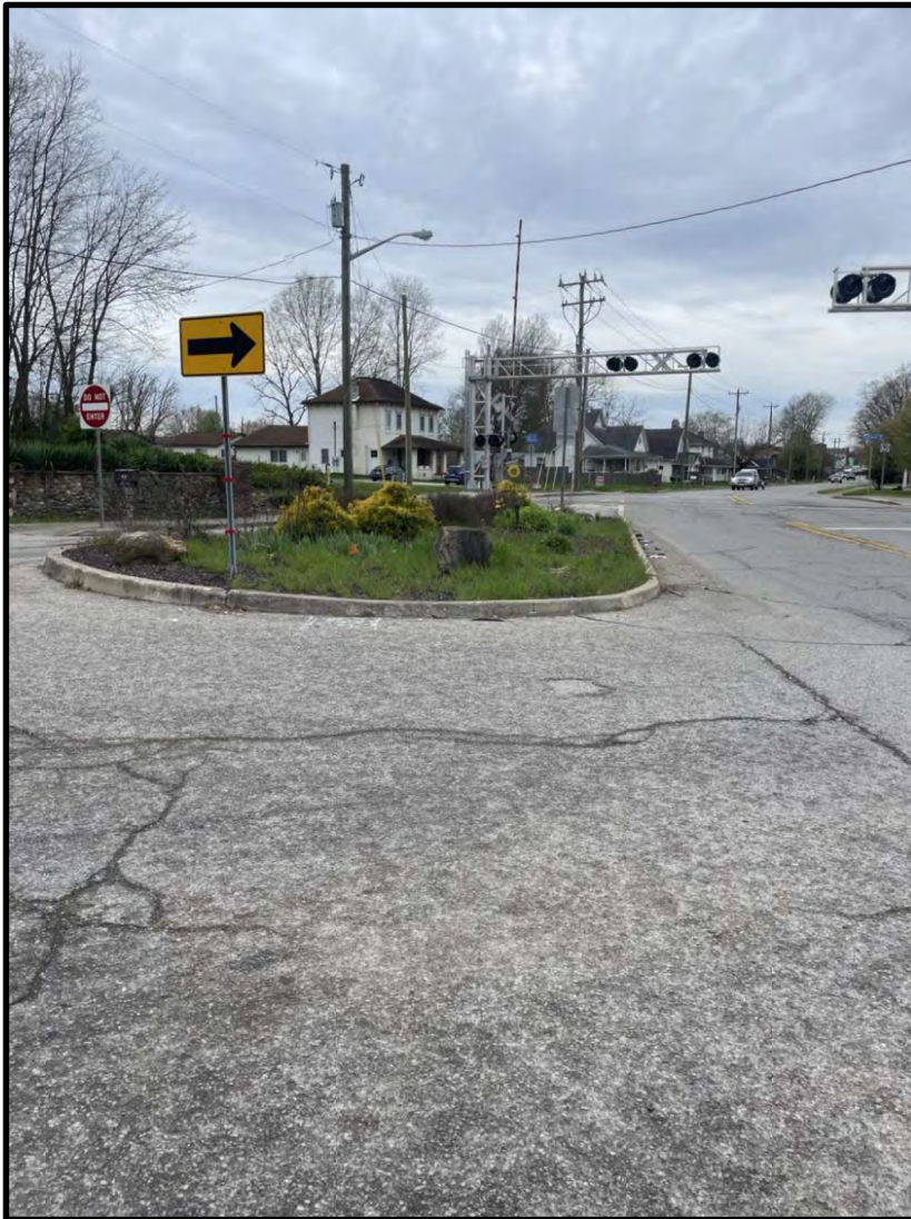
5. View Southwest along SR 135 toward Washington Street. 4/20/2022
