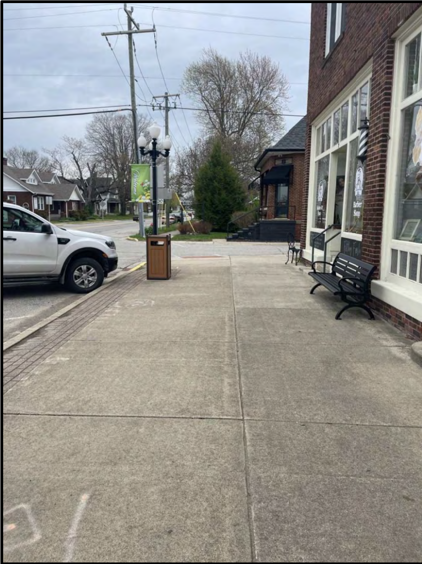
21. View East along Washington Street. 4/20/2022
