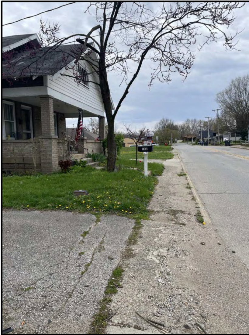
53. View South along Marion Street. 4/20/2022
