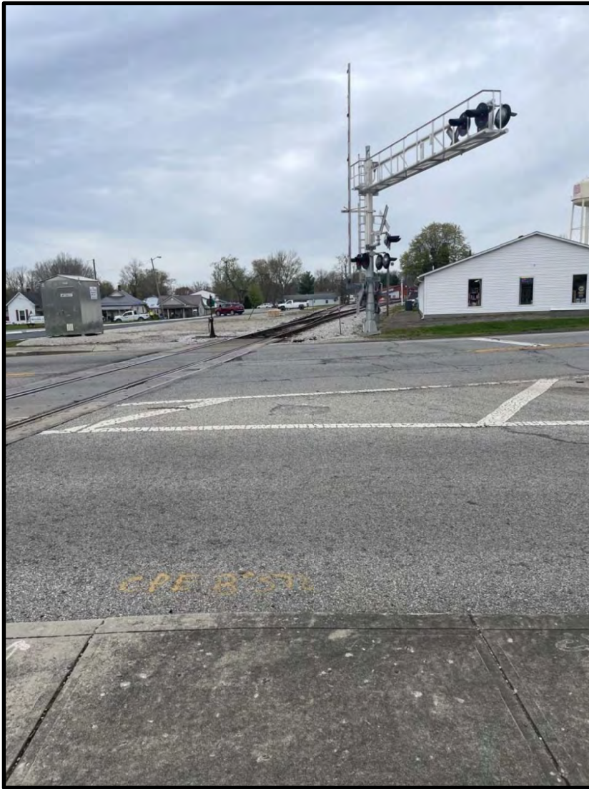
9. View North towards railway from SR 135. 4/20/2022
