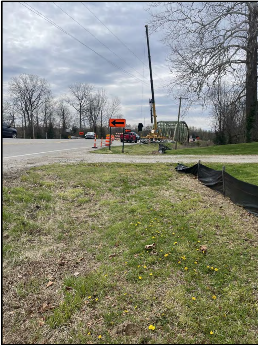
65. View Southeast along SR 135 toward existing bridge over Indiana Creek located outside study area 4/20/2022
