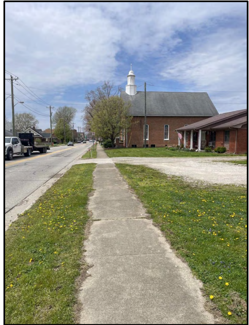
14. View West along Washington Street facing Chapel. 4/20/2022
