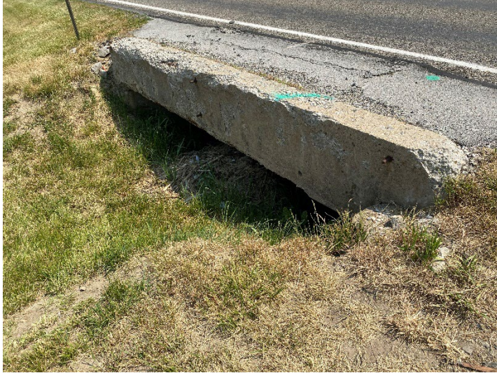
Photo 3: The small structure is showing effloresce.
