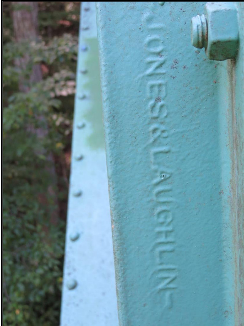
Figure 12. Detail of a vertical, steel member of the bridge (P000-40-07088 B; NBI No. 060380) featuring the embossing of "JONES & LAUGHLIN," looking south.
