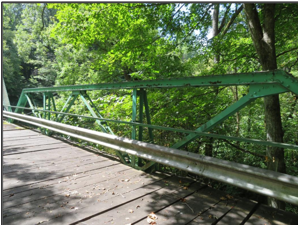
Figure 11. Detail of the approach span of the bridge (P000-40-07088 B; NBI No. 060380) showing the Warren truss, looking southwest.
