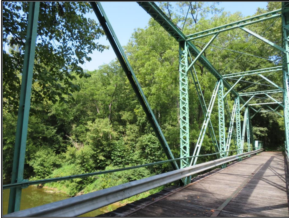
Figure 10. Detail of the main span of the bridge (P000-40-07088 B; NBI No. 060380) showing the Parker truss, looking northwest.
