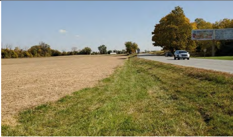
5. Northwest corner of SR 32 and CR 925 W.
