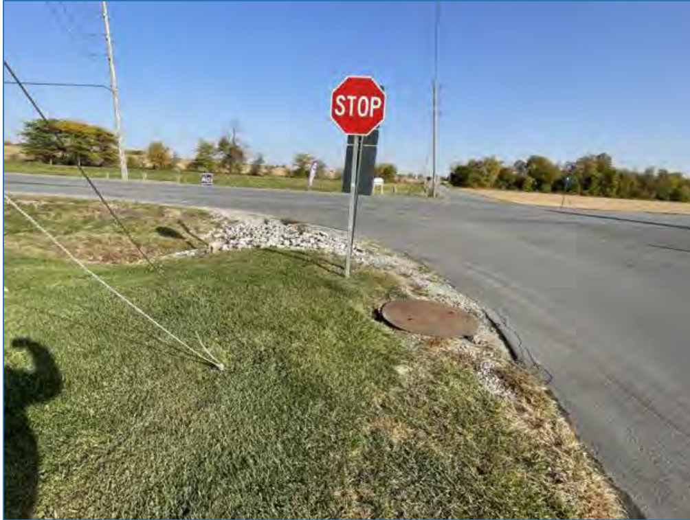
Photo 11. View toward the intersection of CR 925 W and CR 32, from the southwest quadrant of the intersection, facing north.
