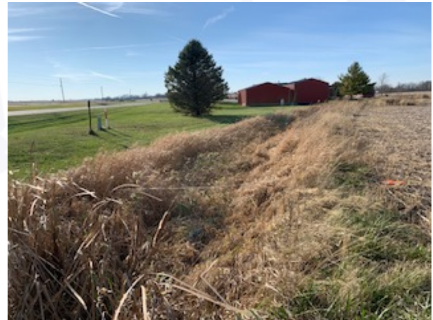
Dry Grass Swale, Hendricks County, Indiana
