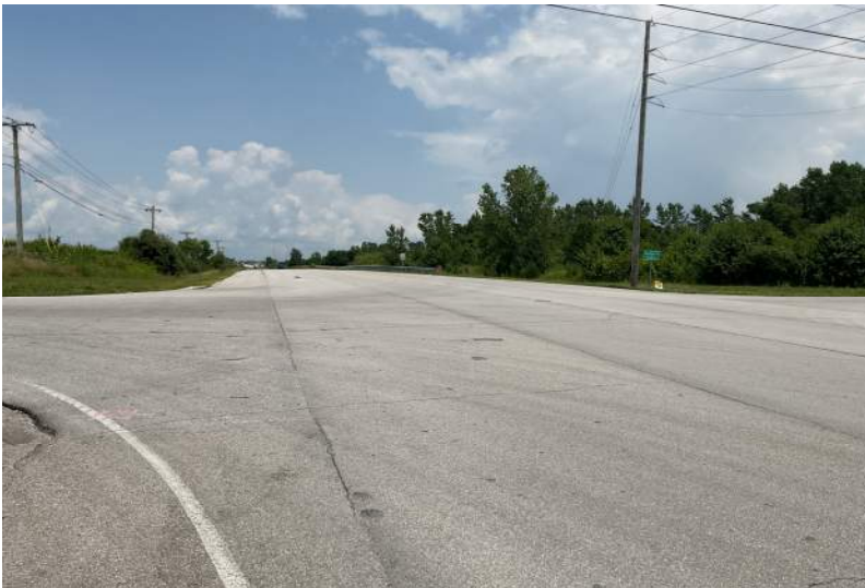
6. Looking northeast at SR 39 from southwest corner of SR 39 and Keller Hill Road intersection.
