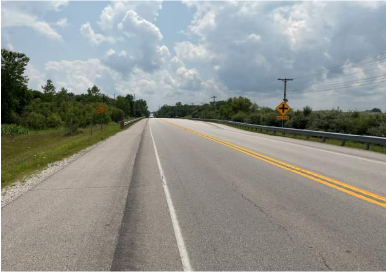
17. Looking south at SR 39, northern terminus of project area.
