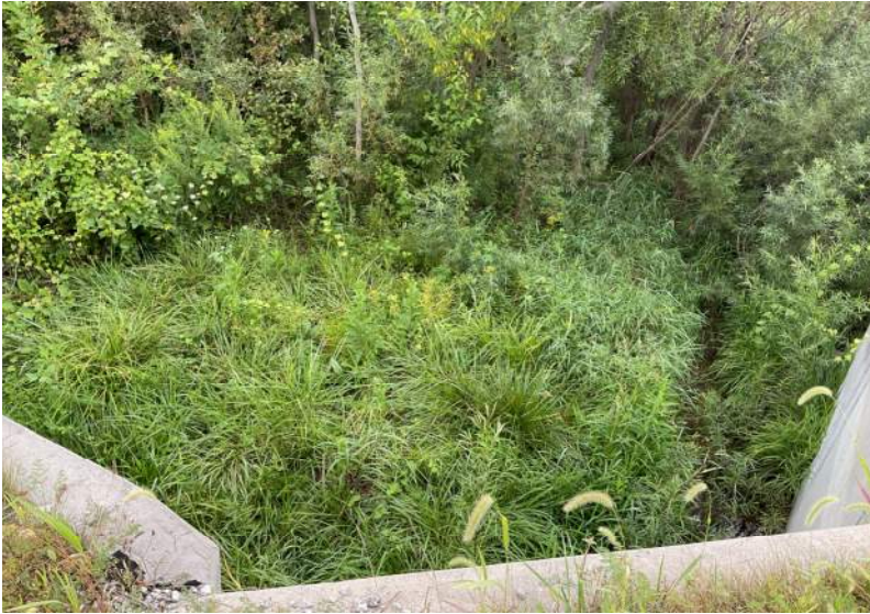
13. Facing west (upstream) looking at UNT 1 to McCracken Creek.
