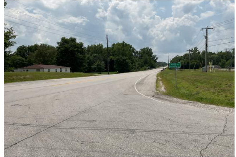
7. Looking southeast at SR 39 from northwest corner of SR 39 and Keller Hill Road intersection.
