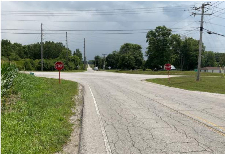
2. Looking east at the SR 39 and Keller Hill Road intersection, from the northwest corner on Keller Hill Road.
