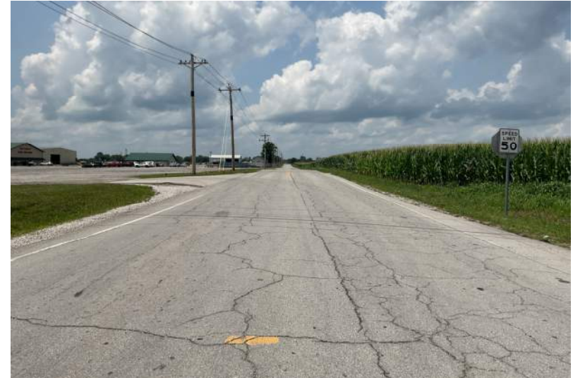
3. Looking west at Keller Hill Road from western edge of SR 39 and Keller Hill Road intersection.
