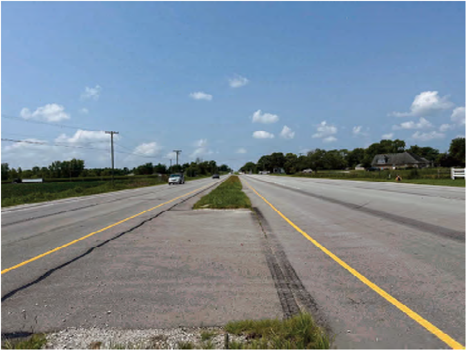
20. Looking west within the median of US 40
