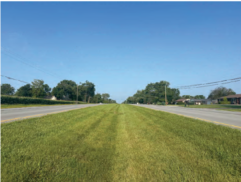
2. Looking west within median of US 40
