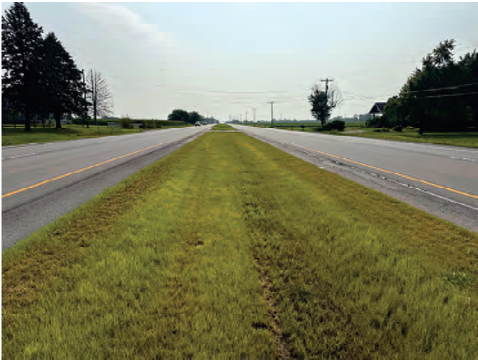
23. Looking east along US 40 from the median
