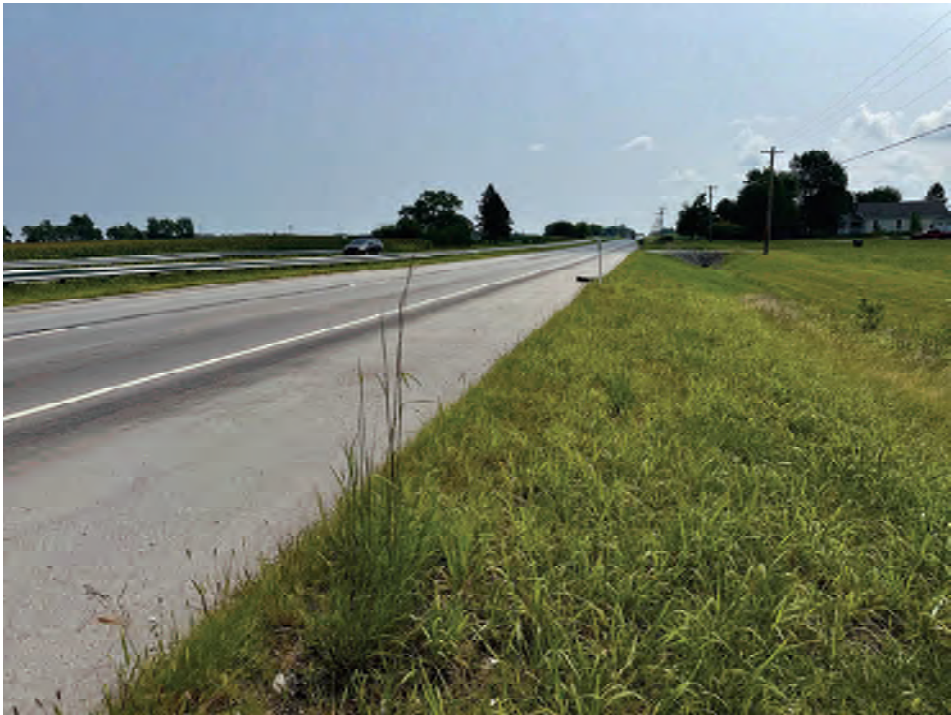
21. Looking east along US 40 from Bridge #040-30-08072 AEBL
