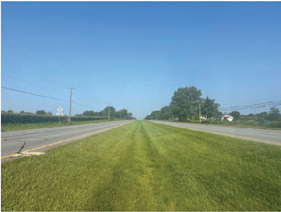
3. Looking west within median of US 40
