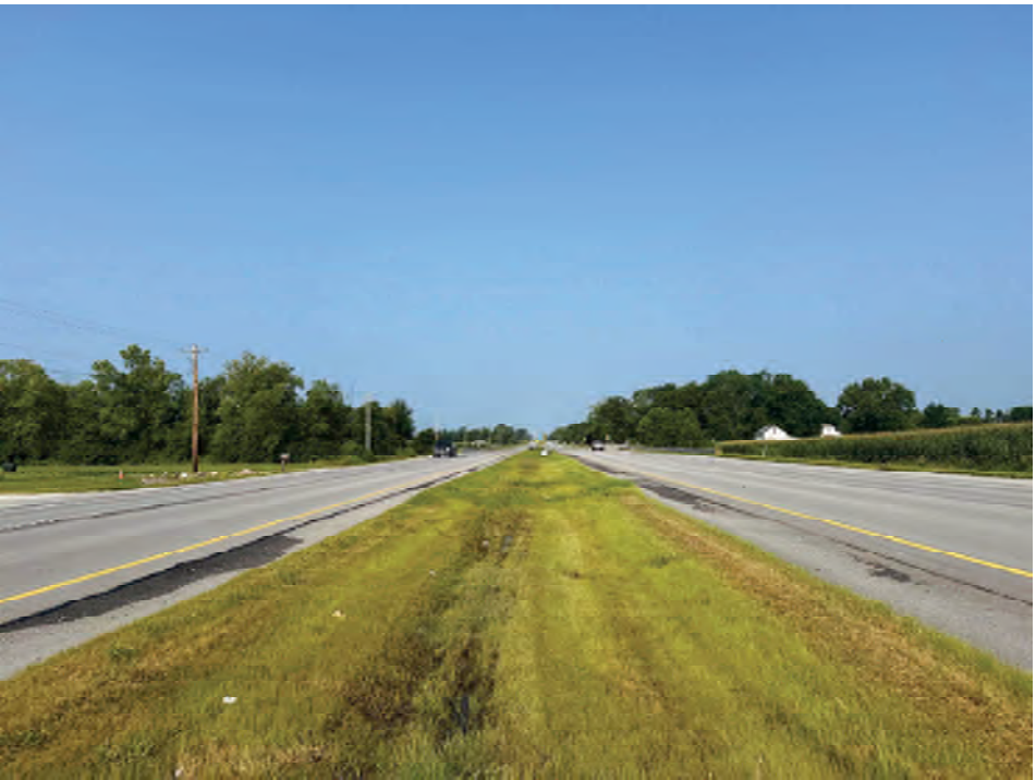
24. Looking west within the median of US 40
