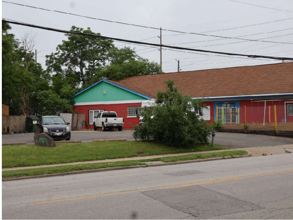
Photograph 13. View along Rural Street north of Brookside Avenue, looking northwest and showing a Non-Contributing day care building.
