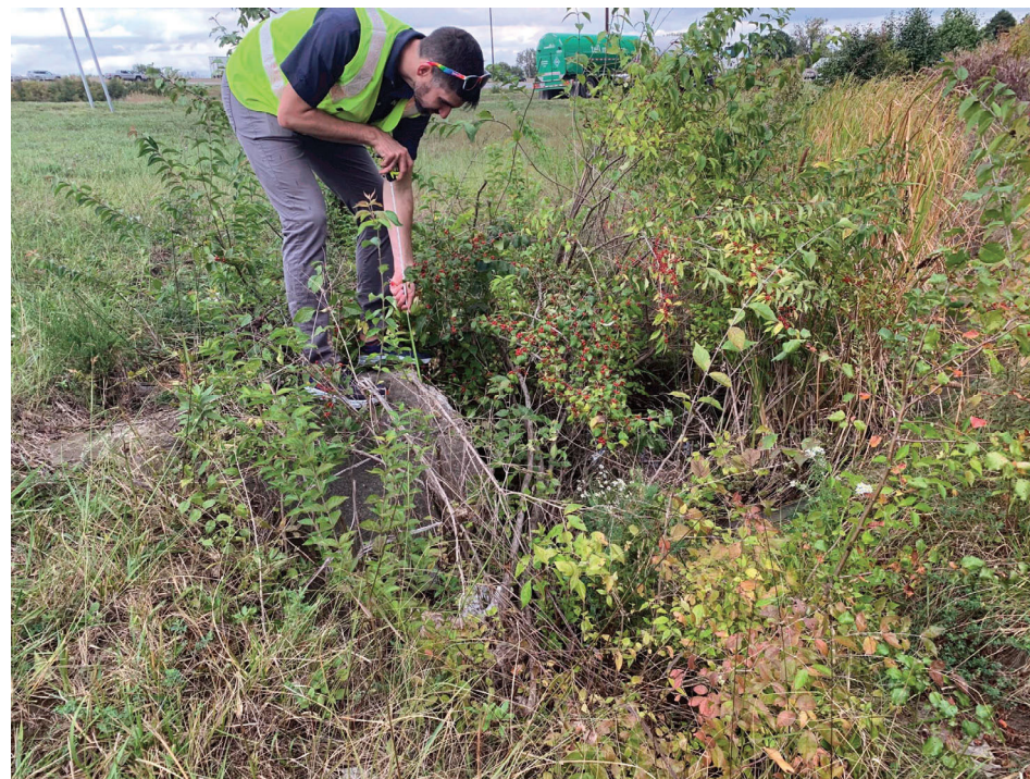
20. Facing northeast at RCP culvert inlet on east side of Rural St.
