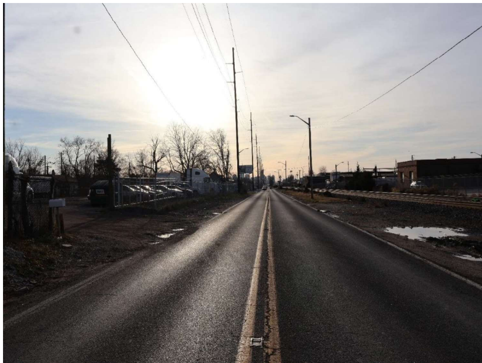
Photograph 6. View along Massachusetts Avenue from the eastern edge of the APE, looking southwest.
