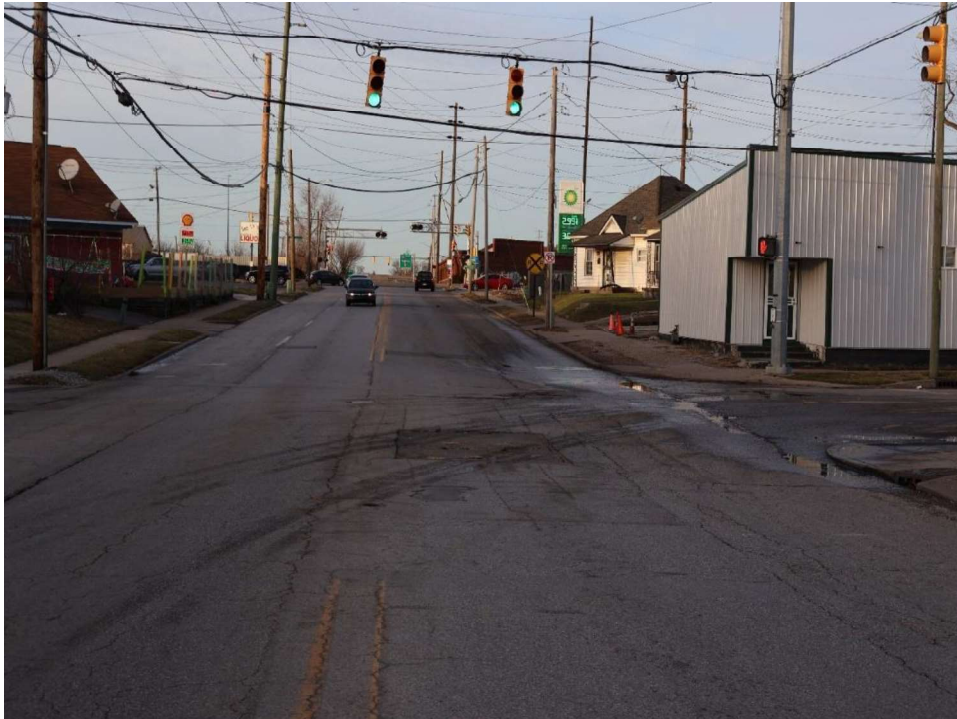
Photograph 2. View along Rural Street from E. Brookside Avenue, looking north.
