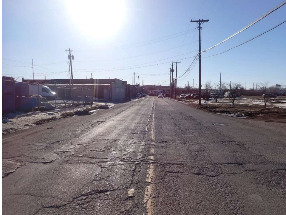
Photograph 9. View along Roosevelt Avenue from 2917 Roosevelt Avenue (IHSSI # 098-295-10171), looking southwest.
