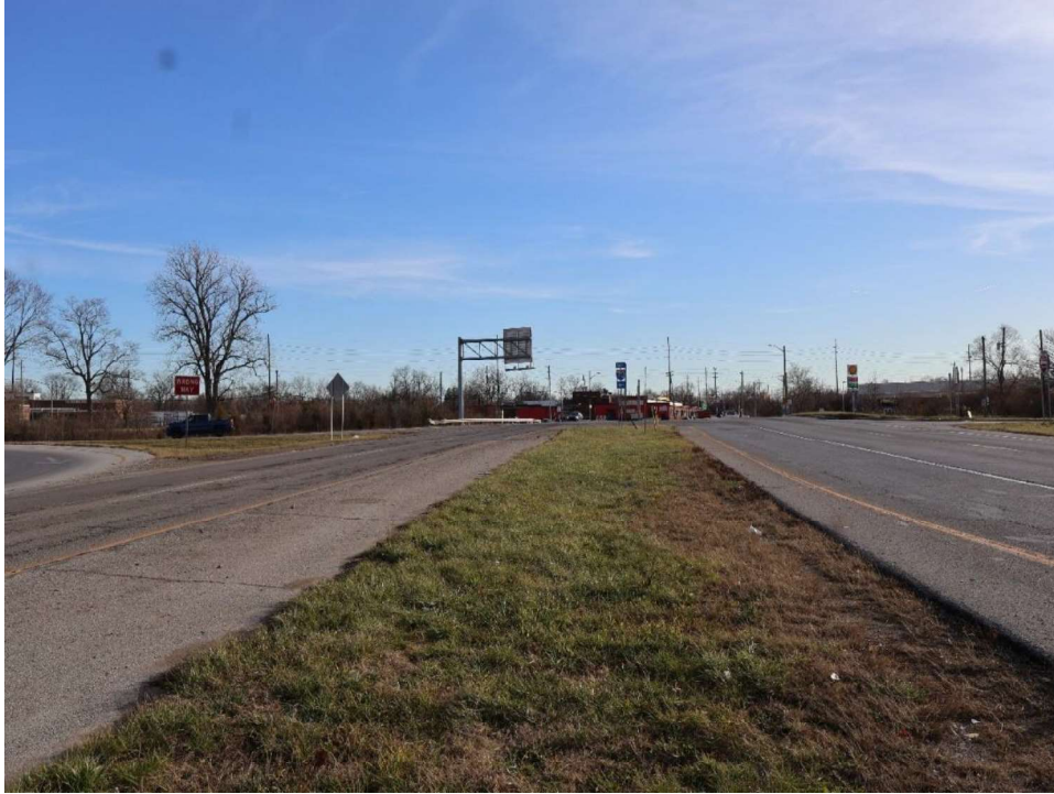
Photograph 1. View along Rural Street from I-70, looking southeast.
