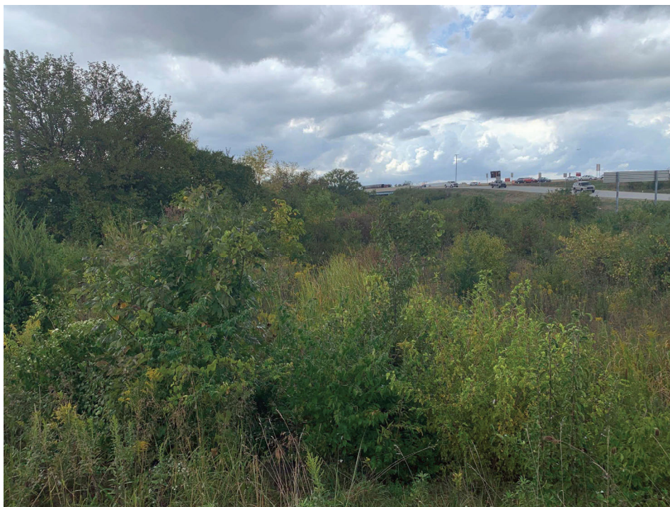
19. Facing west at vegetated area at RCP culvert outlet.
