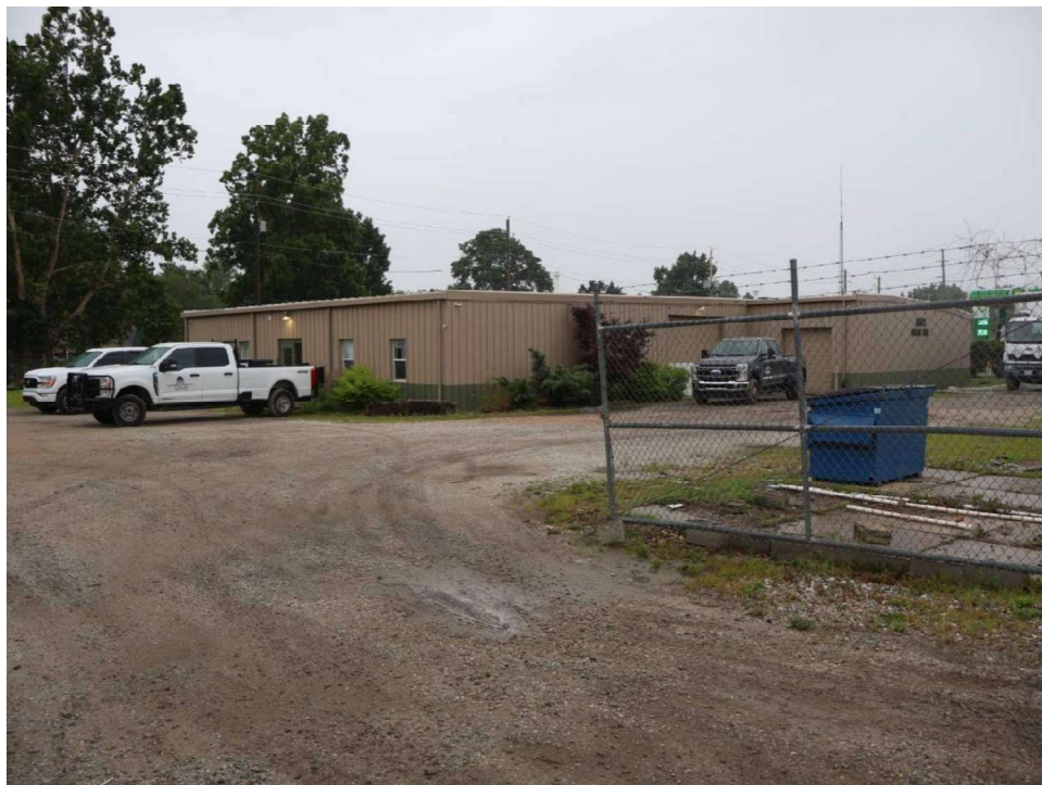
Photograph 16. View along Massachusetts Avenue, looking south and showing a Non-Contributing warehouse/office building.
