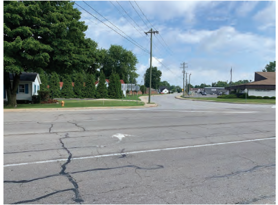
34. Looking north across US 36 toward SR 13
