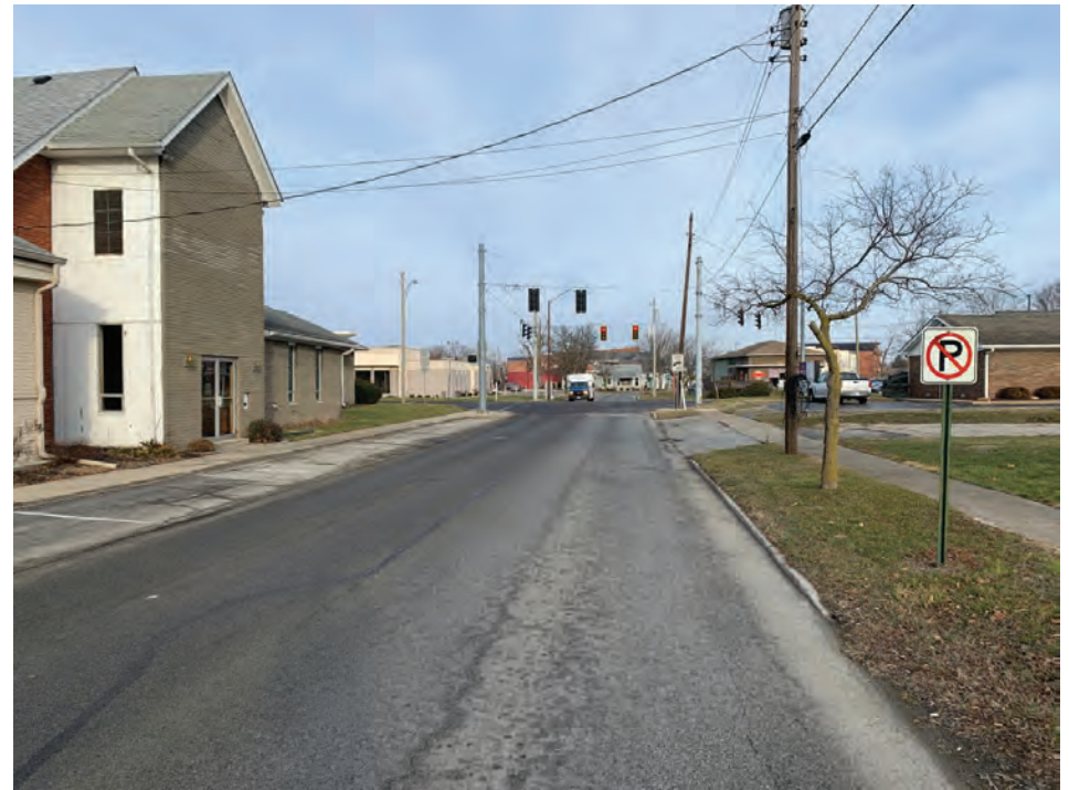
18. Looking north along Maple Street
