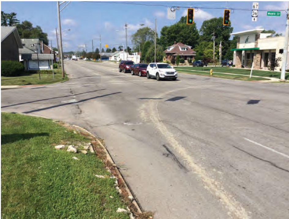
17. Looking southwest at intersection of US 36 and Maple Street
