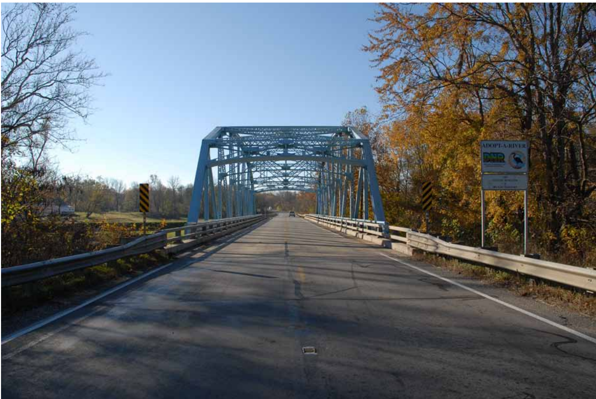
2. The north elevation of the Parker through truss bridge (NBI No.: 24970).
