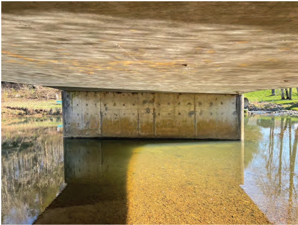
Mid-channel pier and slab deck of Union Chapel Road bridge at Buck Creek - 4/1/2022
