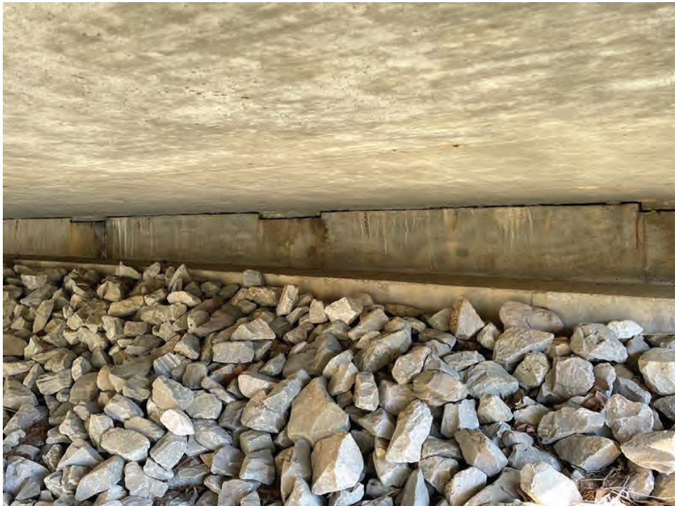
Riprap bank protection and low height abutment at Union Chapel Road bridge at Buck Creek - 4/1/2022
