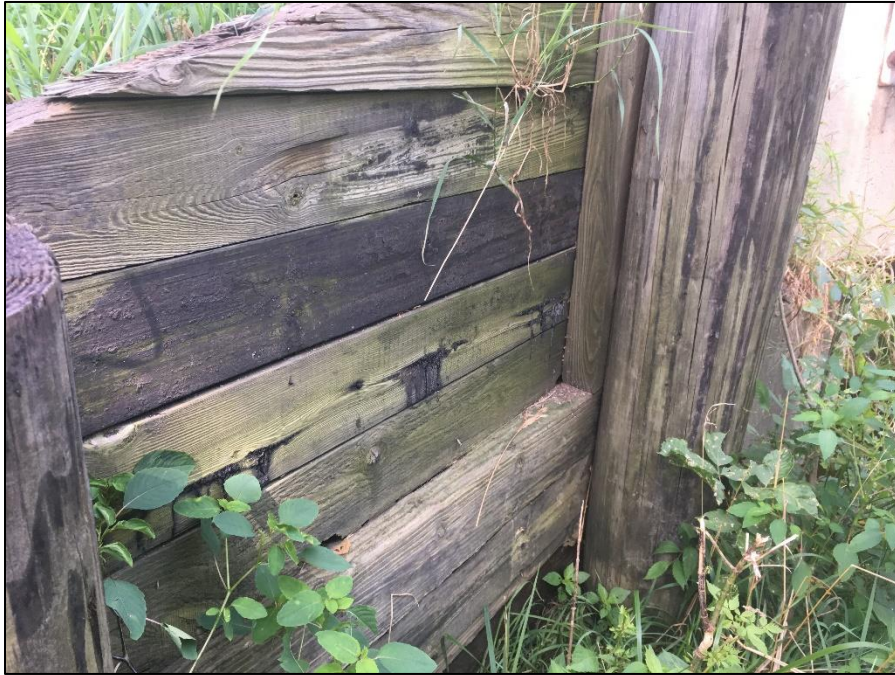
Figure 3: Timber wingwall
