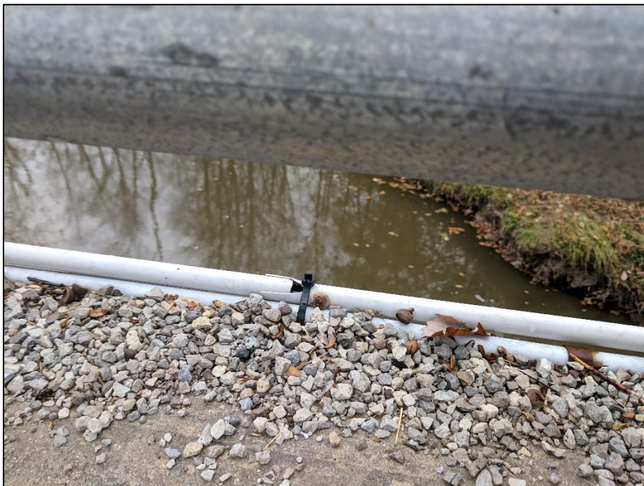
Figure 10: Utility attached to structure
