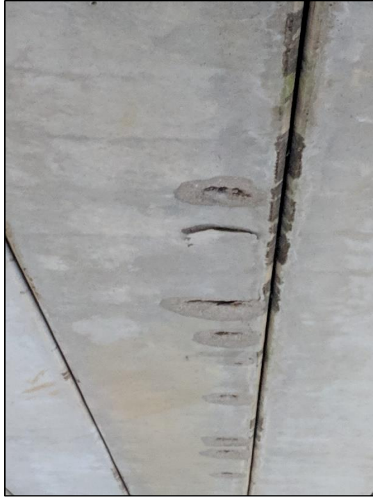
Figure 5: Prestressed box beam spalling and moisture between girders
