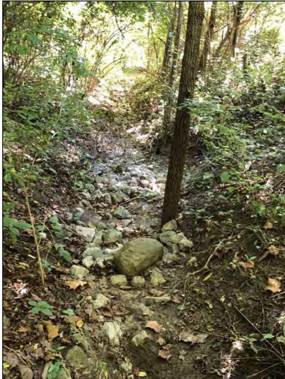
Picture 41—RSD1 riprap area—note medium-sized tree ( Juglans ) in bed; southeast view; 1 SEP 2021.
