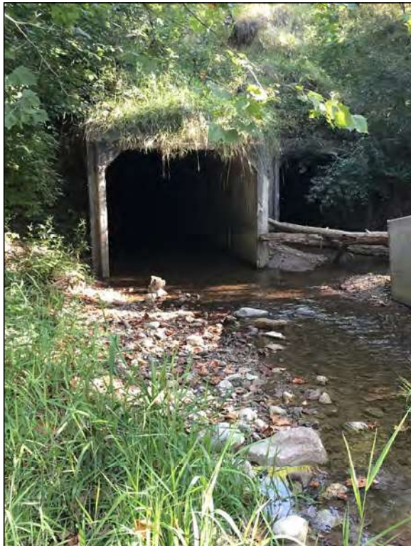
Picture 1—Goose Creek upstream and west project structure CV 026-079-28.10 , north view; 1 SEP 2021.
