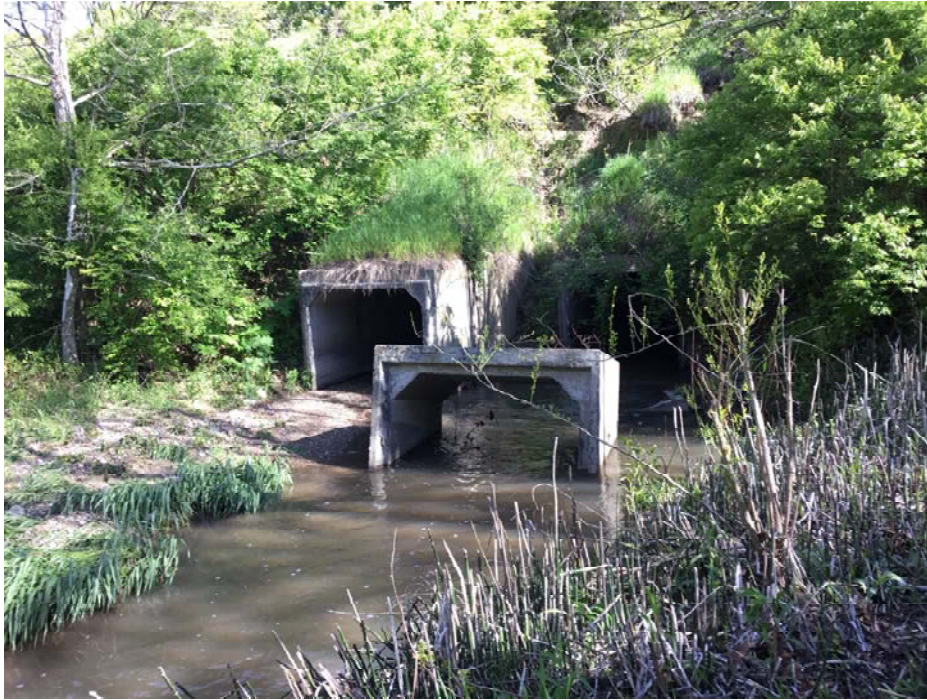
PHOTO 13 Condition Description Down stream alignment looking North or up stream
