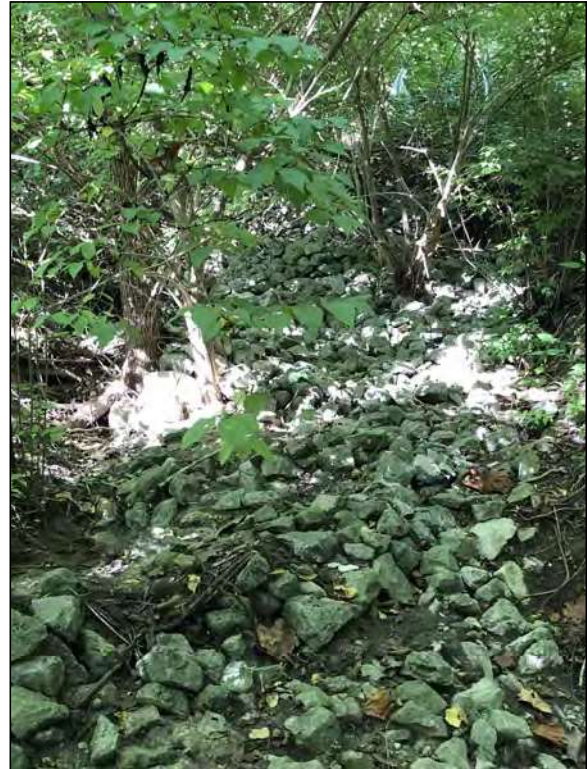
Picture 42—RSD1 riprap area; southwest view; 1 SEP 2021.
