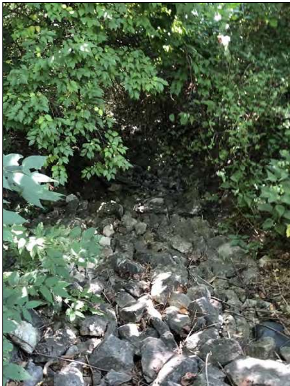
Picture 43—RSD1 riprap from open area; northeast view; 1 SEP 2021.
