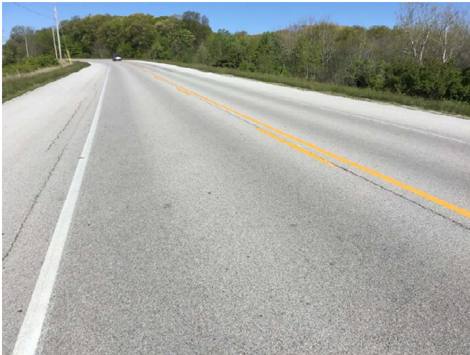
PHOTO 2 Condition Description Road alignment looking West
