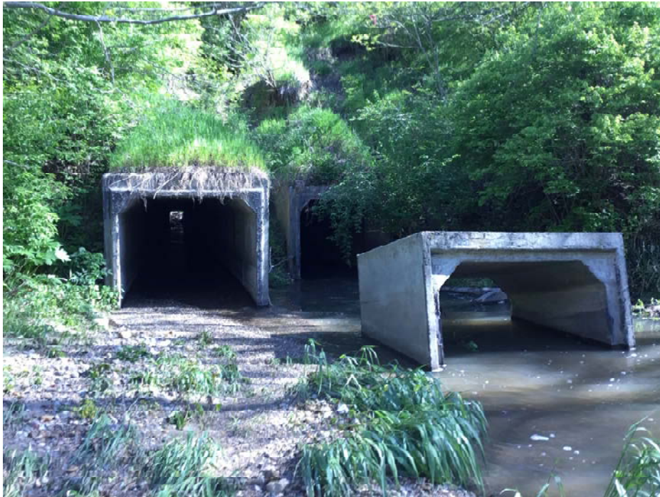
PHOTO 4 Elevation, Condition Description Profile looking North
