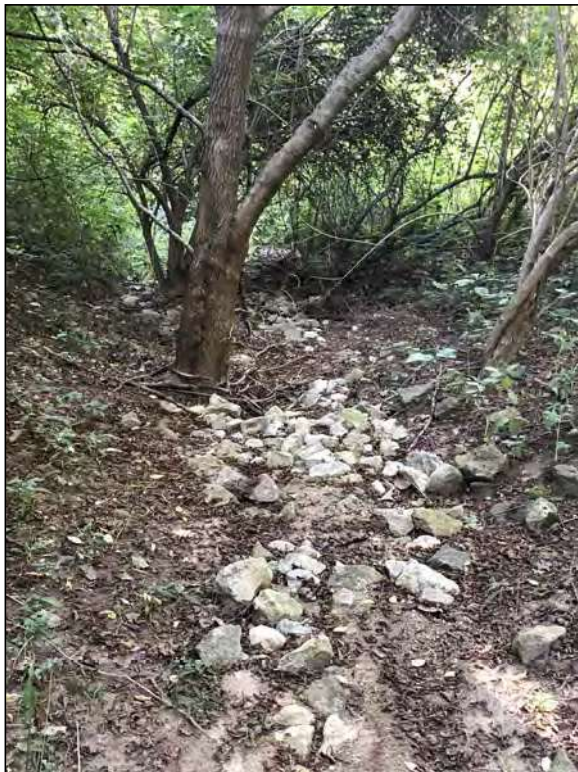
Picture 35—UNT 3 to Goose Creek downstream from end of bed and bank structure—note riprap; east view; 1 SEP 2021.
