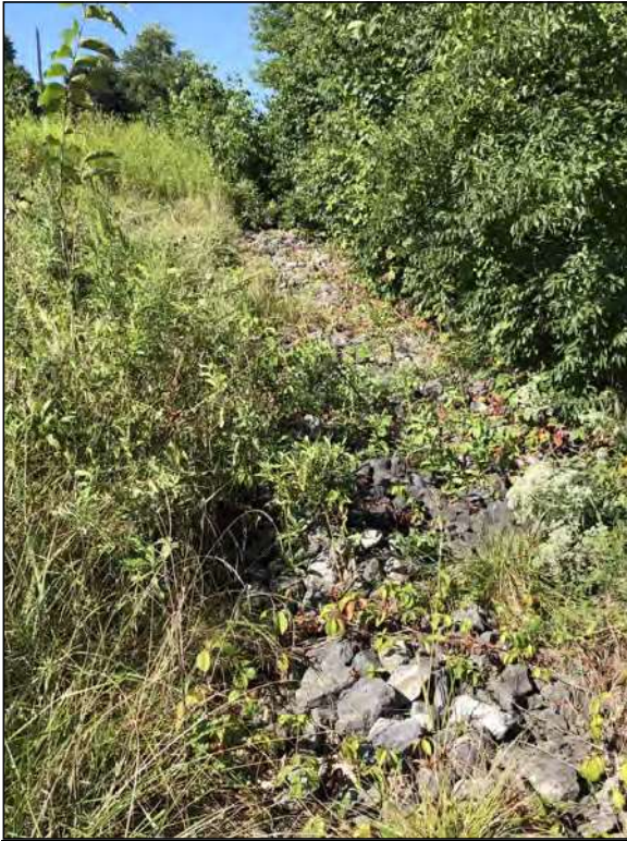
Picture 45—RSD1 open area; southwest view; 1 SEP 2021.
