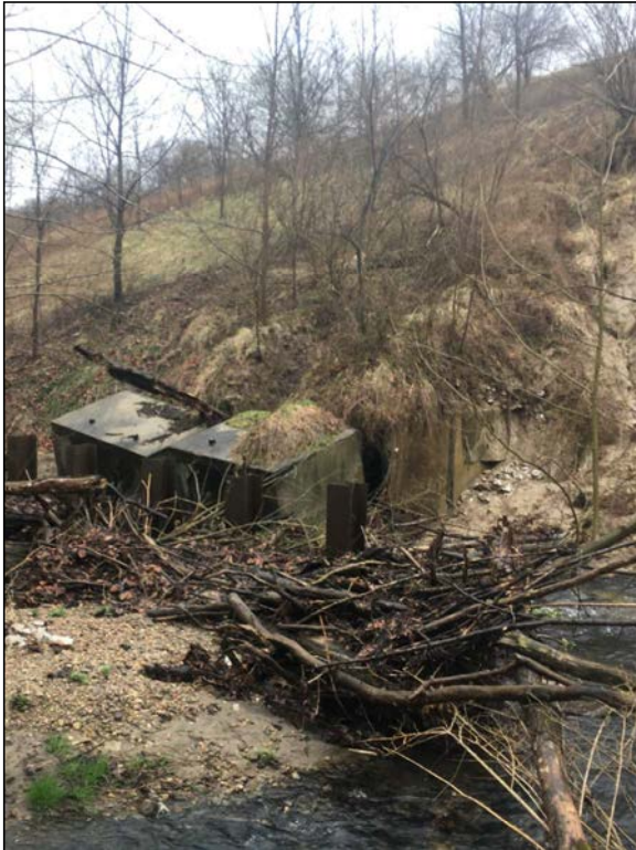
Picture 1—DES 1900333 structure inlet; southeast view; 04 APR 2022.
