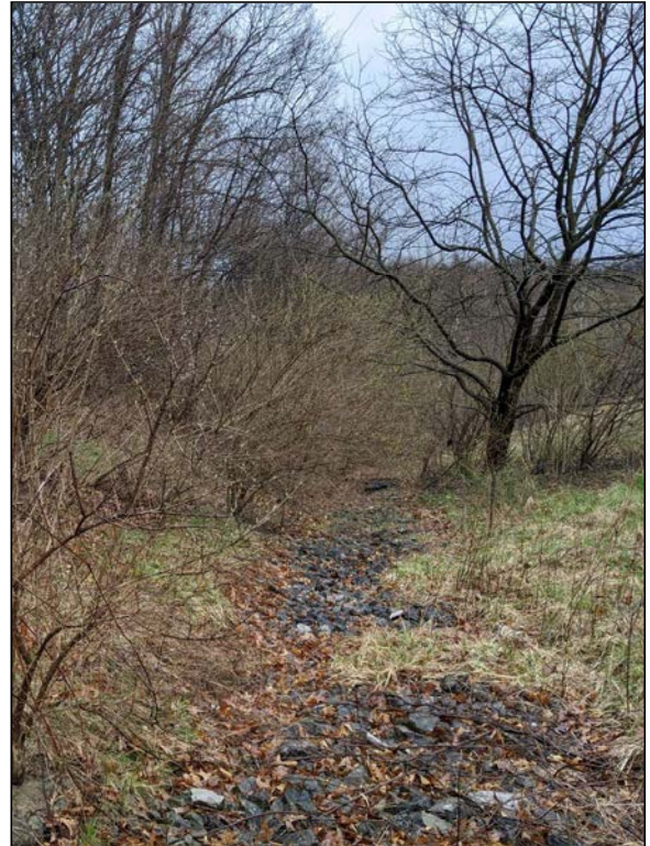
Picture 2—Riprap-lined roadside ditch; northeast view; 04 APR 2022.
