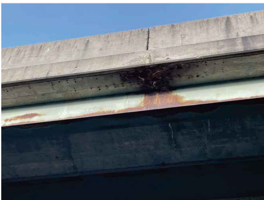
East deck coping and beam 7 condition
