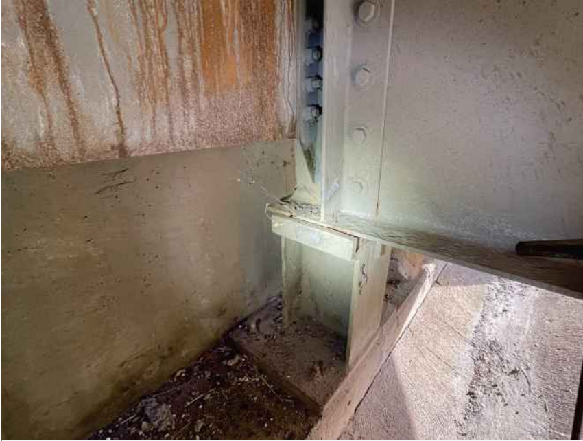
Bent 4 beam 6 and bearing fix condition
