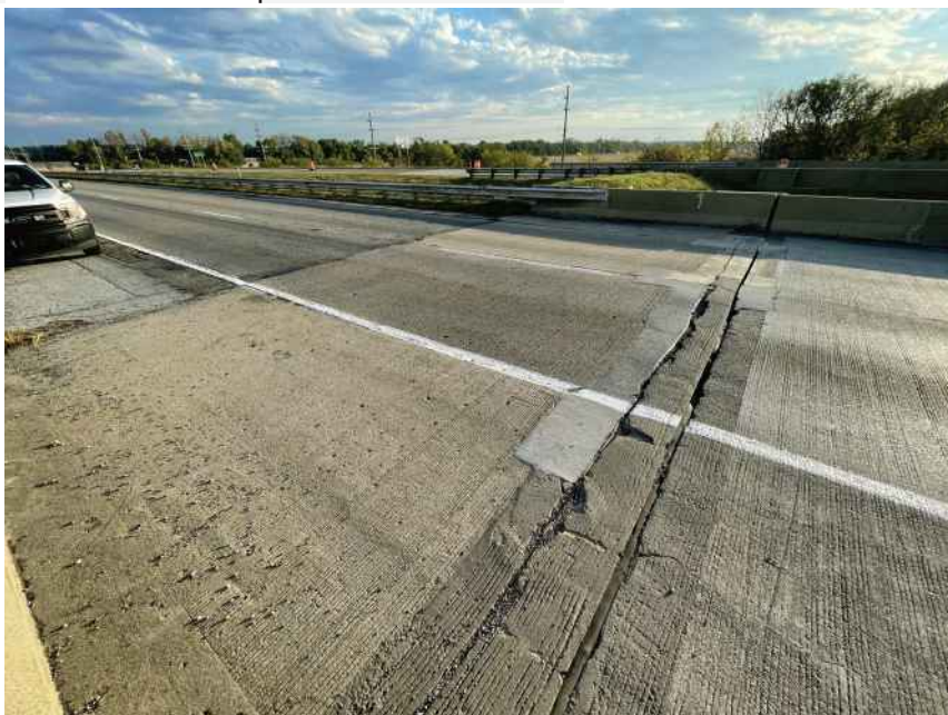
North approach slab and joint condition
