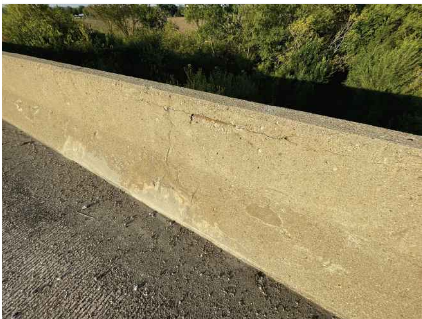
West bridge rail condition at top of rail
