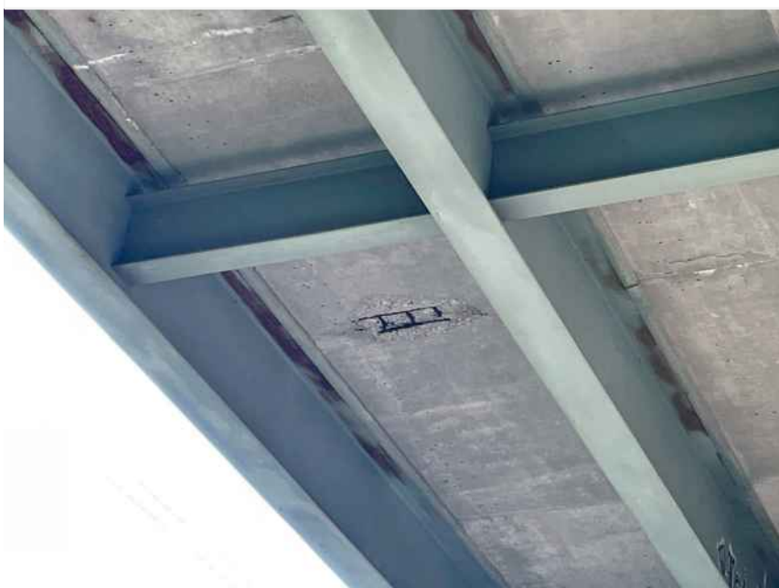
Span C underside spalled between beams 1 and 2
