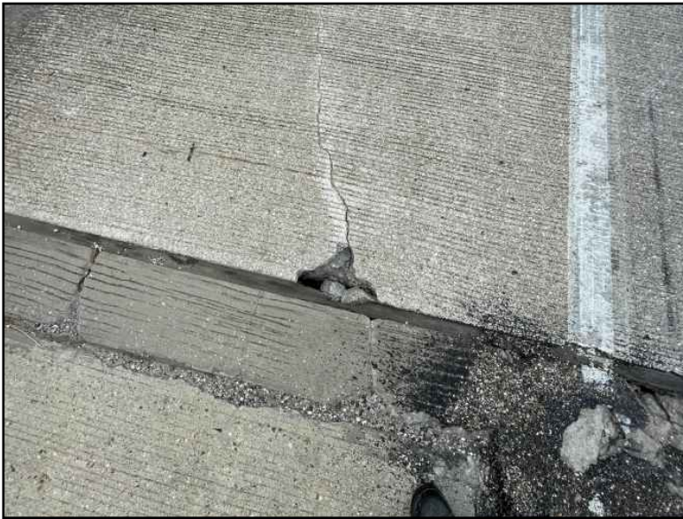
Wearing surface spalled at the north joint * PHOTO
