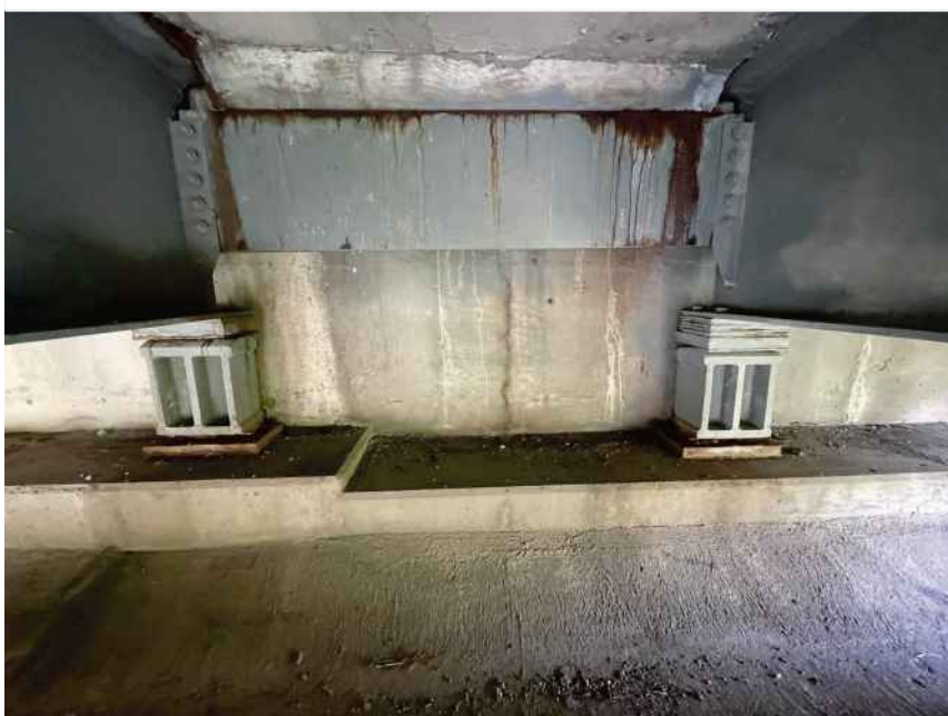
Bent 1 has vertical cracking
