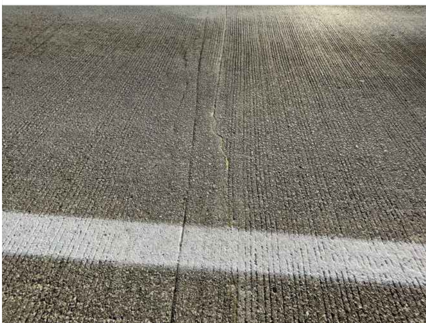
Wearing surface has hairline to wide cracks some have been sealed
