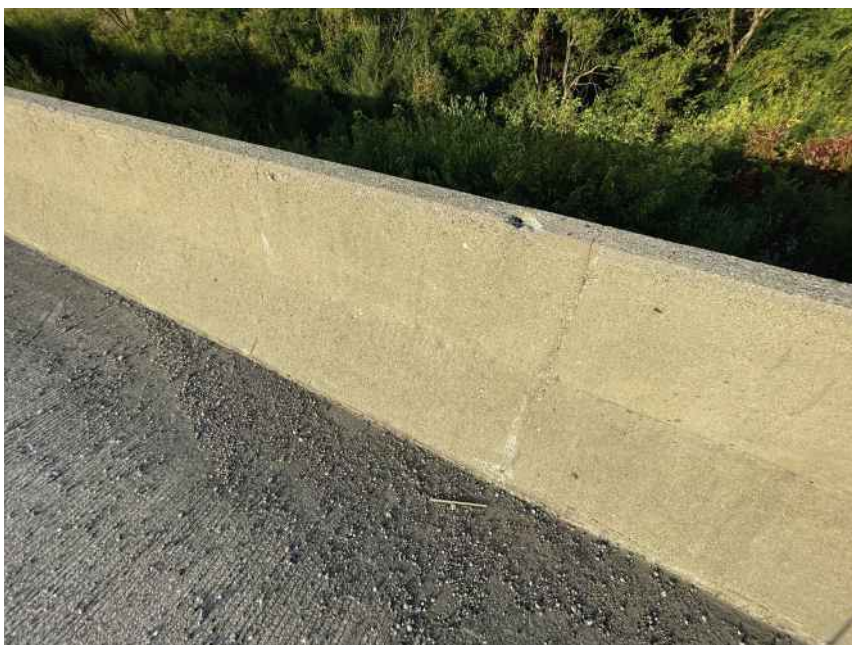
Typical cracking in bridge rail
