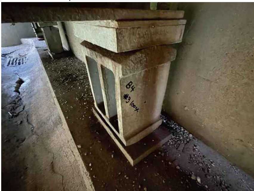
Bent 4 bearing 3 is loose
