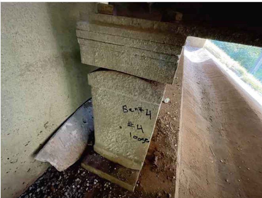
Bent 4 bearing 4 loose
