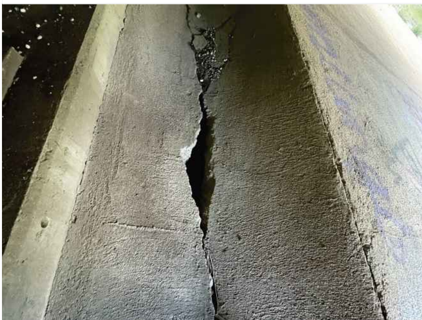
North concrete drain trough spalled
