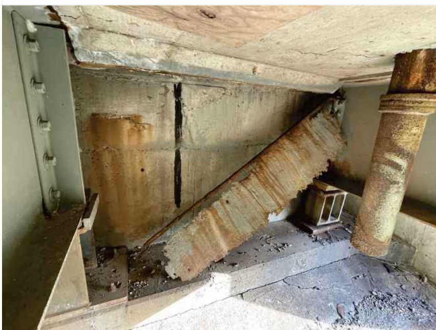
Bent 4 diaphragm between beams 6 and 7 rotted off
