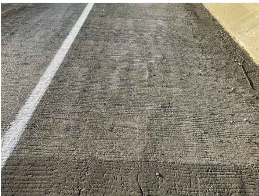
Wearing surface has hairline to wide cracking
