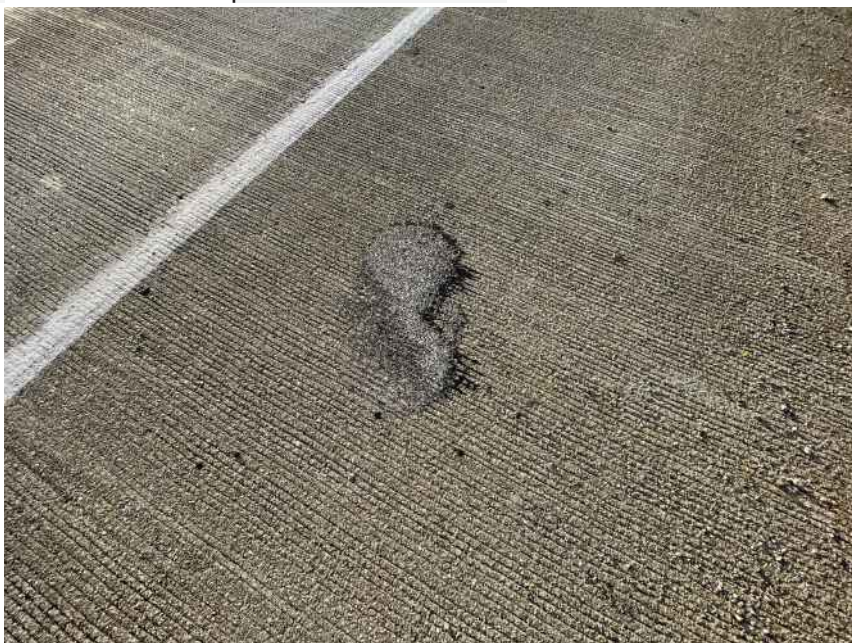
Wearing surface has a asphalt patch on the west shoulder
