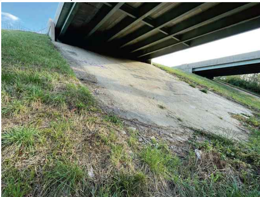
North slope wall condition has cracking
