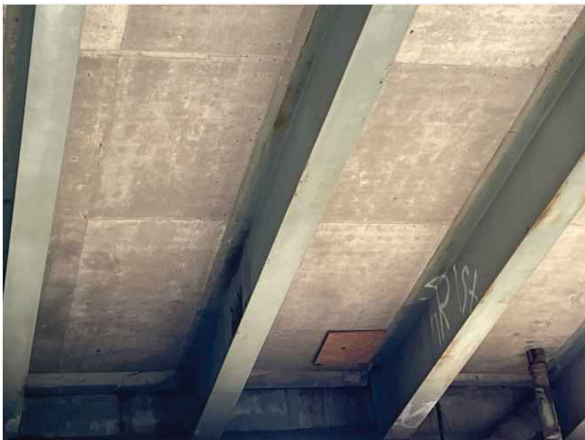
Span C full depth patch near bent 4
