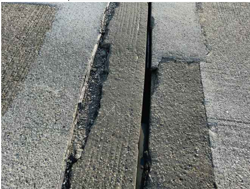
North joint failed and bent 4 is spalled
