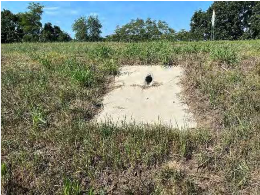
Photo 7. Investigated Area - Looking southwest at an unnumbered median drain pipe located in the southeast quadrant of the investigated area.
