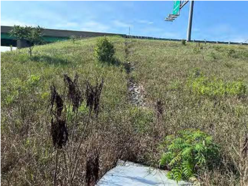
Photo 37. Investigated Area - Looking south towards a riprap lined drainage turnout (RDT 5).
