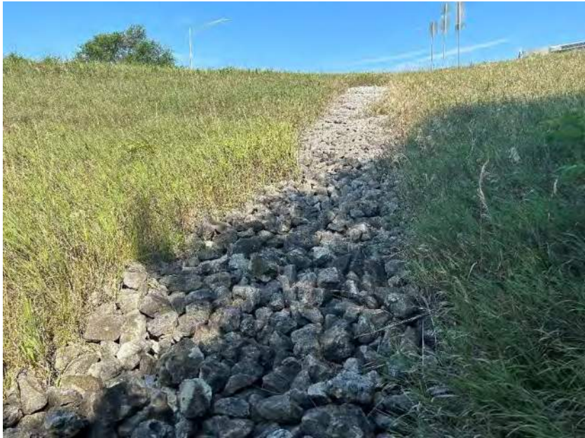
Photo 10. Investigated Area - Looking northwest at a riprap lined drainage turnout depicted in Photo 6 (RDT 1).
