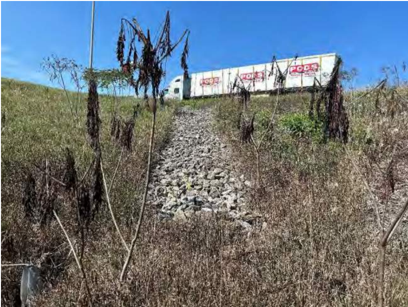
Photo 38. Investigated Area - Looking southwest at a riprap lined drainage turnout located in the northeast quadrant of the southbound ramp junction (RDT 6).
