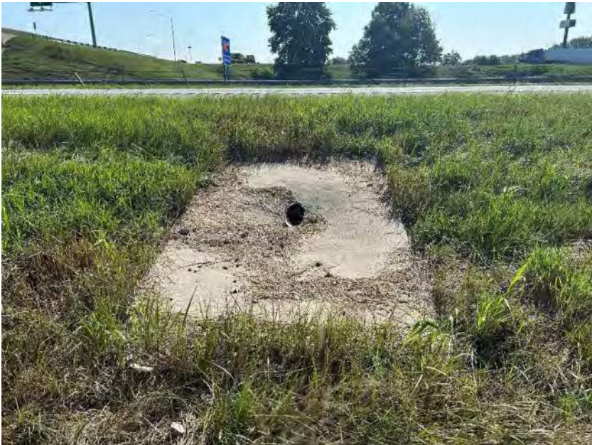
Photo 11. Investigated Area - Looking east at an unnumbered median drain pipe located on the west side of the southbound travel lane of I-65.
