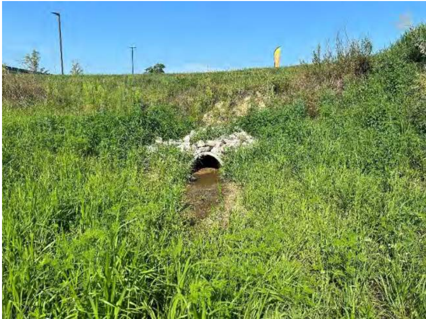
Photo 2. Investigated Area - Looking west at an unnumbered culvert and roadside ditch (RSD) 1. Drainage is conveyed east along SR 10 and south along I-65 via this roadside ditch.
