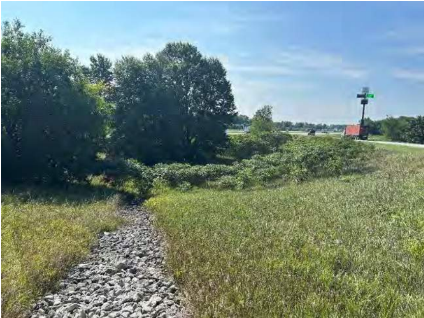
Photo 9. Investigated Area - Looking southeast towards a riprap lined drainage turnout (RDT 1).
