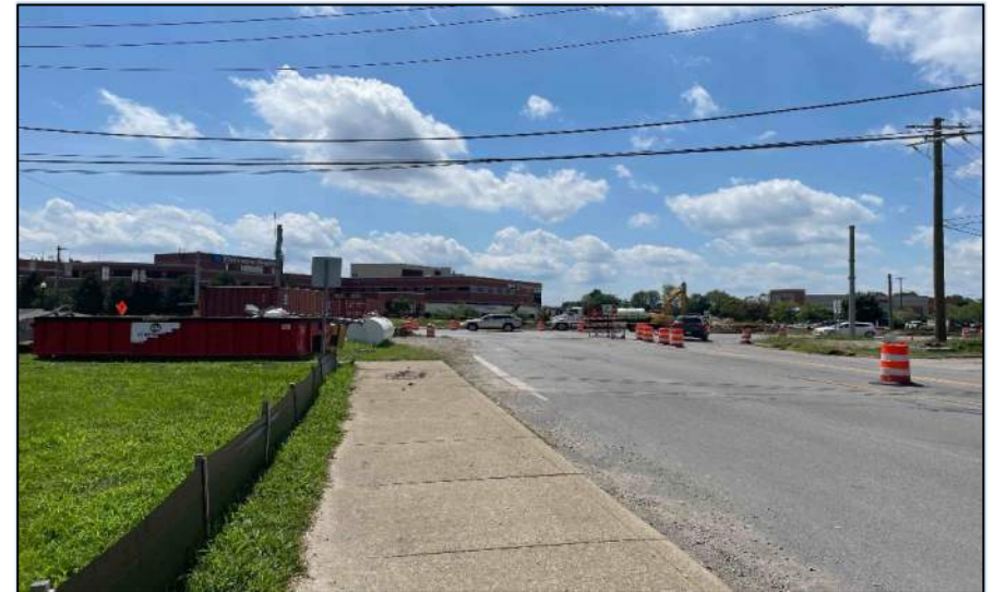
Photo 36: On the east side of SR 38 facing south, just north of SR 32/Westfield Road.
