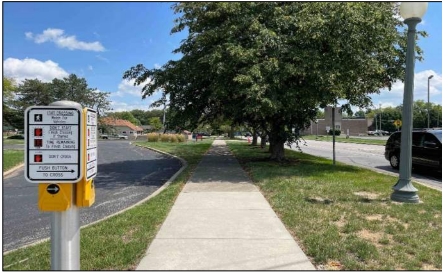
Photo 21: At the northeast corner of the SR 38 and Logan Street intersection looking east.
