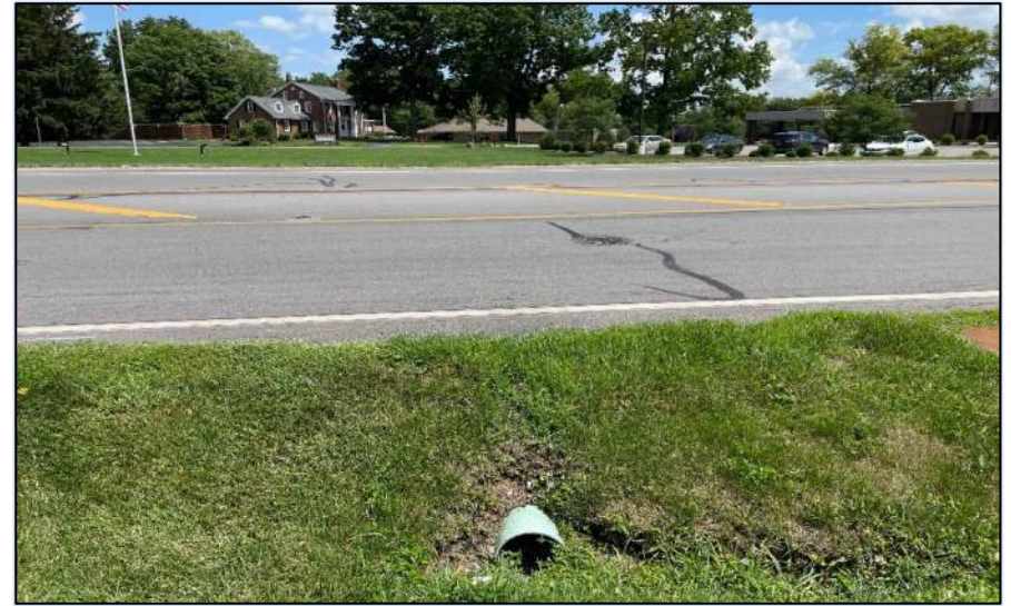
Photo 18: West of SR 38 looking northeast toward a drainage pipe that runs beneath the road.
