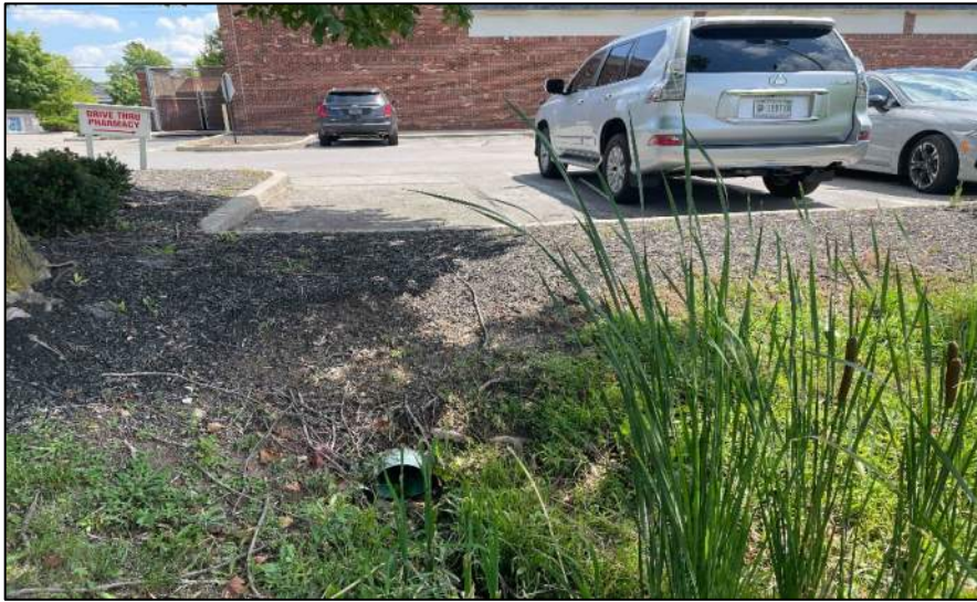
Photo 33: Facing east toward a drainage pipe draining toward Wetland A.
