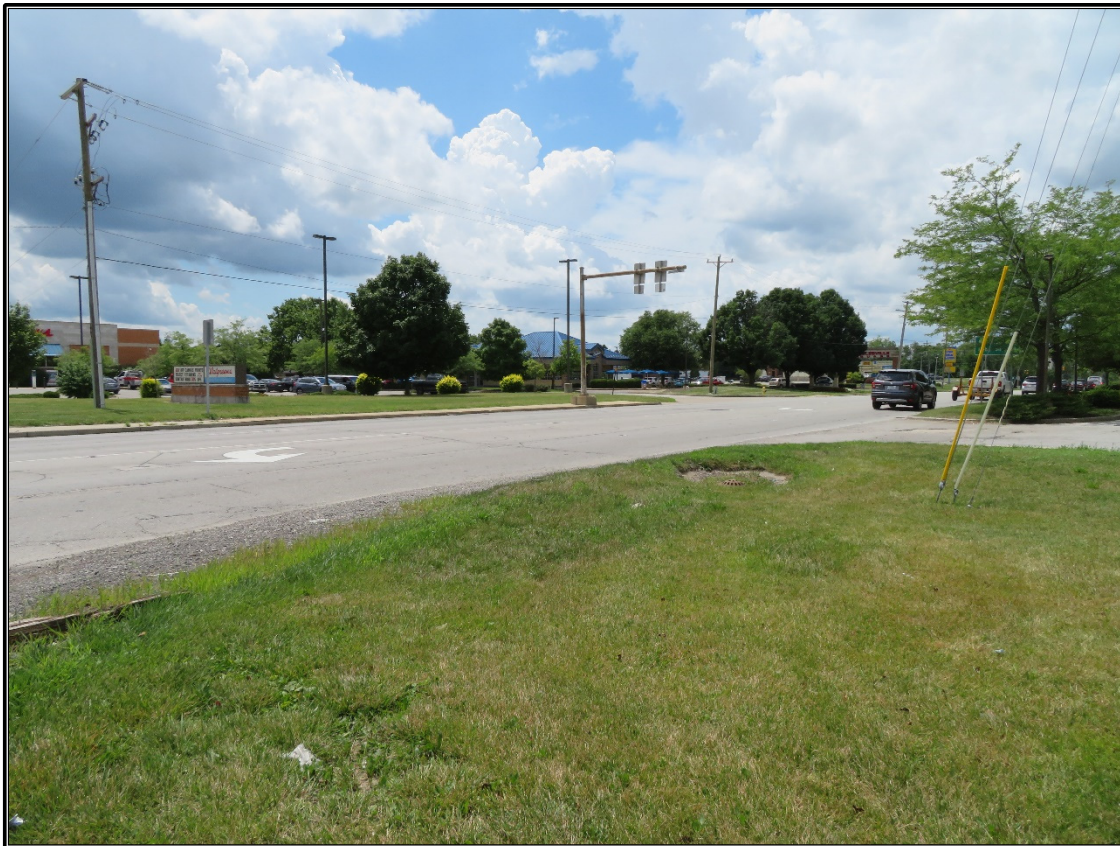
Figure 7. View of modern, commercial landscape, constructed during the late twentieth and early twenty-first centuries, facing southeast.
