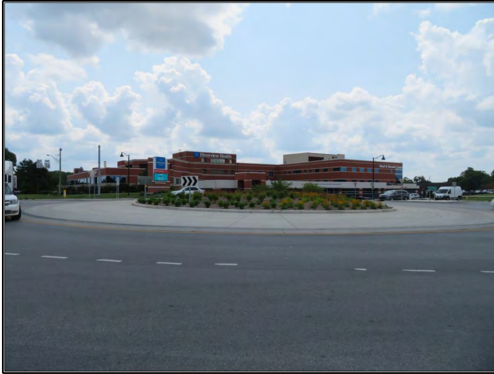
Figure 5. Overview of project area at the Sheridan Road/SR 38 and SR 32 Intersection, facing southeast.
