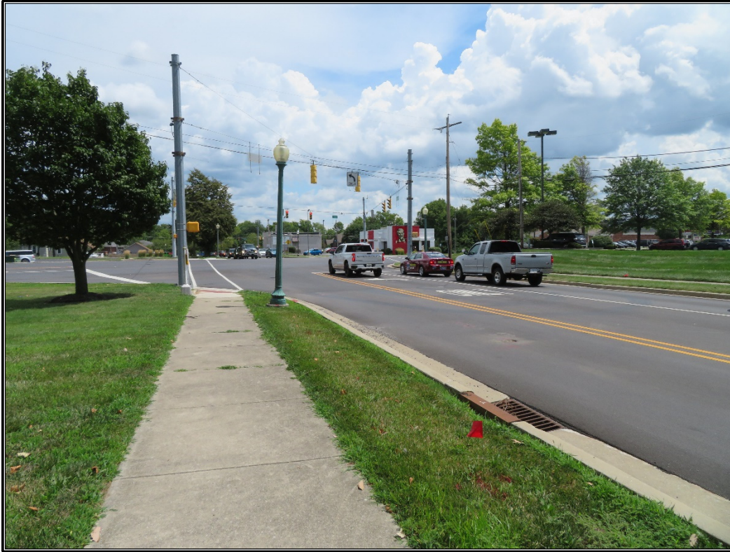
Figure 3. Overview of project area at SR 38 and Logan Street intersection (site of new roundabout), facing southeast.
