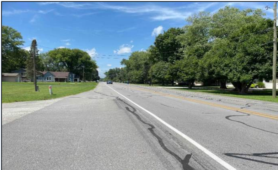
Photo 3: On the southbound side of SR 38 looking northwest, approximately 0.07 mile north of Monterey Drive.
