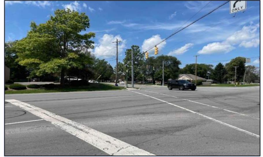
Photo 26: At the southeast corner of the SR 38 and Logan Street intersection looking west.
