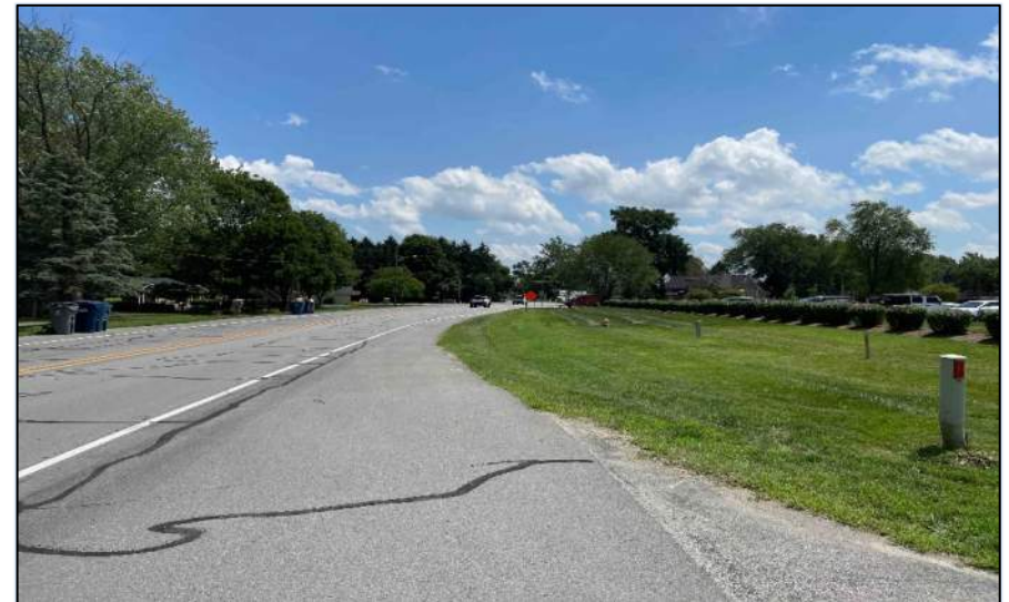
Photo 4: On the southbound side of SR 38 looking southeast, approximately 0.07 mile north of Monterey Drive.
