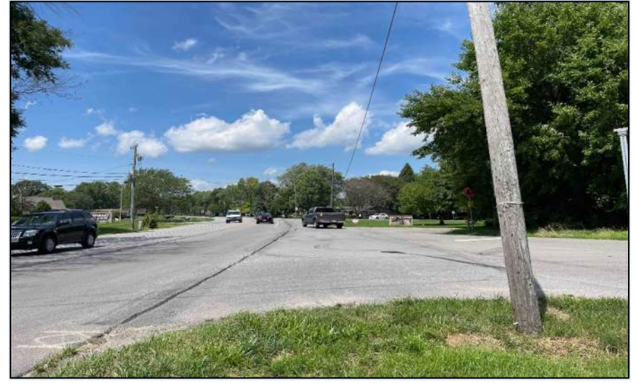
Photo 14: On the northbound side of SR 38 looking northwest, at the intersection of Lafayette Road.
