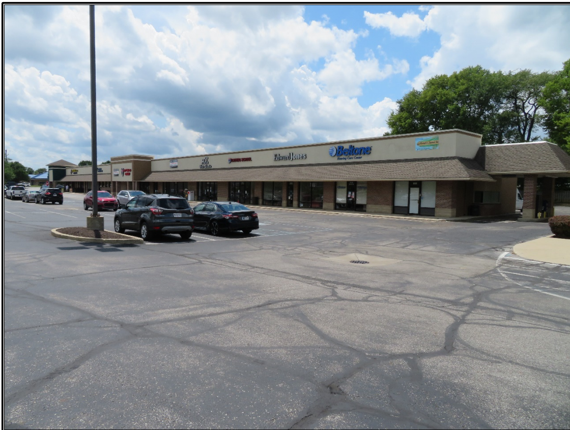
Figure 6. View of commercial building constructed during the 1970s, façade (east) elevation and north elevation, facing southwest.
