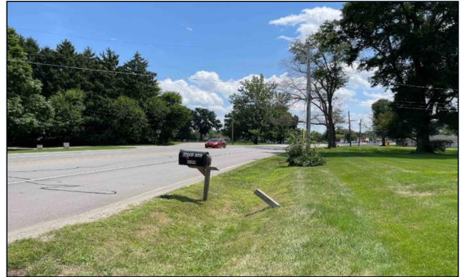
Photo 8: On the southbound side of SR 38 looking southeast, at the intersection of Monterey Drive.
