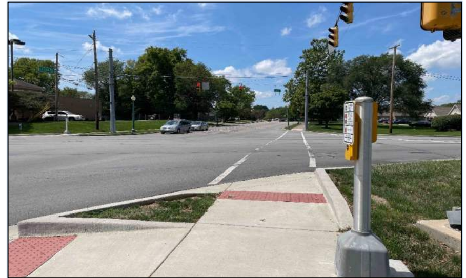
Photo 20: At the northeast corner of the SR 38 and Logan Street intersection looking west.
