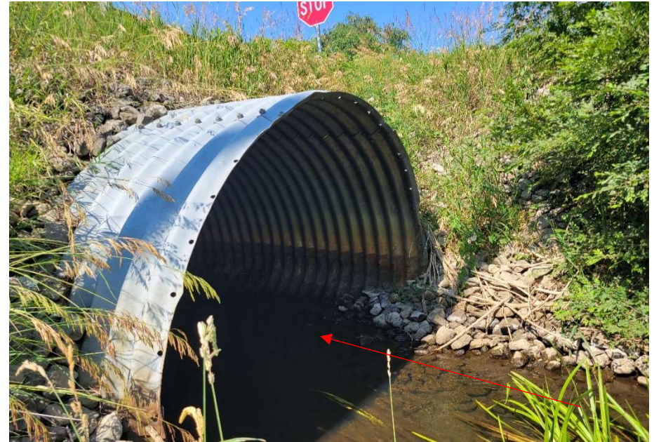
Photo 24. Facing southwest toward the project structure (inlet). Riprap is visible.
