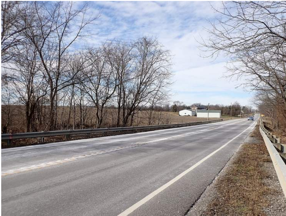
Photograph 2. View looking northwest from near the east end of the project area.
