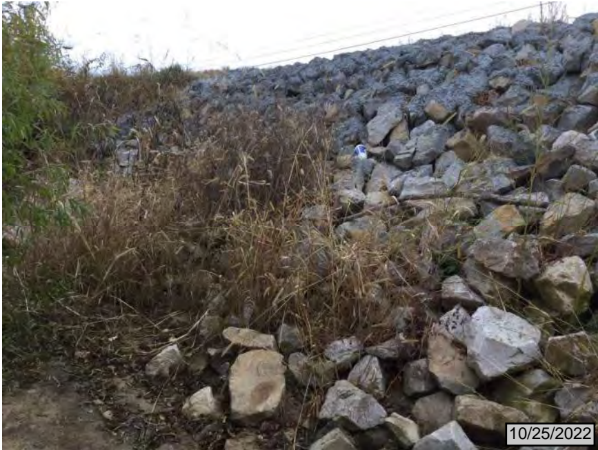
13. From Lost Creek, facing southeast toward armored fill slope and SR 64
