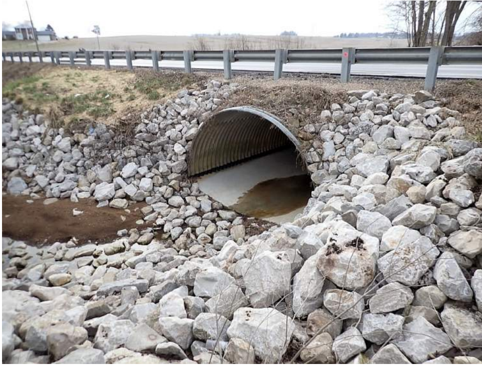
Photograph 5. Non-historic culvert in project area, looking southeast.
