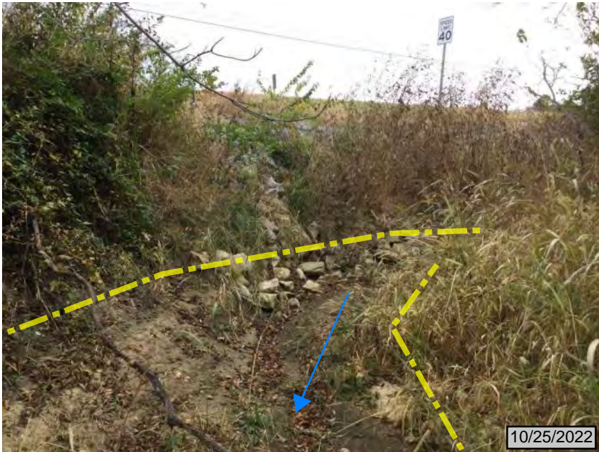
19. Facing south, upstream, toward bend of Lost Creek on north side of SR 64 Des No. 2100263
