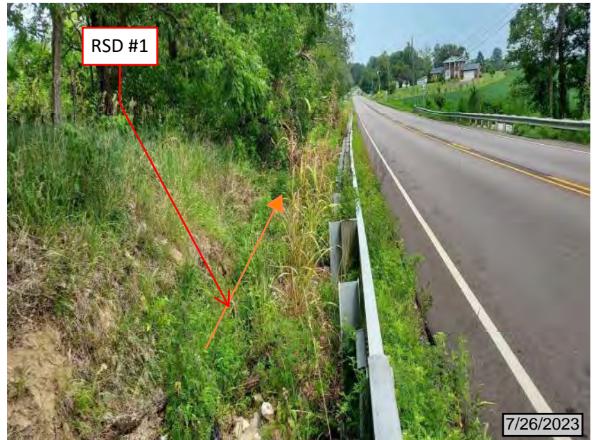
46. North side of SR 64, looking east along RSD #1
