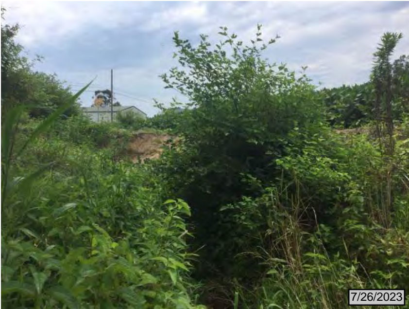
45. North of SR 64, looking southwest from UNT 2 to Lost Creek. Note severe erosion of bank
