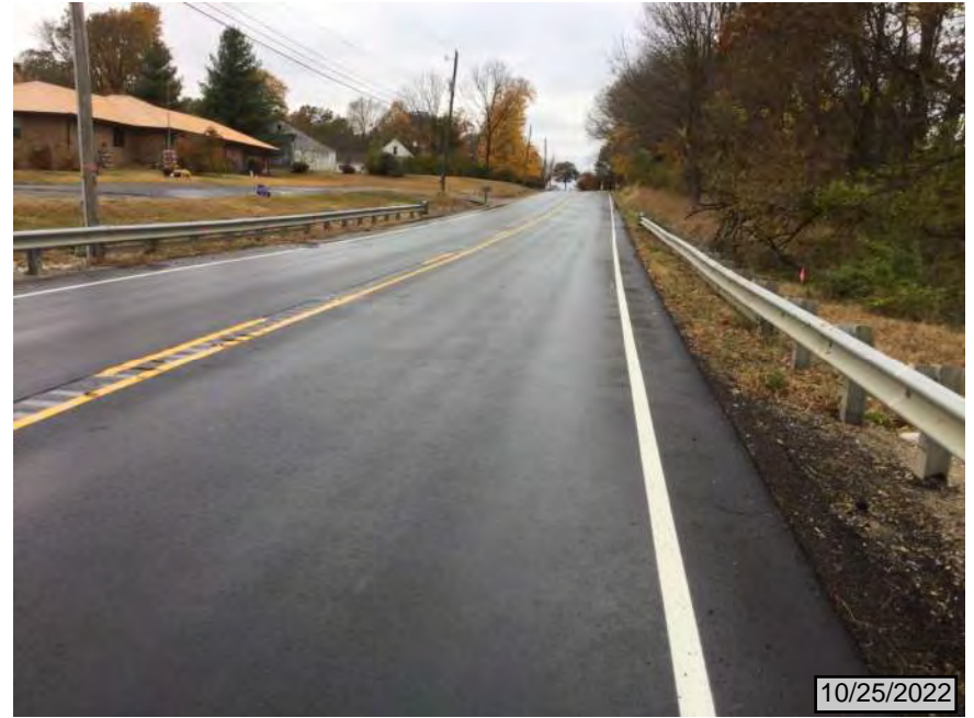
2. North side of SR 64, looking southwest along SR 64
