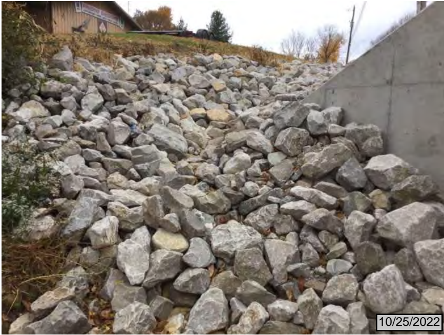
5. On south side of SR 64, facing west toward riprap armoring at headwall
