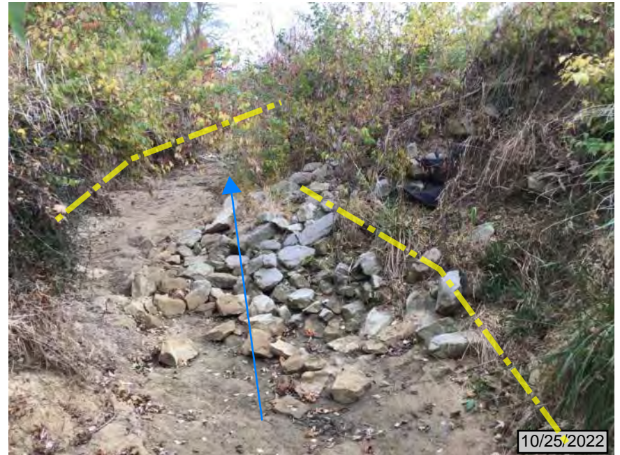
16. Looking east, downstream, along Lost Creek on north side of SR 64
