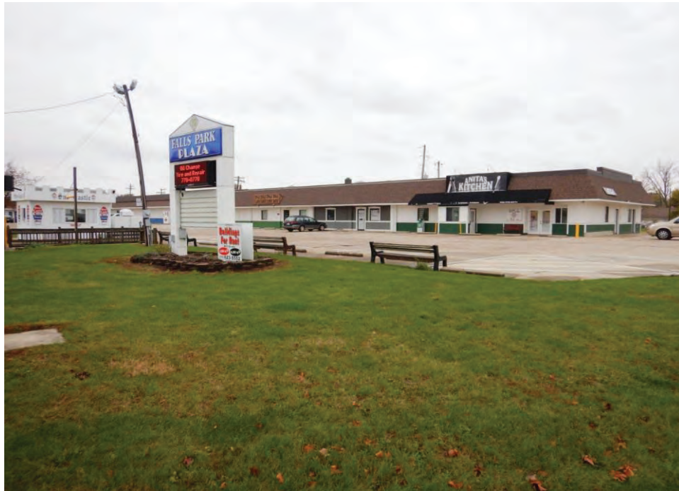
Photograph 7. Overview of commercial property at the northwest corner of Water Street and SR 9, looking northwest.
