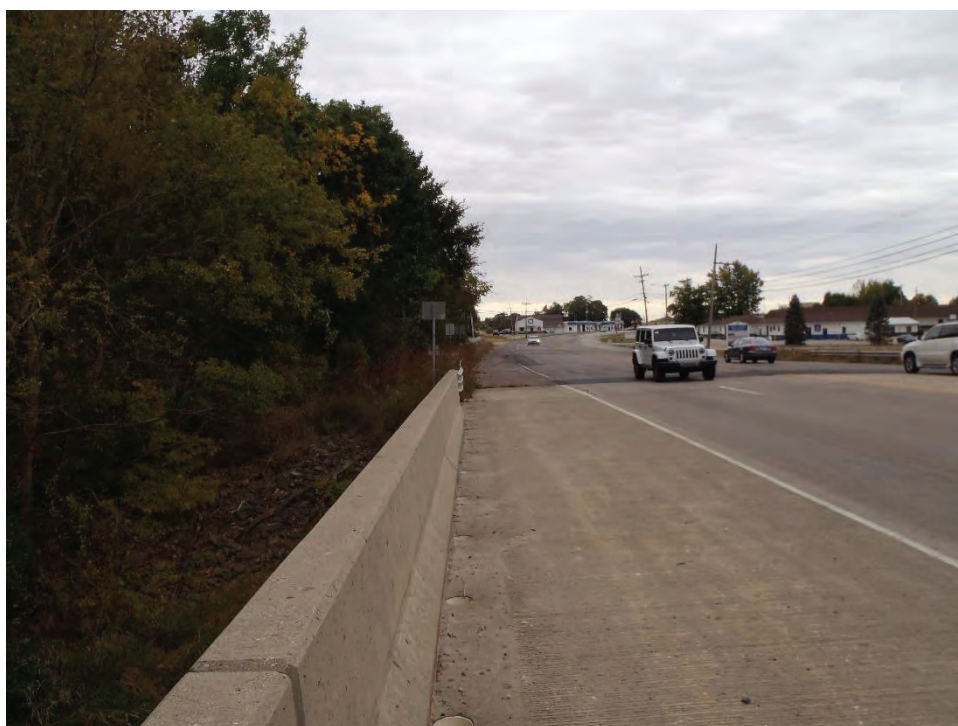
Photograph 8. View of SR 9 from the bridge over Fall Creek, facing south.
