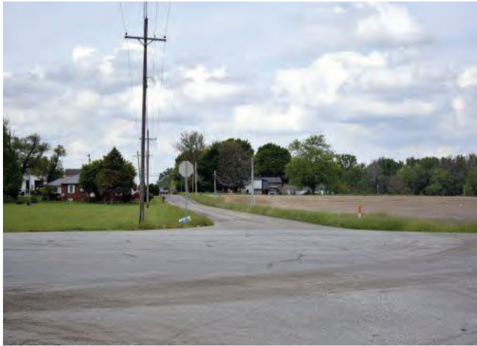
Photograph 11. Street overview of S CR 300 W, looking north-northeast from the US 36 and S CR 300 W intersection.
