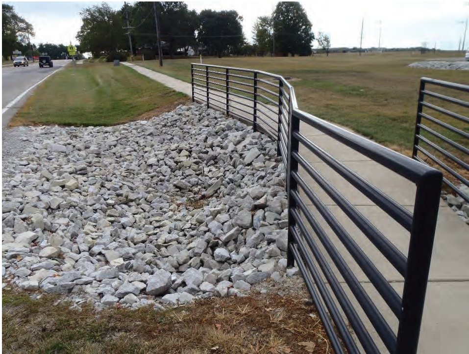
Photograph 6. View of the pedestrian bridge on the eastern project boundary, south of SR 38, facing southeast.
