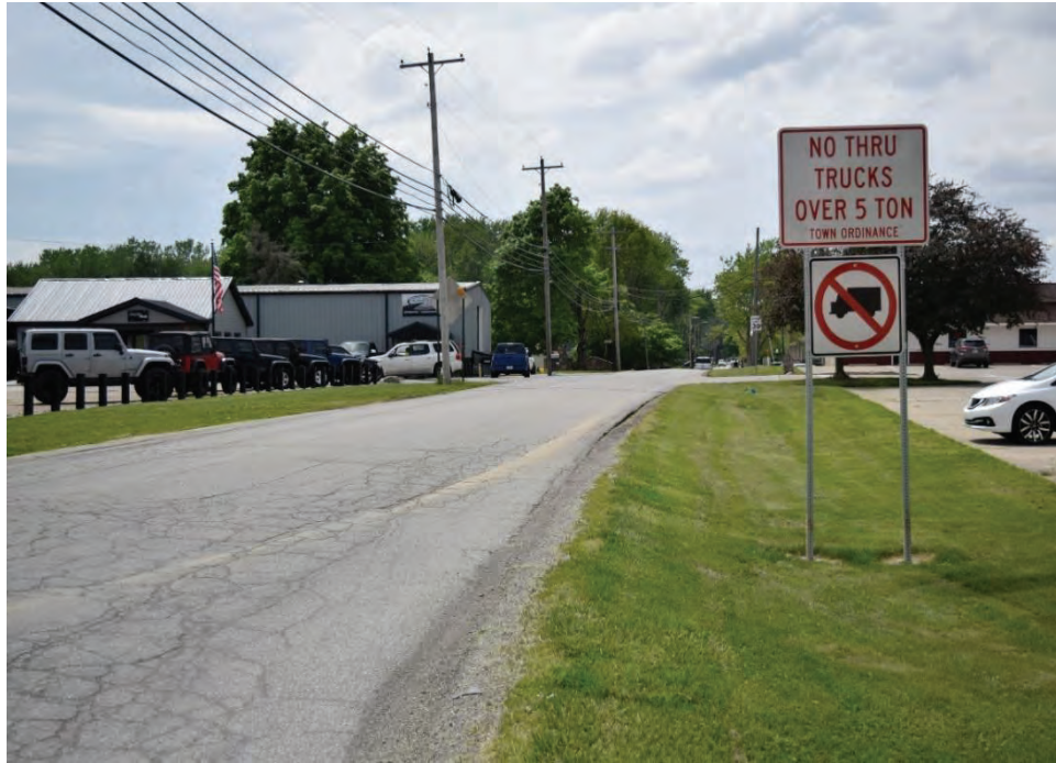
Photograph 9. Street overview of East Water Street, looking west from SR 9.
