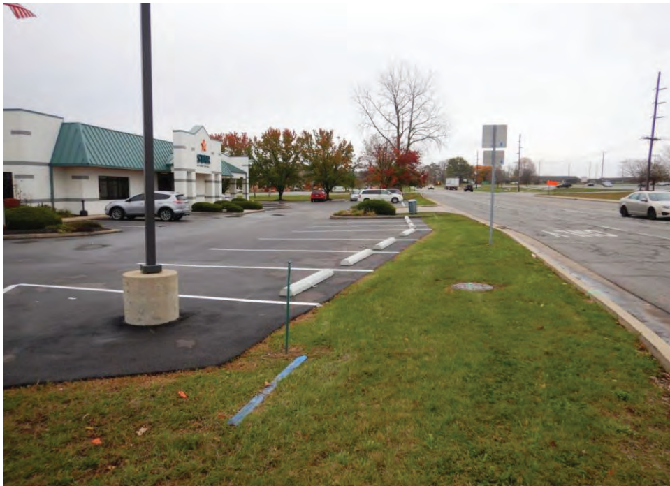
Photograph 14. Overview of commercial lot in the northeast quadrant of the SR 9 and SR 38 intersection, looking east-southeast.
