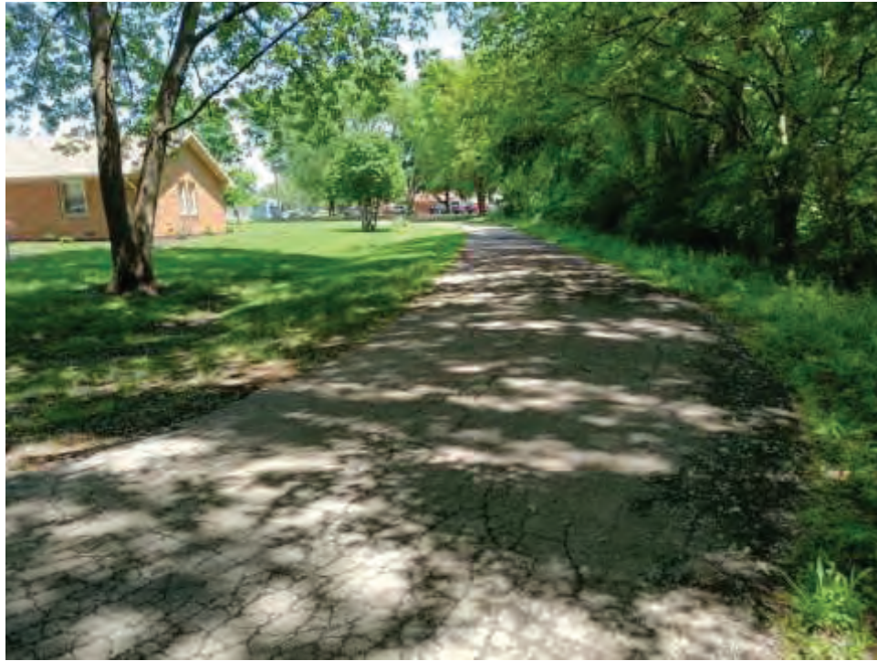
Photo 11. View looking east along Hayden Way.
