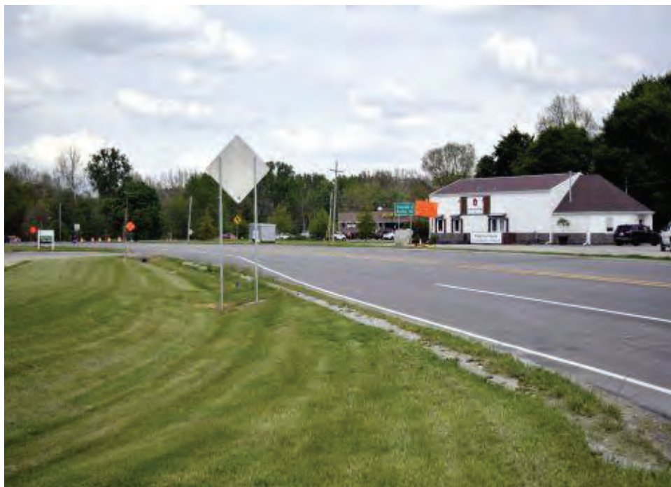
Photograph 8. Street overview of SR 9, looking north-northeast from the SR 9 and East Water Street intersection.
