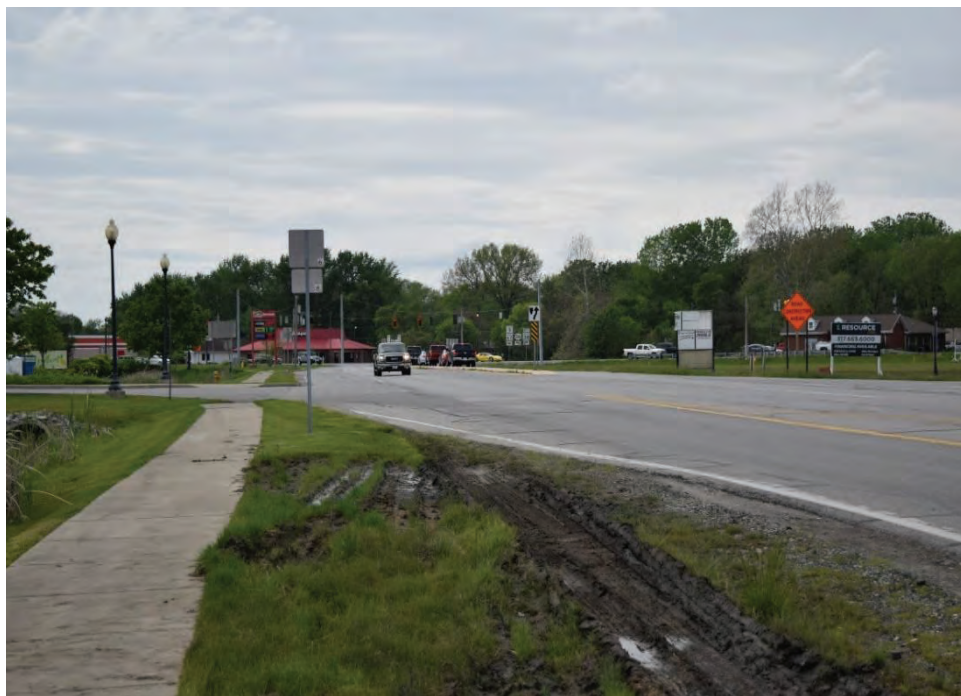
Photograph 12. Street overview of US 36, looking west from the US 36 and S CR 300 W intersection.
