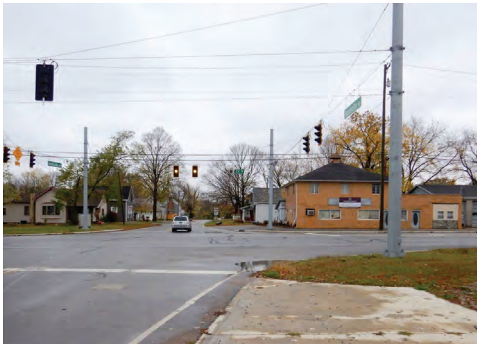
Photograph 4. Street overview of Huntsville Road/CR 500 S/CR 500 S, looking west from the Huntsville Road/CR 500 S/CR 500 S and SR 9 intersection.
