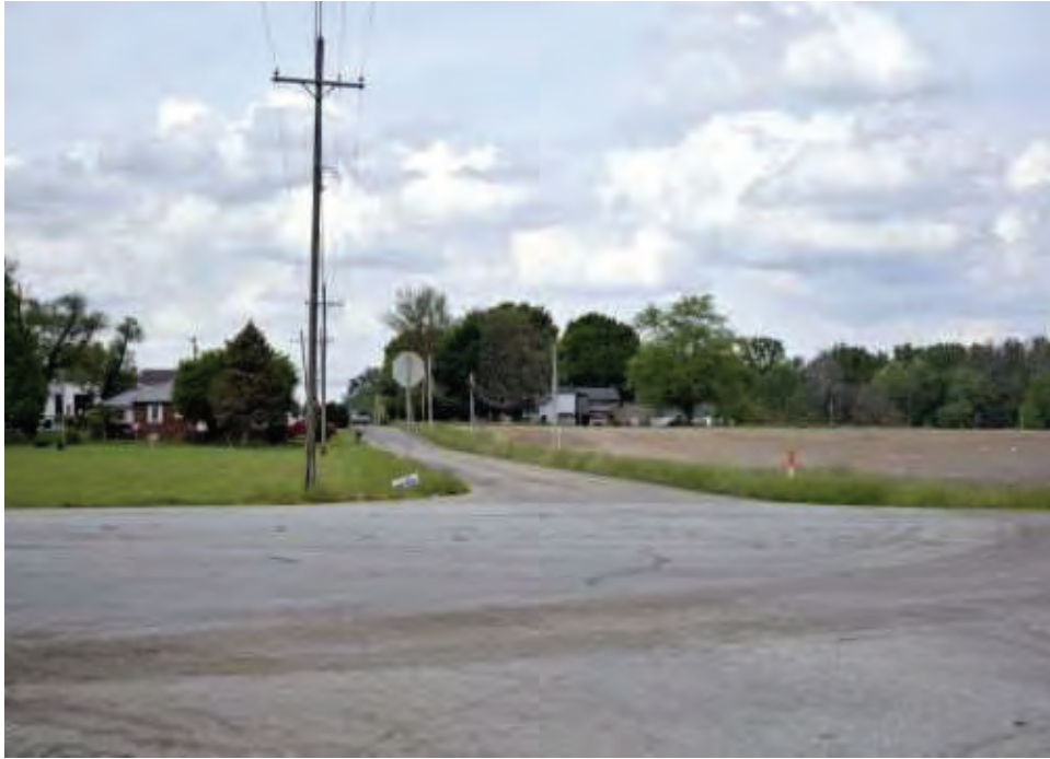
Photograph 3. Street overview of S CR 300 W, looking north-northeast from the US 36 and S CR 300 W intersection.
