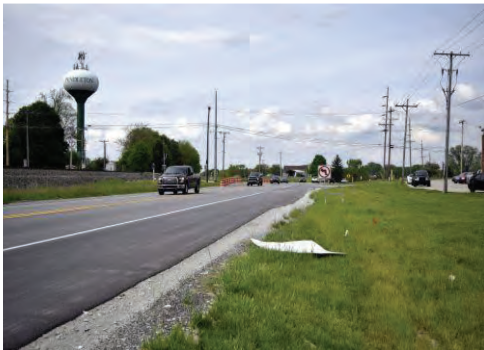
Photograph 18. Overview of SR 67, looking north-northwest from the southern end of the project area.
