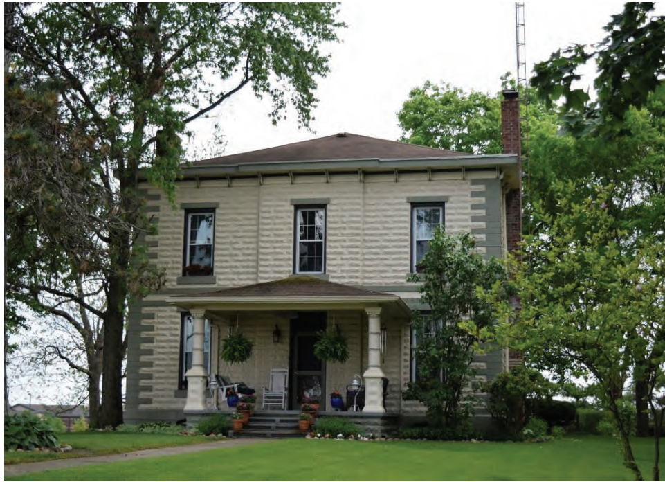
Photograph 1. Overview of house at 3021 SR 38, looking south.
