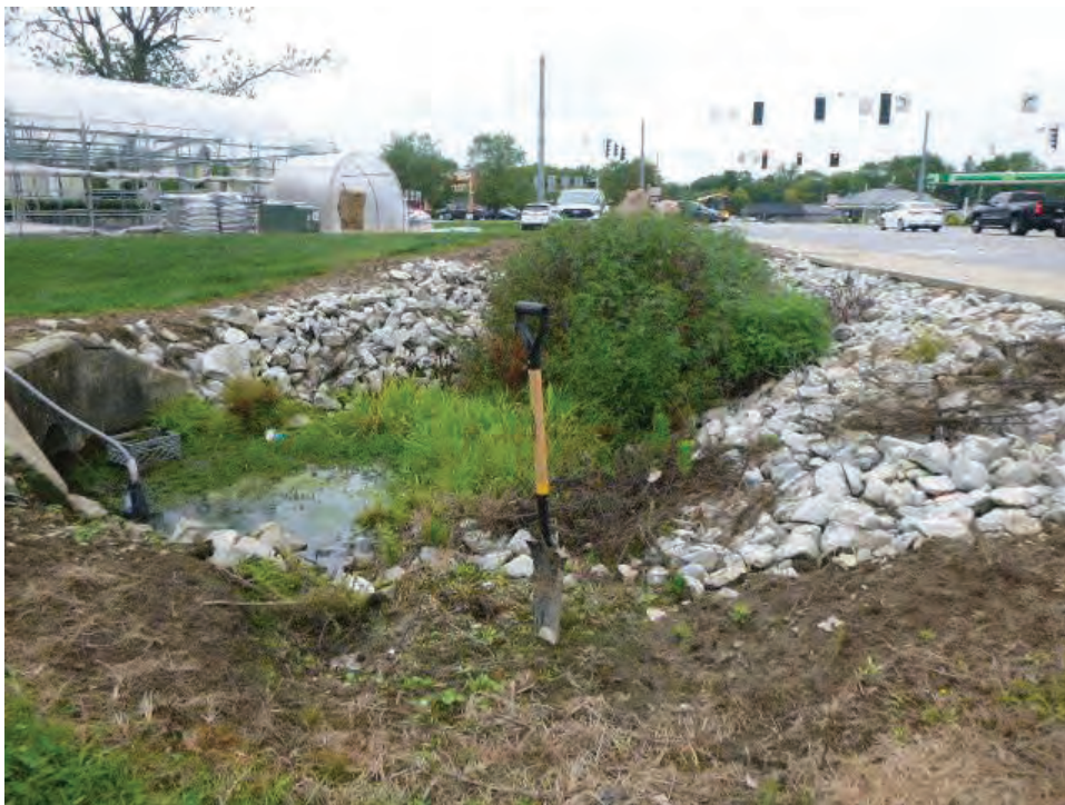
Photograph 24. View of riprap, south of SR 38, facing northwest (taken on September 18, 2022).
