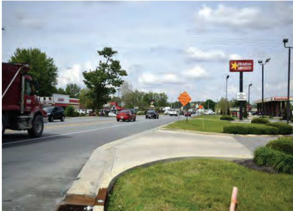
Photograph 15. Street overview of SR 67, looking north from the SR 67 and SR 38 intersection.
