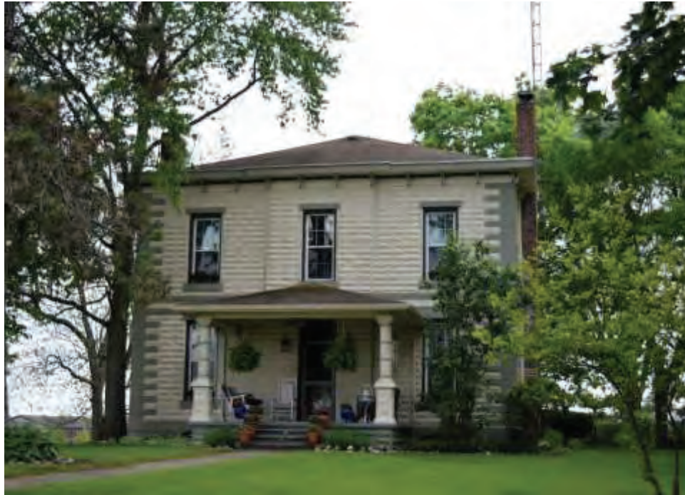
Photograph 1. Overview of house at 3021 SR 38, looking south.
