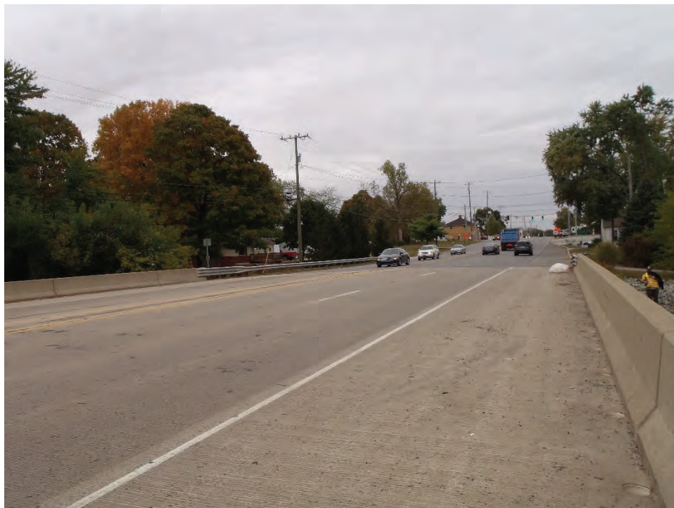
Photograph 7. View of SR 9 on the bridge over Fall Creek, facing north-northwest.
