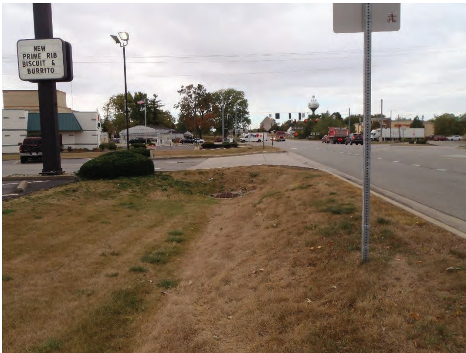
Photograph 20. View of a catch basin along the east project area boundary, east of US 36, facing southwest.
