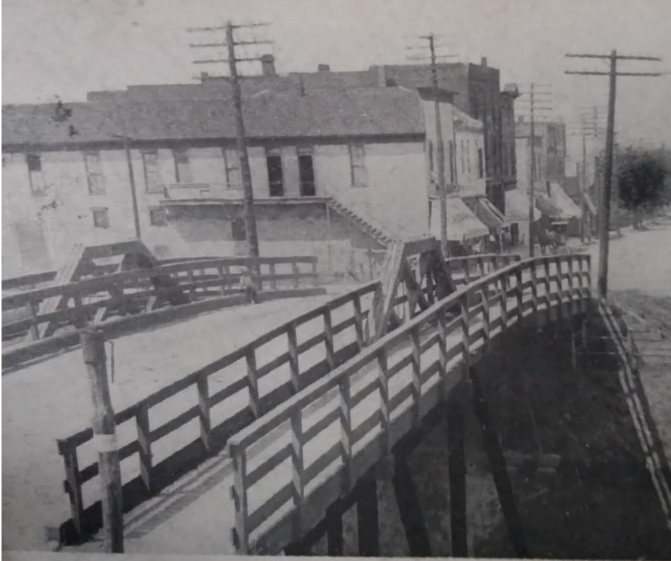
MAIN STREET BRIDGE, UPLAND, IND.
