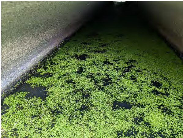
Photo 3: View of standing water in structure.
