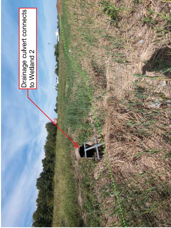
Photo 37. Drainage culvert leading to Wetland 3 facing northwest
