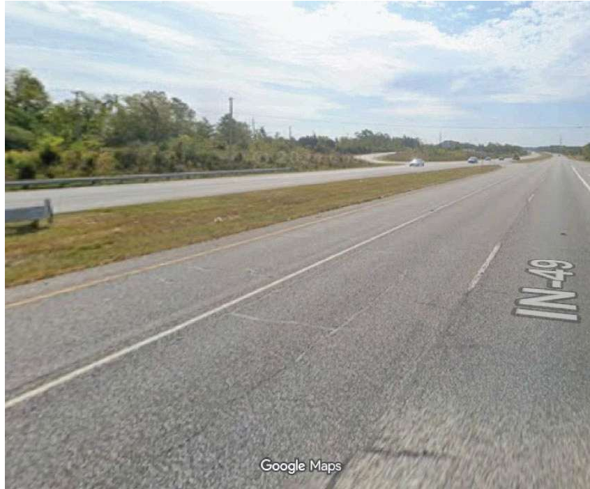
Photograph 9: Looking South Along Southbound Lane at North End of Project Area
