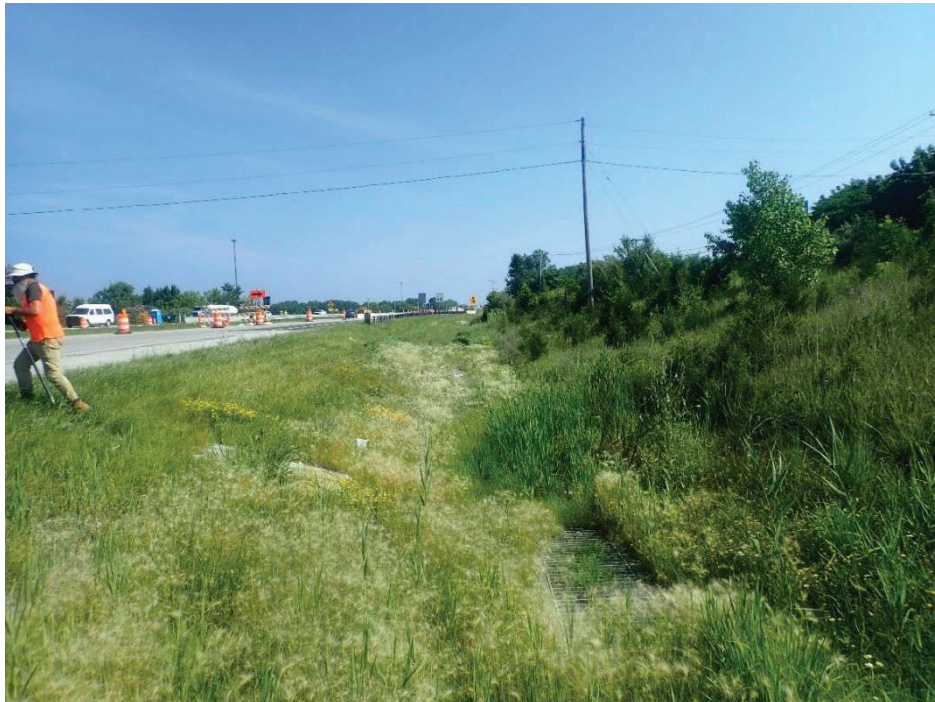
Photograph 22: Looking North Along East Side of S.R. 49 at Proposed Right Turn Acceleration Lane
