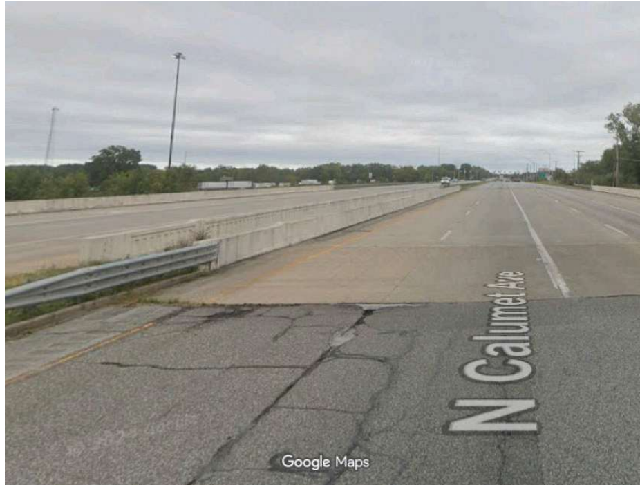
Photograph 13: Looking North Over 80-90 Overpass at North End of Project Area
