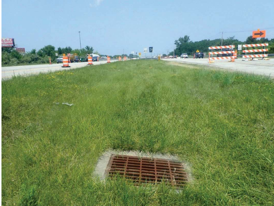
Photograph 21: Looking North at Proposed Structure Nos. 12, 12a, and 12b Site in Median
