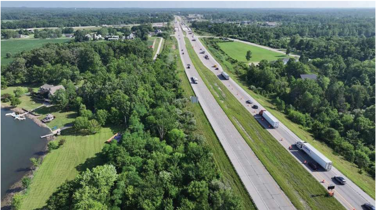
Photograph 2: Aerial View of S.R.49 Looking North from South End of Project Area
