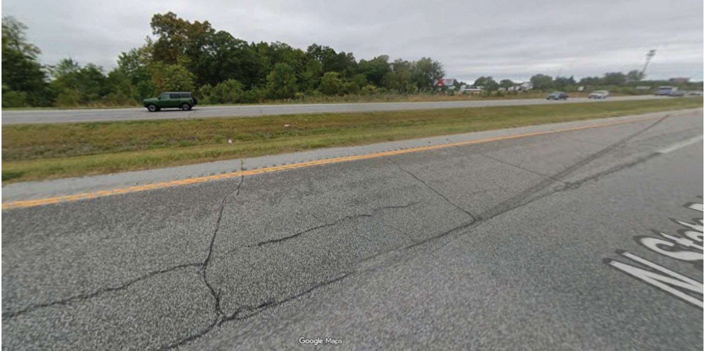
Photograph 17: Looking North Along East Side of Road at Site of Proposed Structure No. 10
