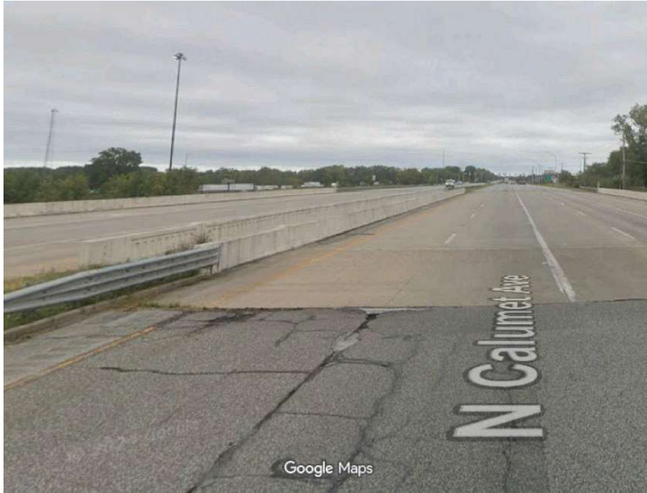
Photograph 13: Looking North Over 80-90 Overpass at North End of Project Area
