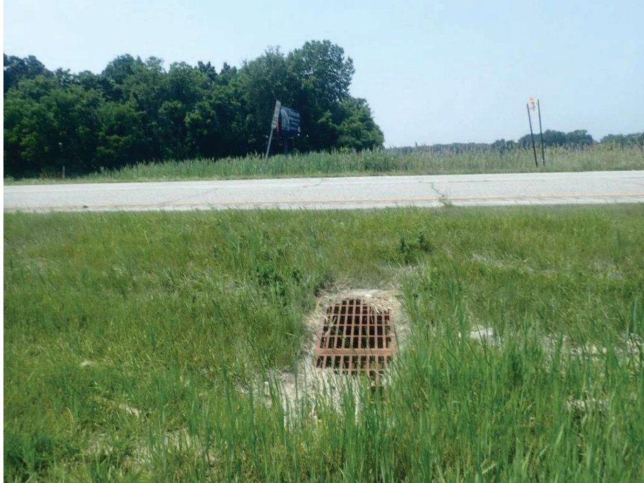
Photograph 19: Looking East From Median Site of Proposed Structure Nos. 11, 11a, and 11b
