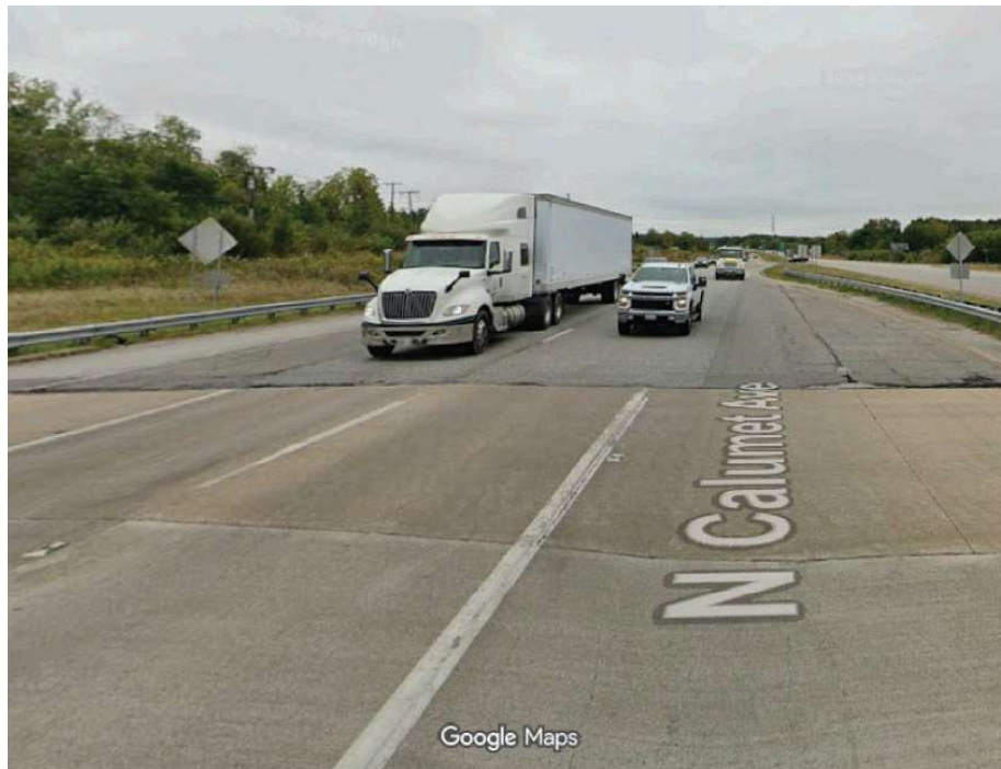
Photograph 10: Looking South from Northbound Lane at North End of Project Area
