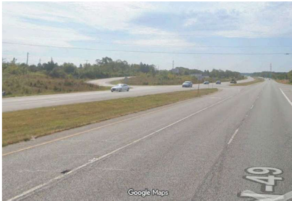
Photograph 8: Looking South at S.R.49 C.R. 950 N/Calumet Avenue Intersection
