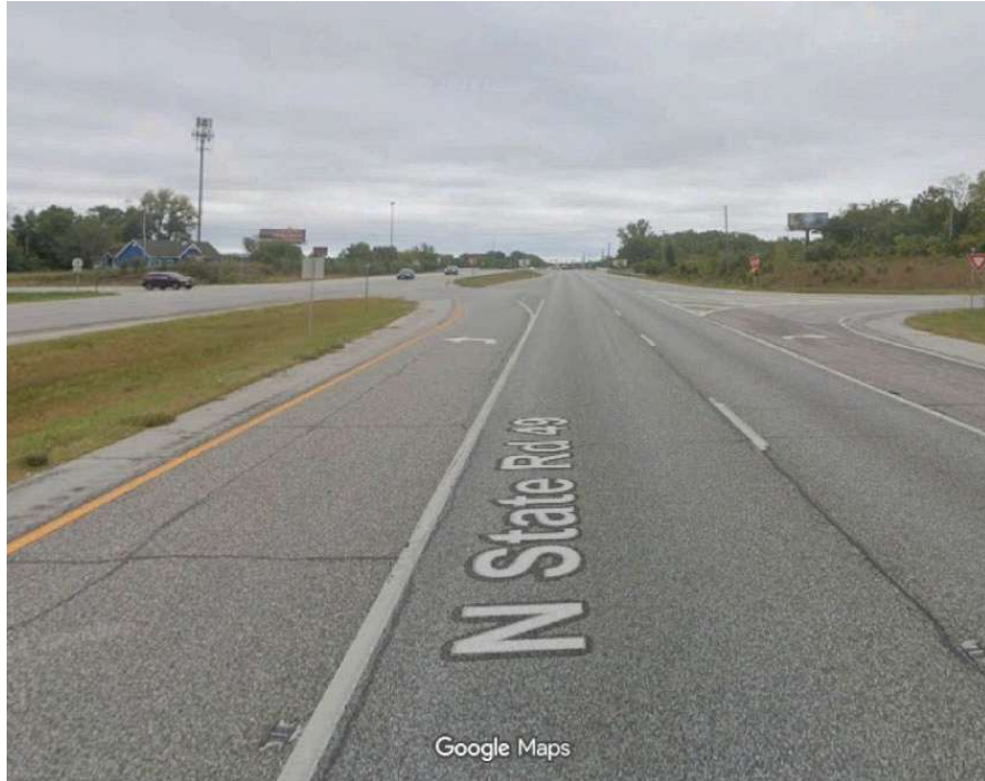
Photograph 5: Looking North at S.R.49 C.R.950 N/Calumet Avenue Intersection
