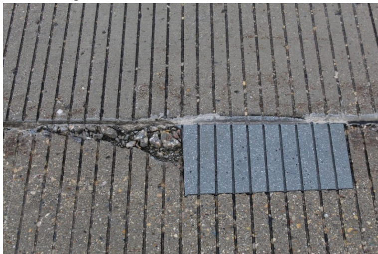
Cracked and delaminated concrete appears next to a small area on Runway 18-36, which had been previously patched.
