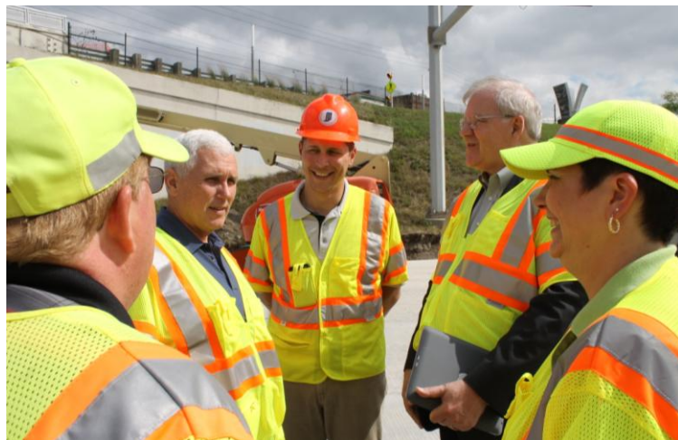
Gov. Mike Pence visited the South Split project on Sept. 30. Joining the governor (second from left) were (left to right) District Construction Director Roland Fegan, Project Manager Trevor Mills, INDOT Commissioner Karl B. Browning, and Greenfield District Deputy Commissioner Brandye Hendrickson.
