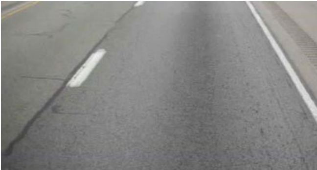
I-64 in 2018 (top photo) reveals only top-level thermal cracks since its 2004 conversion to perpetual pavement; in June 2023 (bottom photo), four years after minor preventative maintenance, the road is in great shape as Kumar Dave stands on it.
