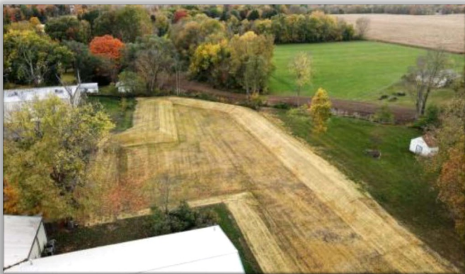
Above: Hammer Street Detention Basin
