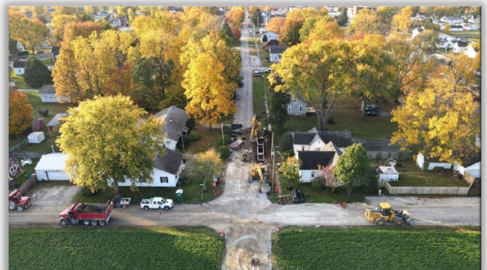
Below: Completed Storm Sewer, Line C
