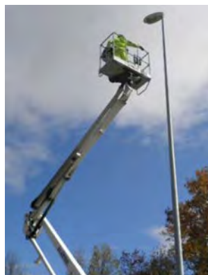
Figure 4.3-22: Lamp replacement
