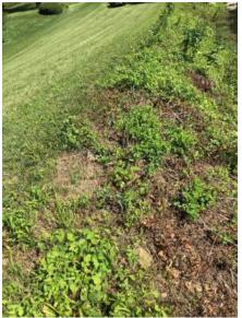
**Photo A25:** View looking north, at upstream embankment east of the spillway where the crest width is only 2 ft wide. Note the downstream sideslope is flat enough to be drivable.
