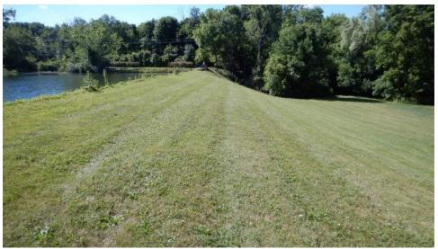
**Photo A23:** View looking South at the downstream embankment east of the spillway. Note the downstream sideslope has a gentle slope.
