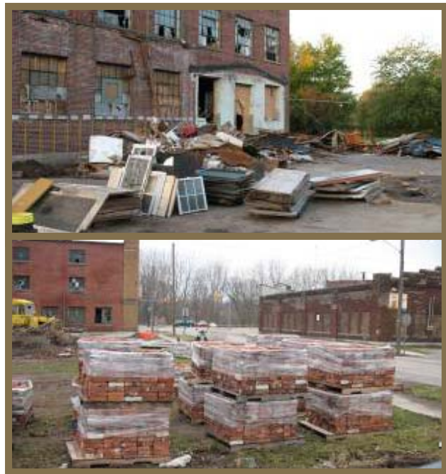
Building materials from the former Essex Wire site in Ligonier in the process of being recycled.
