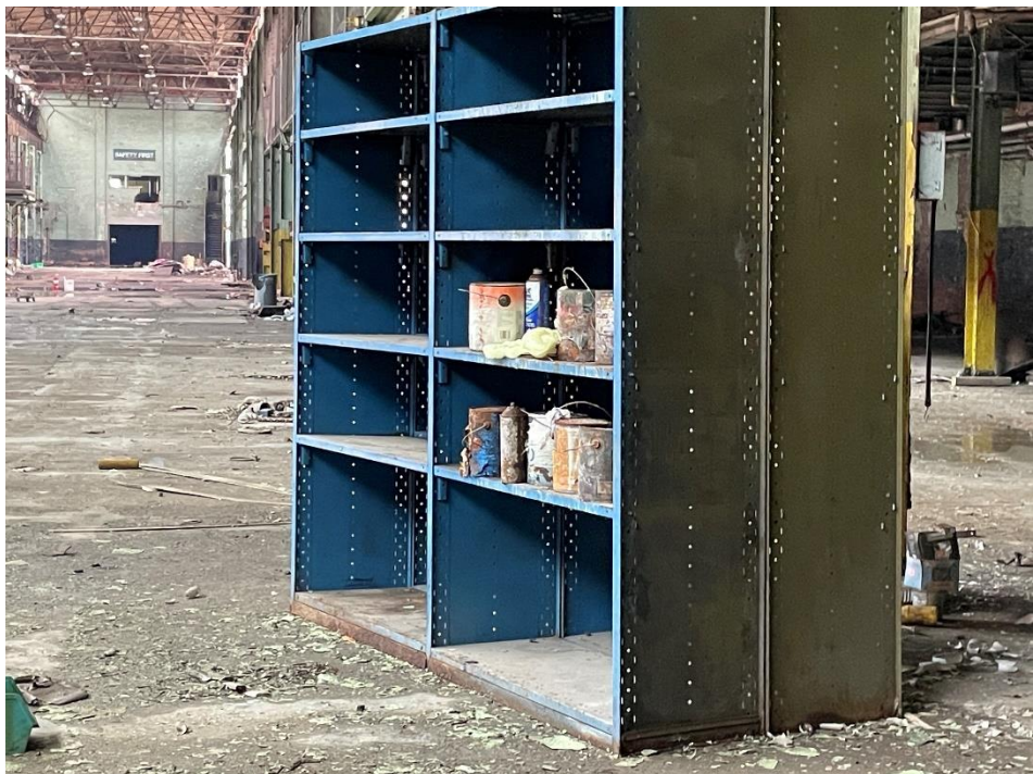
DATE: May 16, 2024 LOCATION: Former Dodge Manufacturing Company / Former RMG Foundry SUBJECT: View of paint in western portion of the complex PHOTOGRAPHER: Robert R. Raduchel (Heartland) PHOTO: 21
