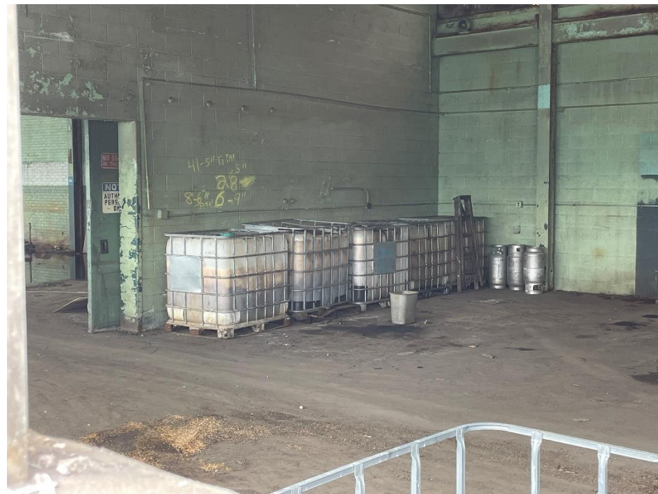
DATE: May 16, 2024 LOCATION: Former Dodge Manufacturing Company / Former RMG Foundry SUBJECT: View of IBC totes and gas cylinders in northern portion of the complex
