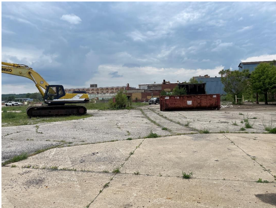
DATE: May 16, 2024 LOCATION: Former Dodge Manufacturing Company / Former RMG Foundry SUBJECT: View of the former rail spur on eastern portion of the subject property PHOTOGRAPHER: Robert R. Raduchel (Heartland) PHOTO: 65
