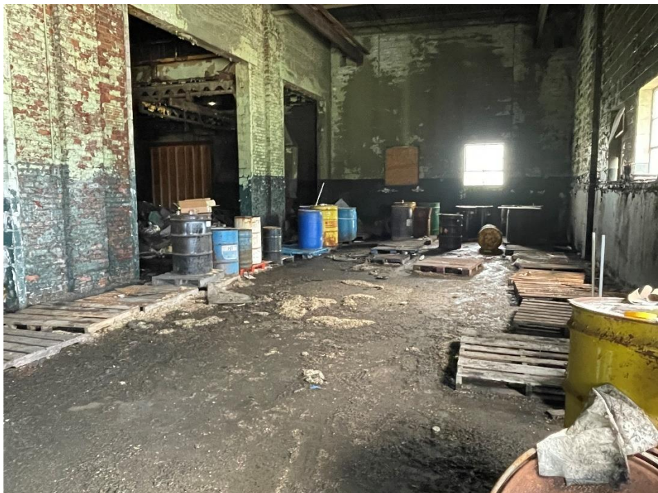
DATE: May 16, 2024 LOCATION: Former Dodge Manufacturing Company / Former RMG Foundry SUBJECT: View of staged chemicals in eastern portion of the complex
