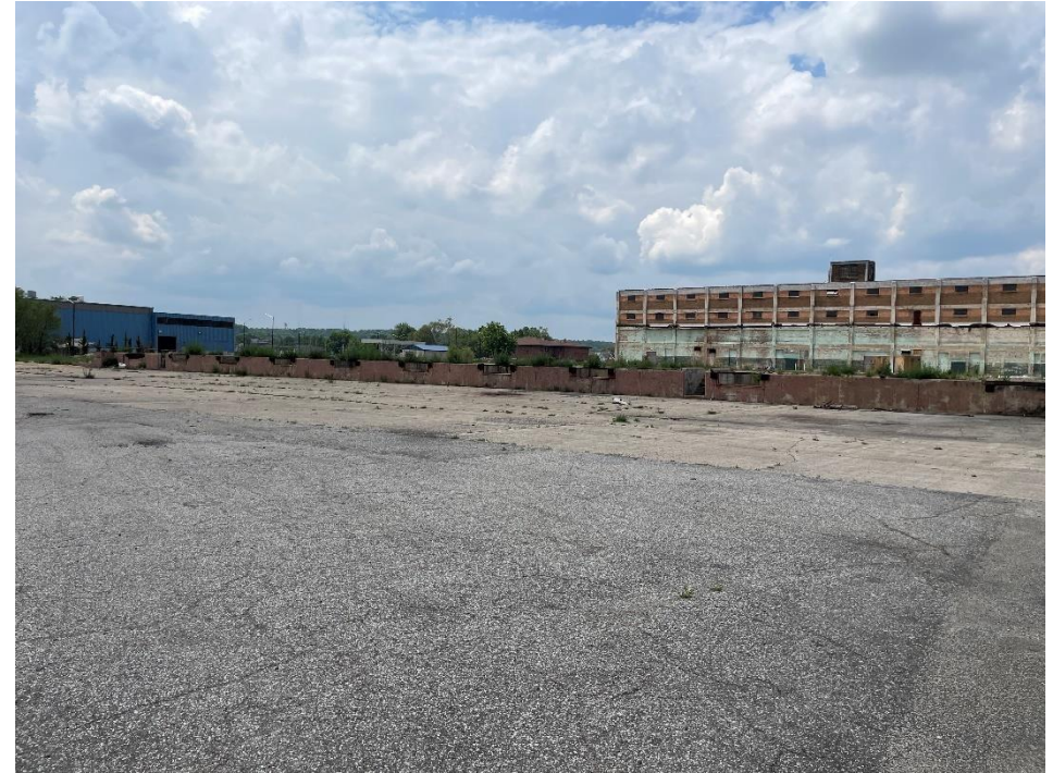
DATE: May 16, 2024 LOCATION: Former Dodge Manufacturing Company / Former RMG Foundry SUBJECT: View of the southern portion of the subject property, looking southwest PHOTOGRAPHER: Robert R. Raduchel (Heartland) PHOTO: 2
