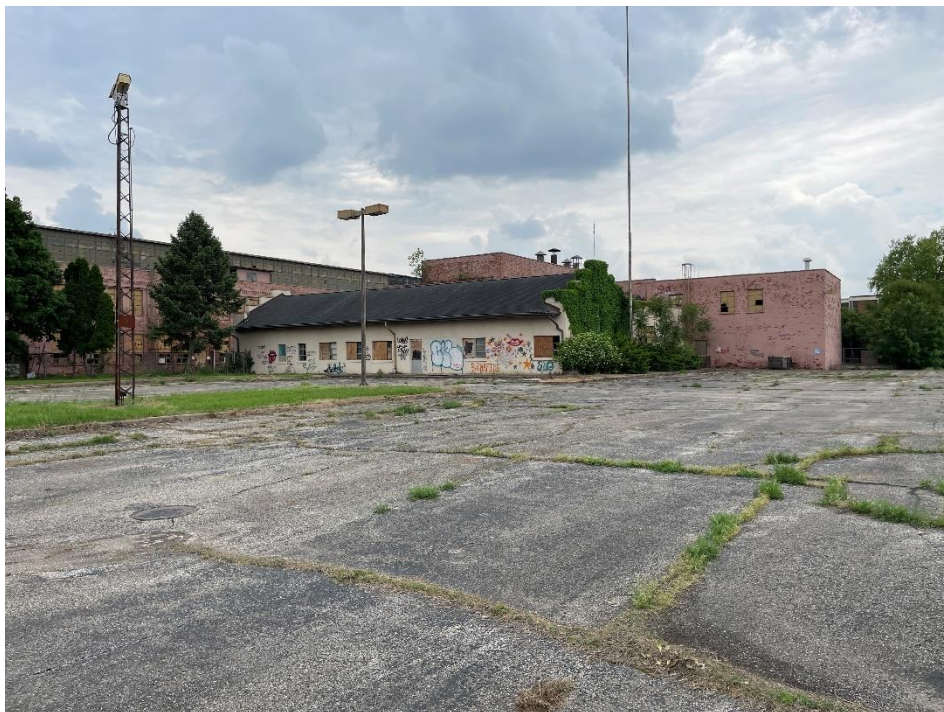
DATE: May 16, 2024 LOCATION: Former Dodge Manufacturing Company / Former RMG Foundry SUBJECT: View of the northern portion of the factory power house, looking southeast PHOTOGRAPHER: Robert R. Raduchel (Heartland) PHOTO: 81
