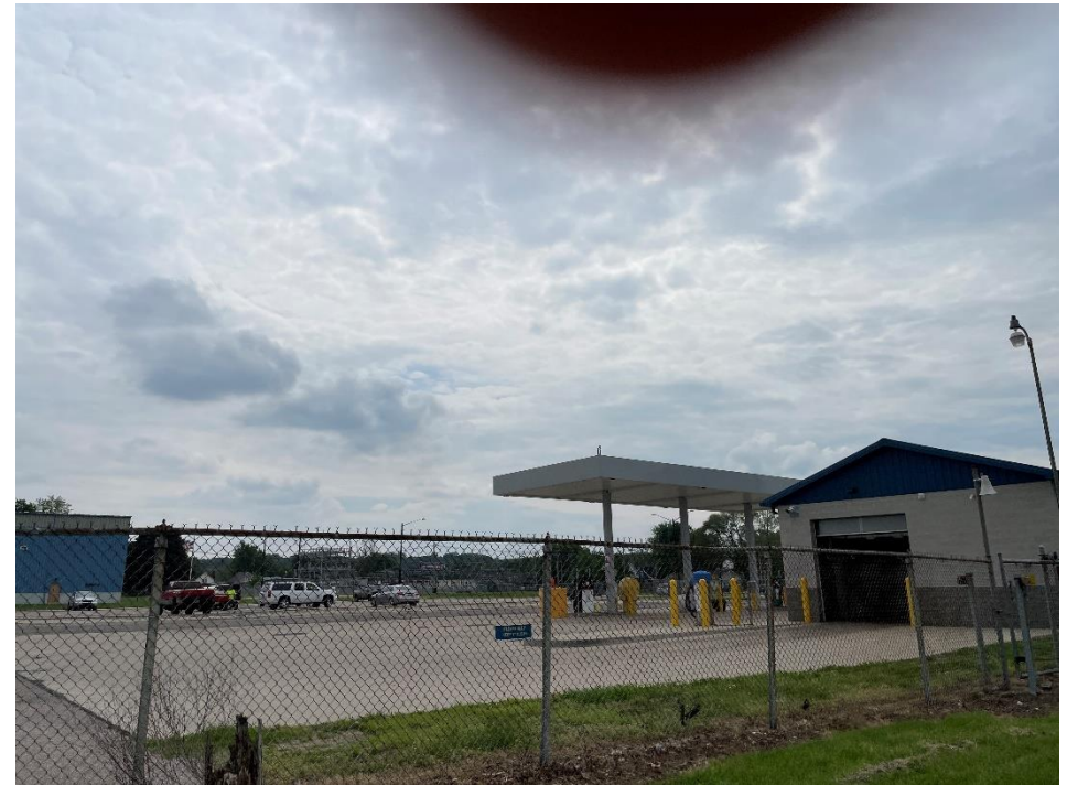
DATE: May 16, 2024 LOCATION: Former Dodge Manufacturing Company / Former RMG Foundry SUBJECT: View of the fueling station adjacent to the south of the subject property
