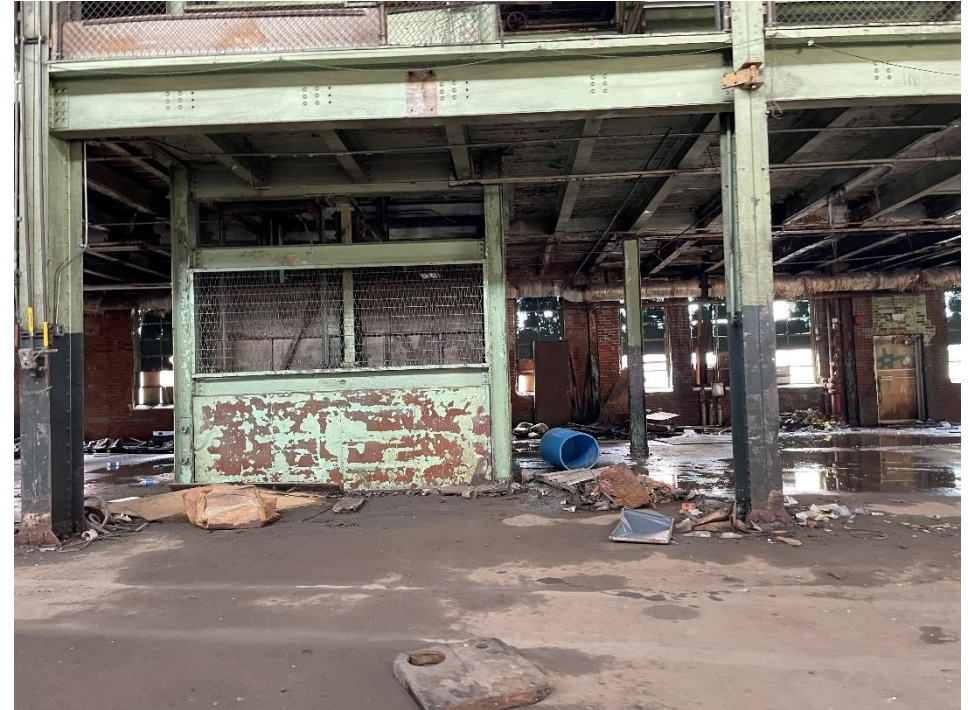
DATE: May 16, 2024 LOCATION: Former Dodge Manufacturing Company / Former RMG Foundry SUBJECT: View of the western freight elevator PHOTOGRAPHER: Robert R. Raduchel (Heartland) PHOTO: 16
