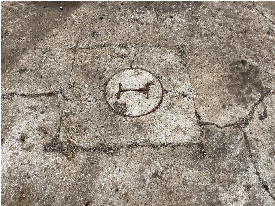
DATE: May 16, 2024 LOCATION: Former Dodge Manufacturing Company / Former RMG Foundry SUBJECT: View of cemented I-beam concrete pad in ground PHOTOGRAPHER: Robert R. Raduchel (Heartland) PHOTO: 13
