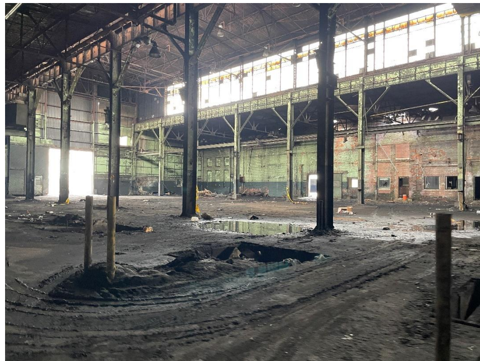
DATE: May 16, 2024 LOCATION: Former Dodge Manufacturing Company / Former RMG Foundry SUBJECT: Additional view of the factory floor area in northern portion of the complex
