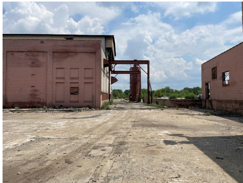
DATE: May 16, 2024 LOCATION: Former Dodge Manufacturing Company / Former RMG Foundry SUBJECT: View of the foundry sand silo (AST), looking east PHOTOGRAPHER: Robert R. Raduchel (Heartland) PHOTO: 8
