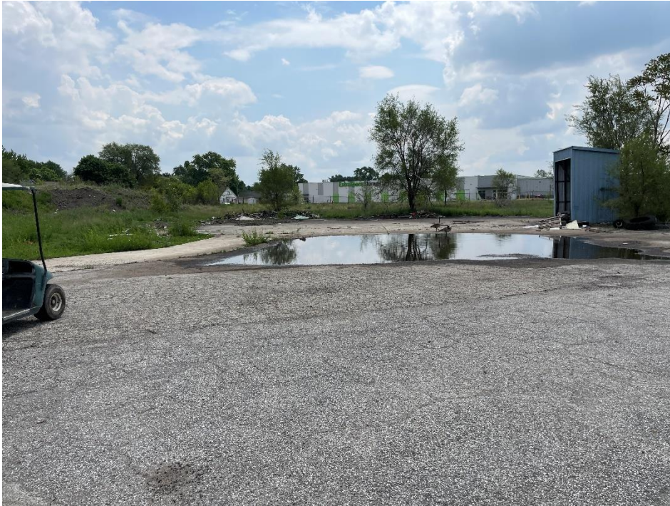
DATE: May 16, 2024 LOCATION: Former Dodge Manufacturing Company / Former RMG Foundry SUBJECT: View of the southeastern portion of the subject property, looking southeast PHOTOGRAPHER: Robert R. Raduchel (Heartland) PHOTO: 1
