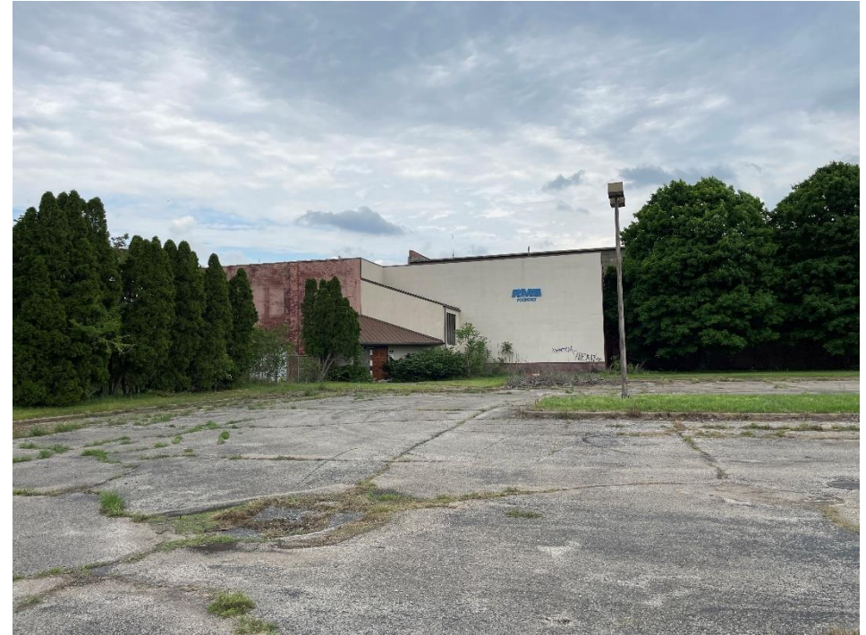
DATE: May 16, 2024 LOCATION: Former Dodge Manufacturing Company / Former RMG Foundry SUBJECT: View of the factory entrance, looking east PHOTOGRAPHER: Robert R. Raduchel (Heartland) PHOTO: 80
