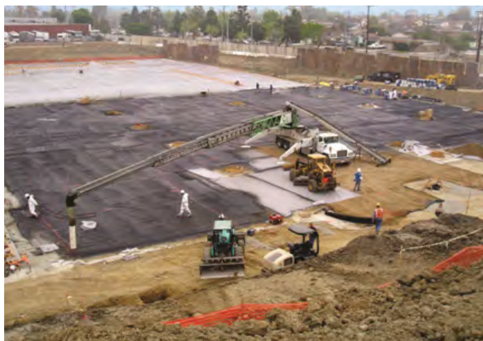
Figure 12. Installation of a spray-applied barrier at a large site.
