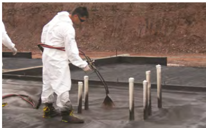
Figure 11. Spraying an emulsified asphalt latex barrier.
