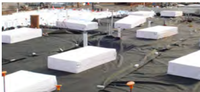
Figure 8. Standard vapor barrier with unsealed seams.
