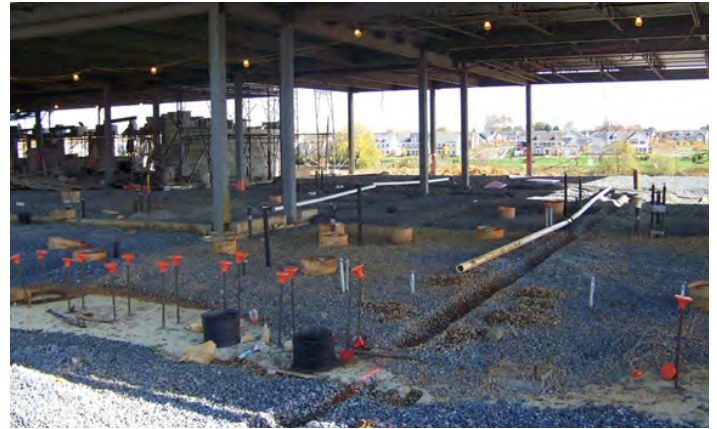
Figure 3. Gravel placed over proof-rolled site with trenching for vent piping.
