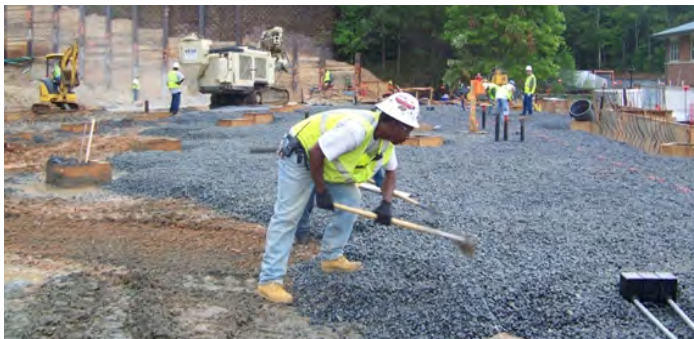
Figure 2. Proof-rolled ground covered with 8 inches AASHTO #57 stone.
