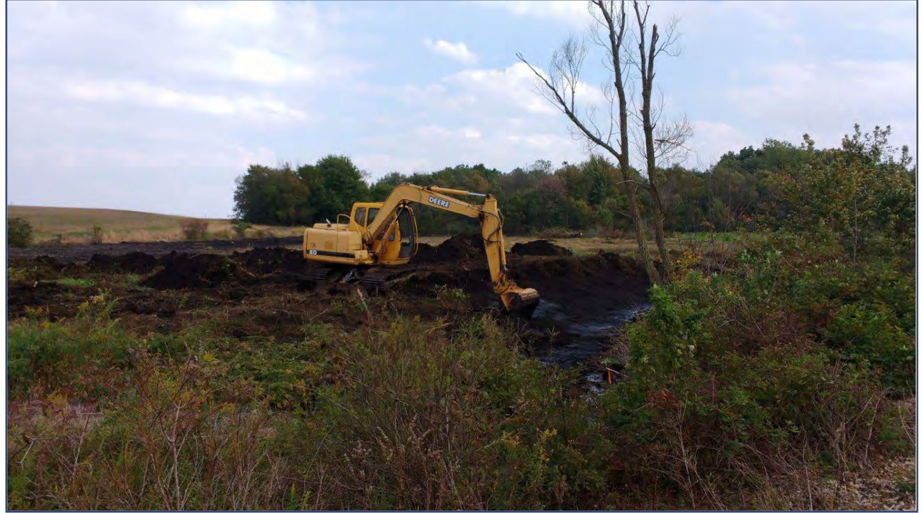
Stream meander creation using a tracked excavator. The steep-sided ditch banks were pulled back and the channel bottom was reconfigured with pools and riffles to create a natural stream course.
