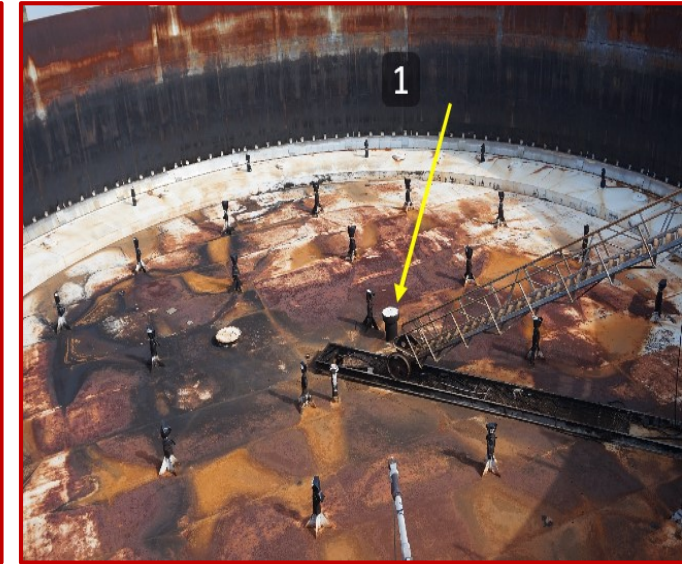
(Above) Leaking vent at a floating roof tank facility. Courtesy: Infrared Cameras Inc.
