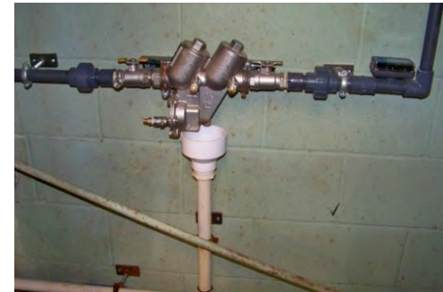
Backflow Preventer & water meter
