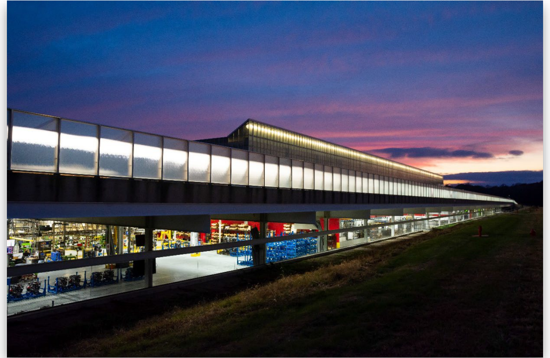
Columbus Midrange Engine Plant
