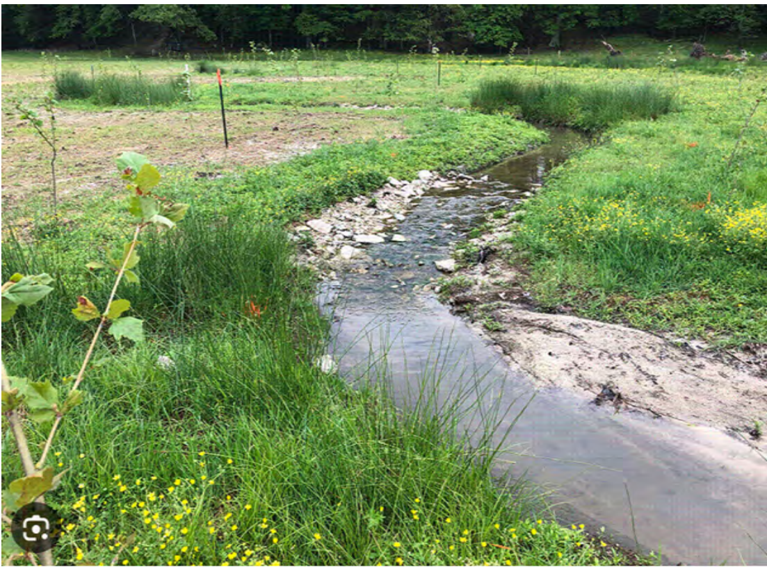
CONSTRUCTED RIFFLE EXAMPLE PHOTO
