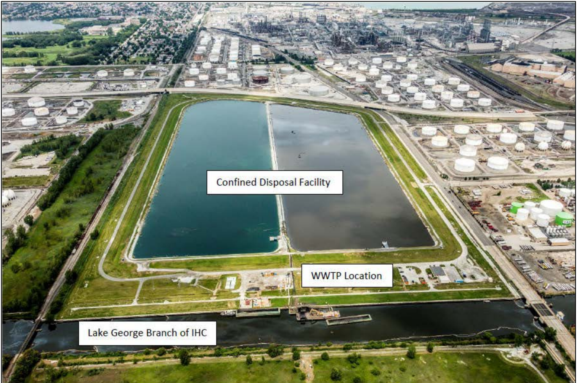
Figure 4 – Confined Disposal Facility and Package Wastewater Treatment Plant
