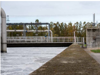
SEA 459 mandates cybersecurity measures for certain water and wastewater facilities.
