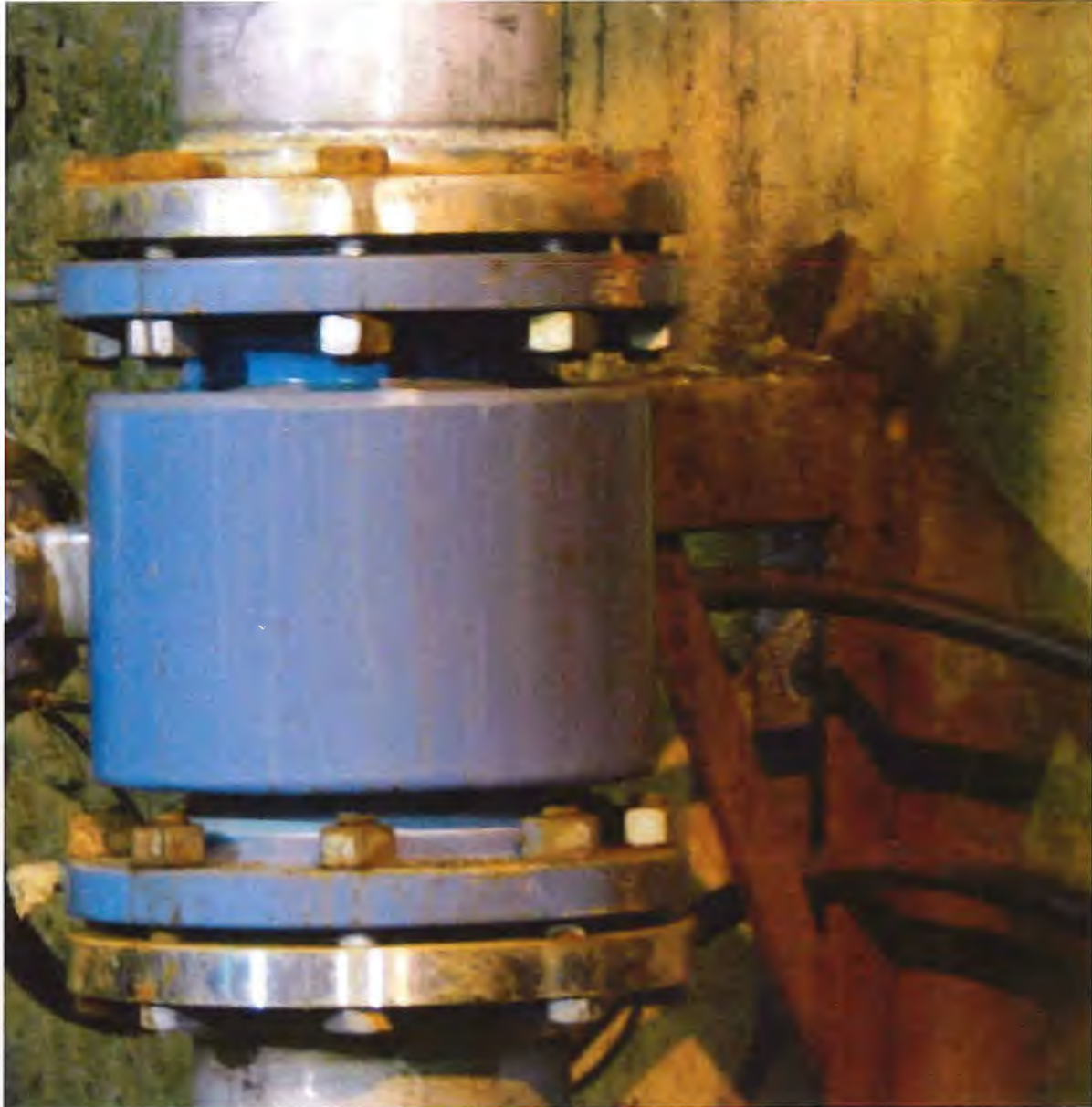
Picture 6: Chrome containment trench: pictures of inlet flow meter on chrome transfer pipeline
