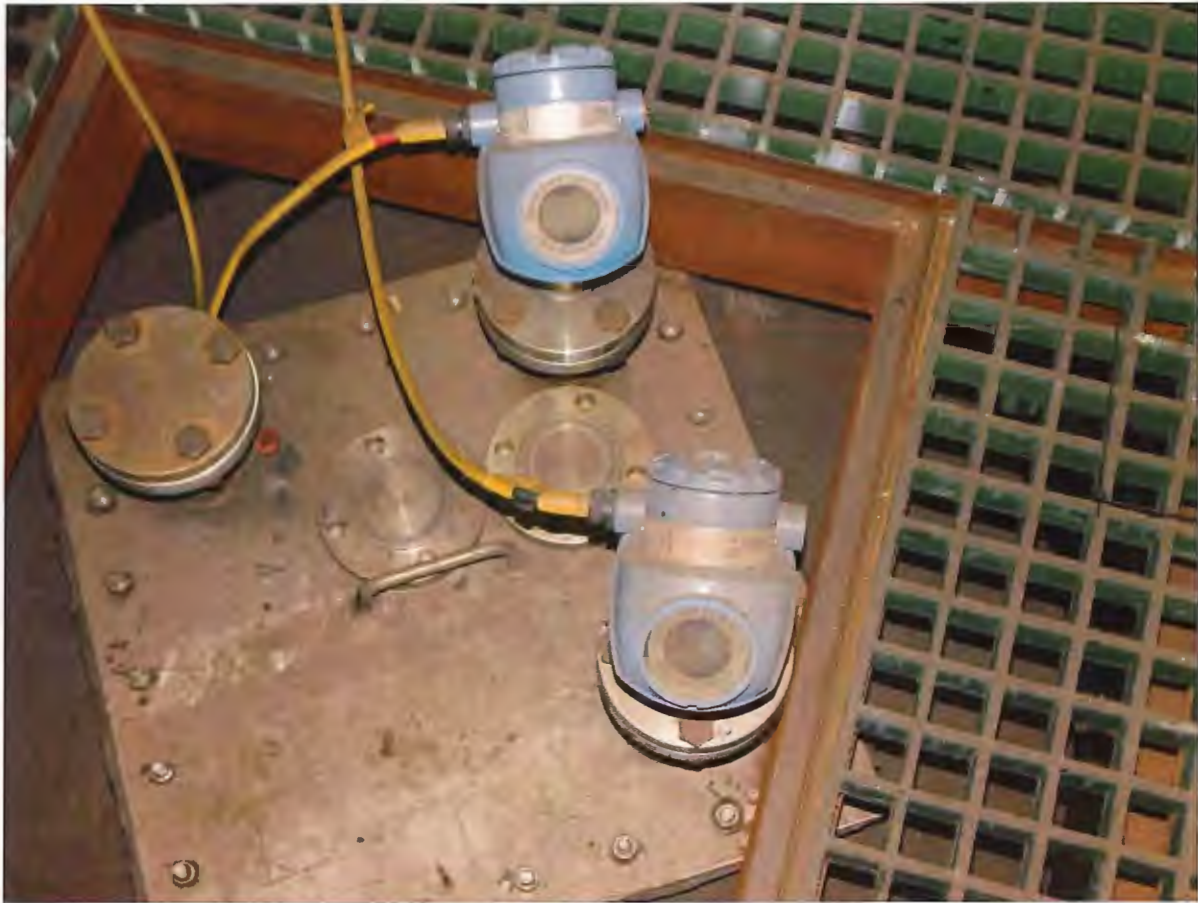
Picture 11: Chrome Line Evaporator: Picture of redundant level sensors installed on top of Evaporator
